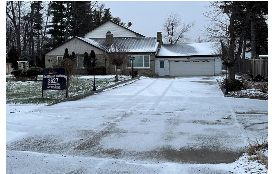
View of site. Existing structure, to remain
