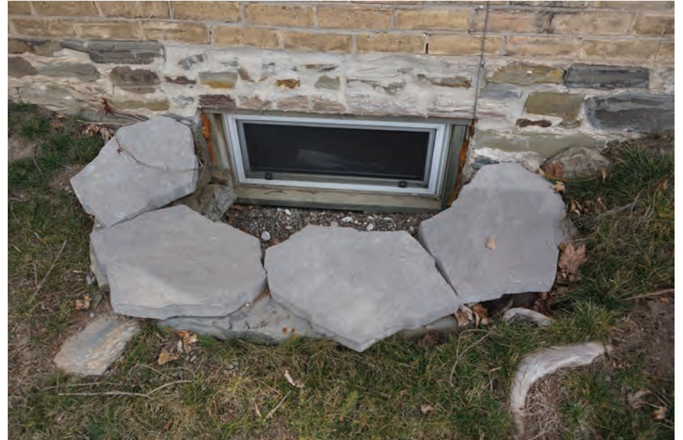
Pressure treated wood framing / drystone light well.
