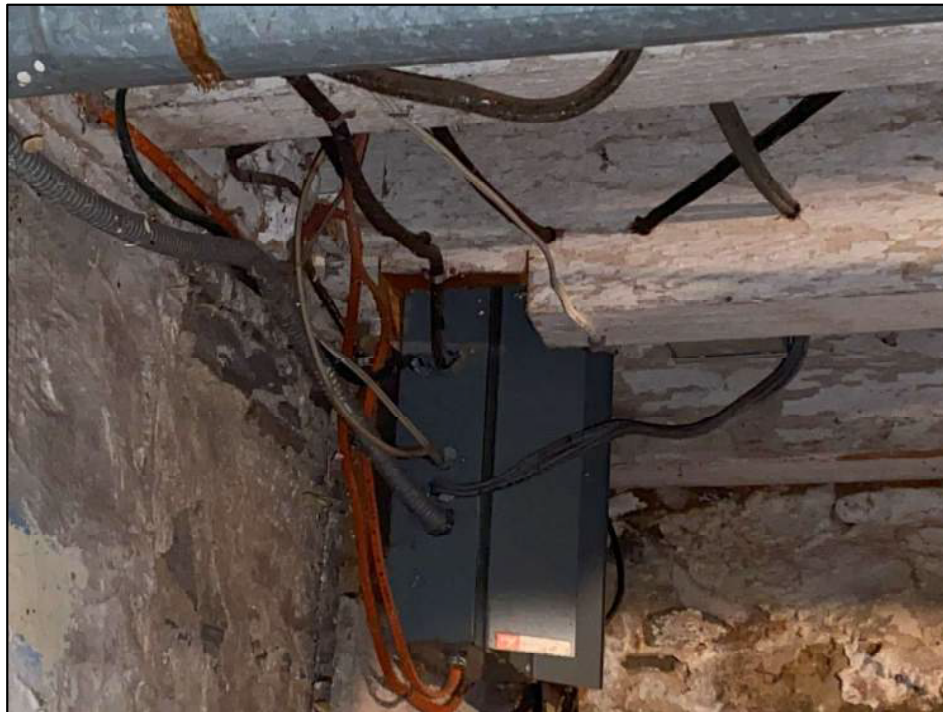
Photograph 3: Notched joist behind furnace
