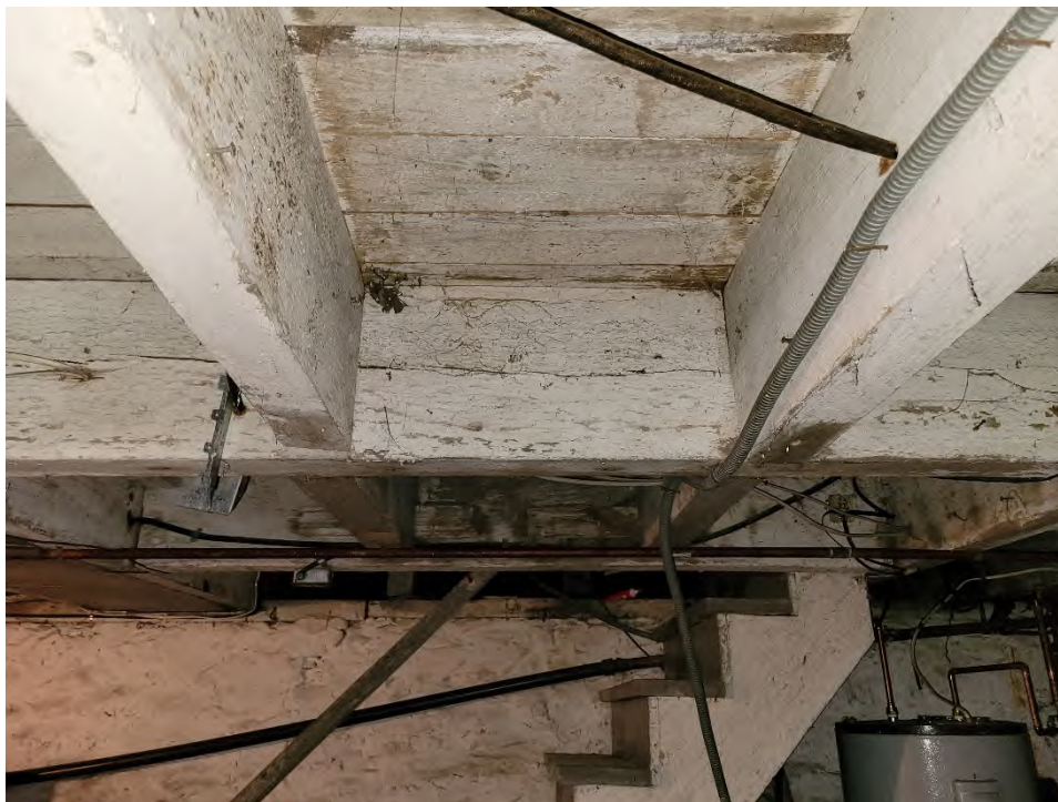
Figure 56: Exposed floor joists left in the rough in the south half of the main block
