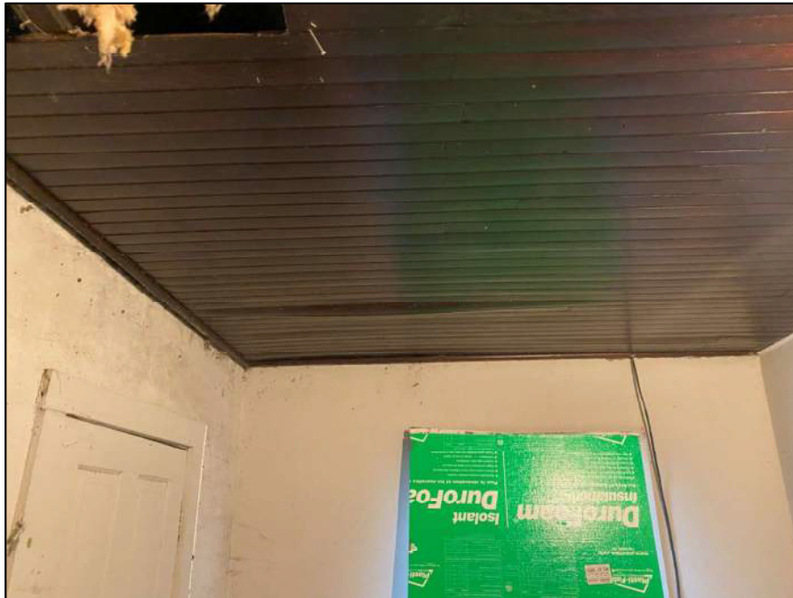
Photograph 5: Water damage to ceiling finishes
