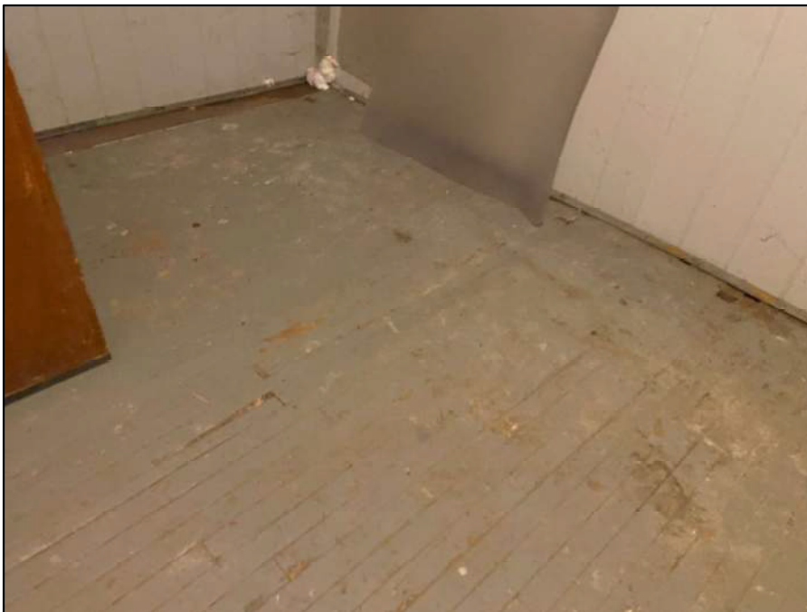
Photograph 6: Water damage to floor finishes
