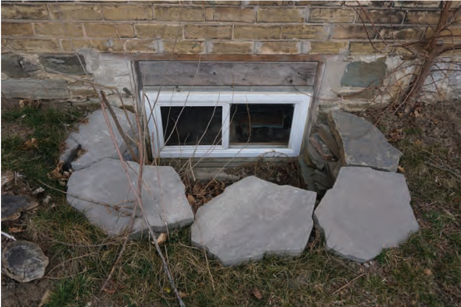
New basement window and wood lintel.
