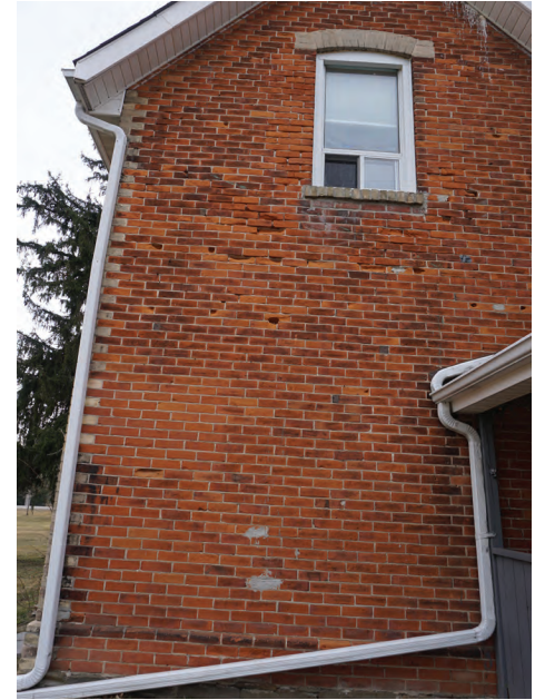
Brick damage along window
