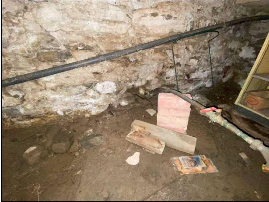
Photograph 4: Undermined section of foundation wall
