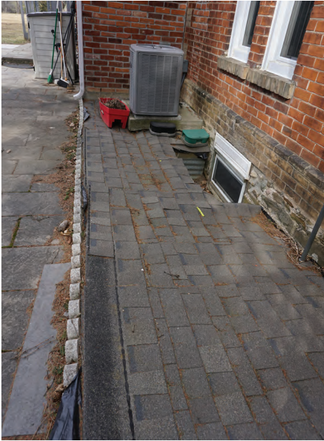
Asphalt single apron and precast curb.
