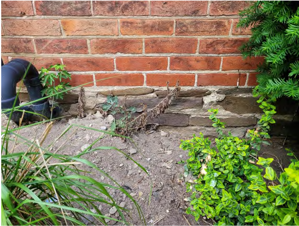
Figure 20: Coursed split fieldstone foundation
