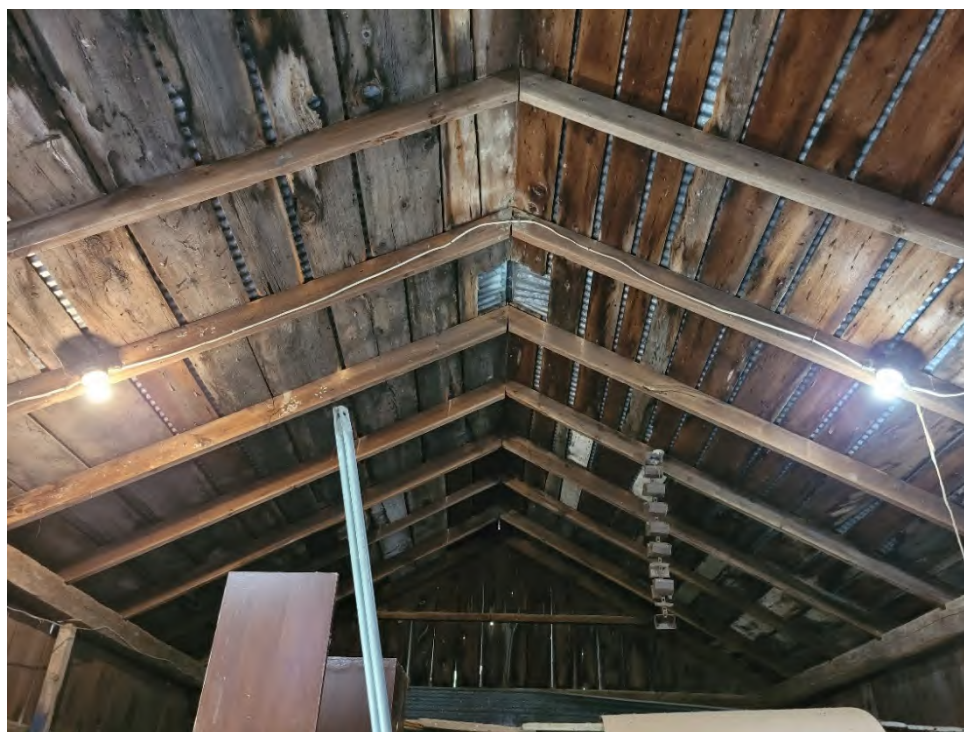
Figure 68: Dimensional cut rafters
