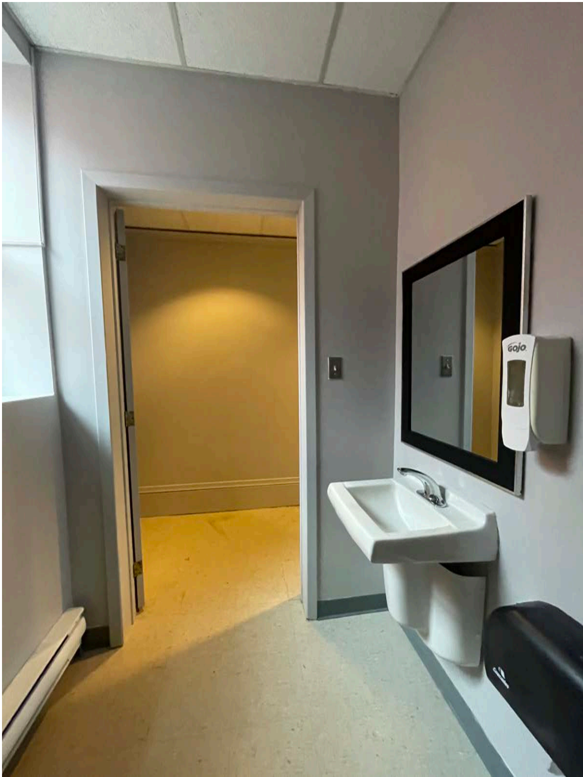
WASHROOM – existing two-piece washroom on the lower level – nor original features or finishes - modern fixtures, drywall, vinyl flooring & acoustic tile ceiling – door casing on interior side is not original
