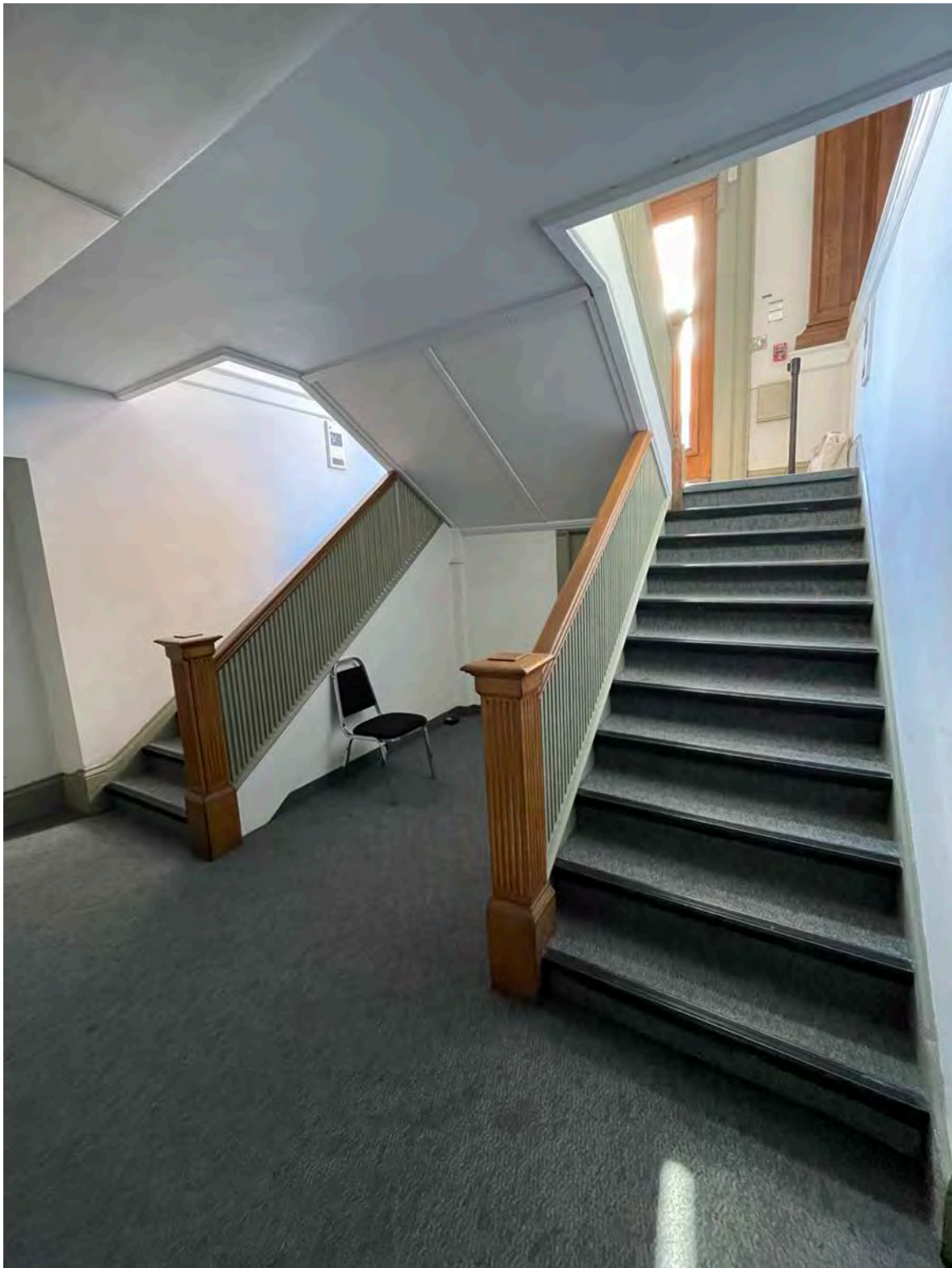
INTERIOR – LOWER LEVEL: view looking up to the entrance vestibule from the lower level – two sets of stairs down to the lower level and one set of stairs to the main floor – original features and finishes include the oak newel posts and railings – plaster & lathe walls and wood baseboards – wall to wall carpet has been installed on the original stair treads and risers
