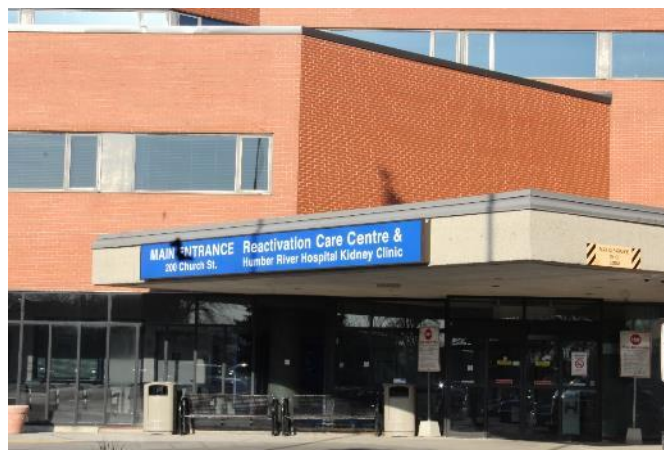
Reactivation Care Unit
