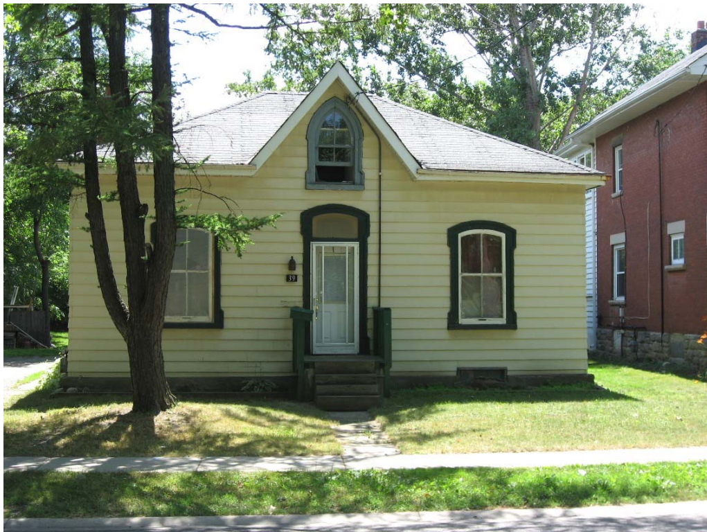
Figure 7: Front facade of 39 Mill Street North with three bays, hipped roof with cross gable sheltering a Gothic window, and wooden sash 2-over-2 windows with storms
