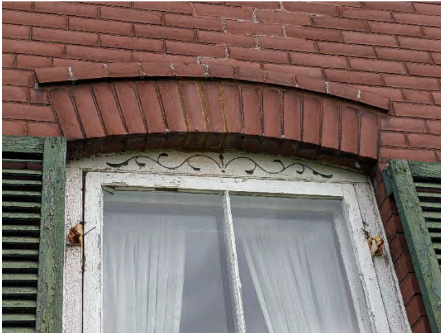
Image 23: Detail of perforated design on some of the segmentally arched windows.
