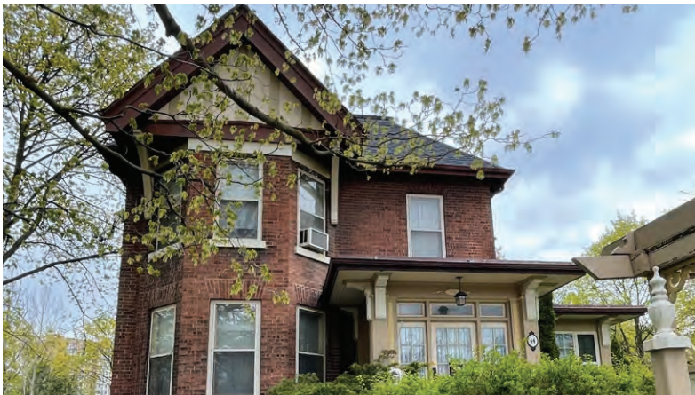
The building at 44 Mill Street North (designated) is clad in red-brick masonry laid in a stretcher bond (ERA, 2024).
