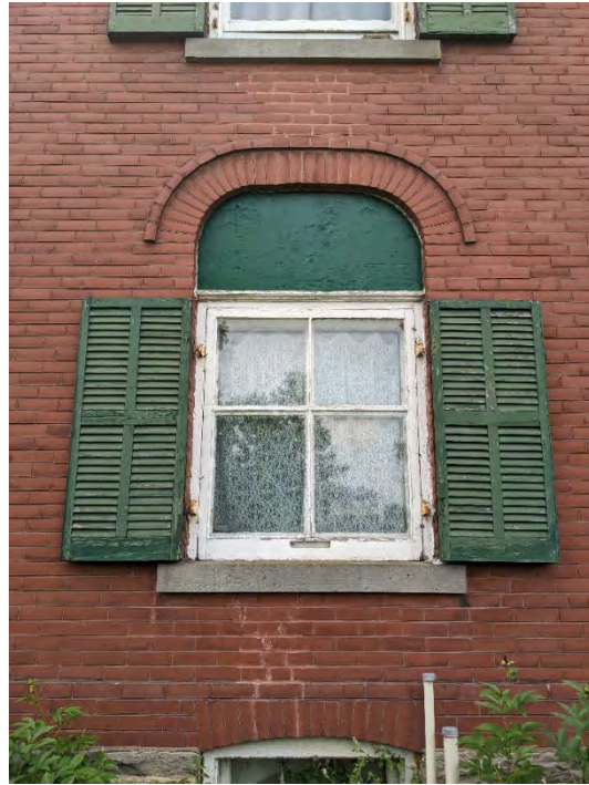
Image 22: View of a rectangular window with a flat arched transom.
