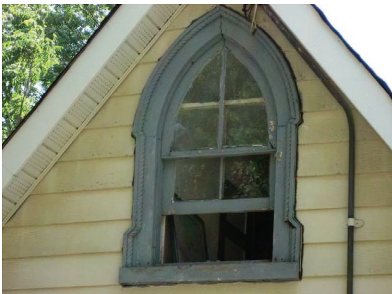
Undated photograph showing a close-up of the lancet arch window above the door at the east elevation of 39 Mill Street North, featuring a window surround with decorative spindling (City of Brampton).
