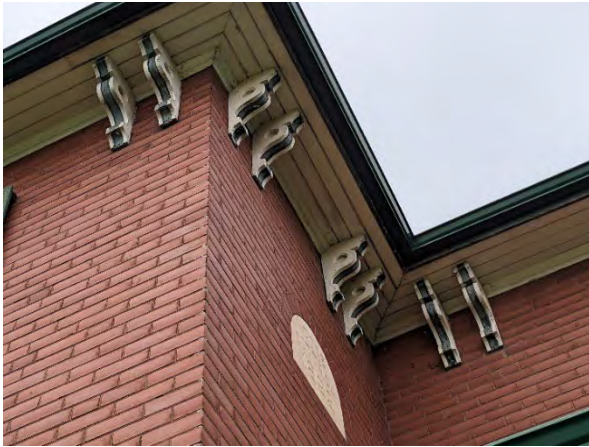
Image 25: Detail of paired brackets under the eaves.
