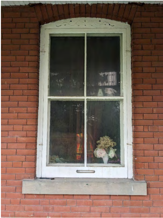
Image 21: View of a segmentally arched window on the farmhouse's front facade.
