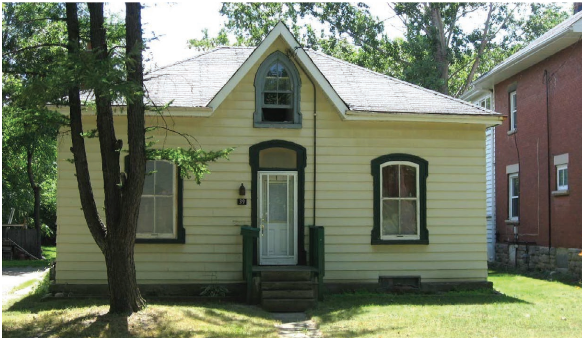
Undated photograph showing the principal (east) elevation of 39 Mill Street. The window and door surrounds have since been overclad or removed, and two-over-two wooden windows and storms removed (City of Brampton).
