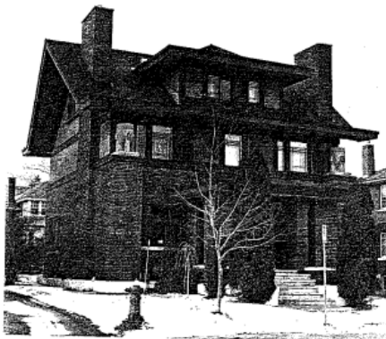
20-1 Noteworthy features of this Prairie-style house in Ottawa include: - continuous stone sill - string courses of dark-stained wood bands - a shortened second-storey level - horizontal or all-stretcher brick bond - square roof cornice - unsupported eaves - geometric window glazing
