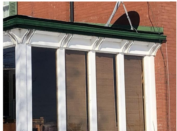
Plate 26: Detail of sunroom showing wooden brackets.
