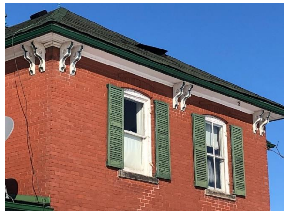
Plate 20: Typical windows and paired wooden brackets.
