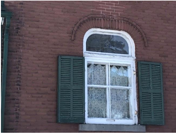
Plate 21: First-storey window with leaded-glass transom and projecting brick arch on east elevation.
