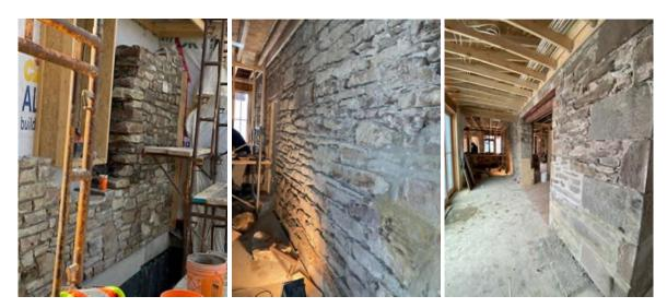
Figure 19: Process to create the masonry veneer. Left: framing complete before laying up veneer. Centre: Veneer laid up in mortar. Right: Grout applied for a uniform finish (subsequently acid treated) (from Robert Wilson House, Town of Caledon, courtesy Sedgwick Marshall Heritage Homes Ltd)
