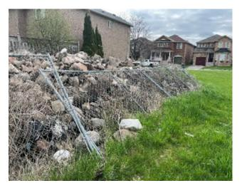
Figure 6: Partially collapsed southwest fencing
