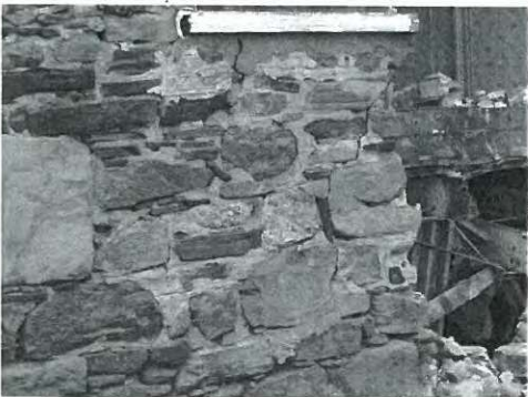
Crack propagation south side.
