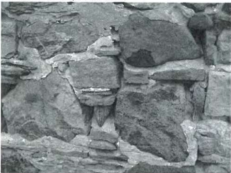
Mortar erosion, west side.
