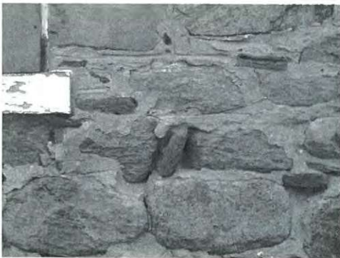
Mortar erosion, west side.
