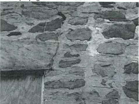
Crack propagation south side.
