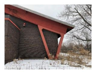
Image 8: View of the concrete pillar supporting the glulam beam, note all concrete pillars are of this shape, but the other concrete pillars are partially enclosed inside the building.
