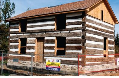
made the City a gift of the log house. Although erected circa 1850, the bricks that clad the building since the early 1920s actually protected and conserved the logs, most of which were determined as being elm. With virtually all of the logs in an excellent, well-preserved condition, the relocated house has become a perfect addition to the Historic Bovaird House site.
