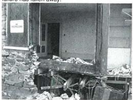
South side. Visible evidence of rot at joist ends.
