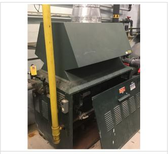
Figure D03.1 – Existing Atmospheric Pool Boiler
