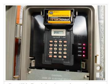
Figure A03.3 – Timerclock used to control some washroom lighting, set to operated 24/7.
