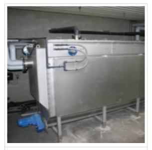
Figure D11.2- Waste Water Source Heat Pump
