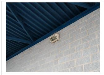
Figure A02.1 – Existing metal halide wall packs
