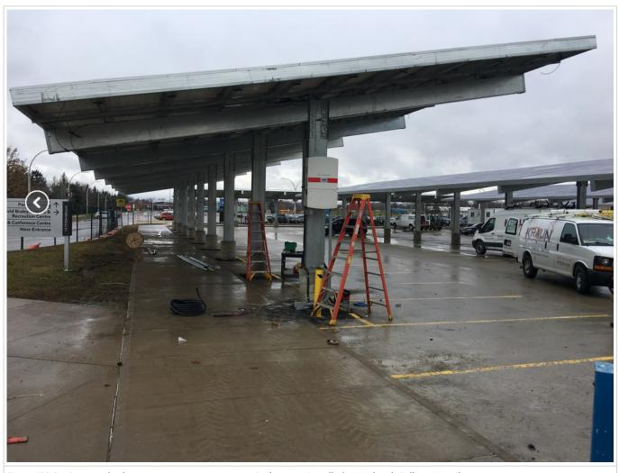
Figure IO2.2: : Proposed solar carport support structure, similar array installed at Mohawk College, Hamilton
