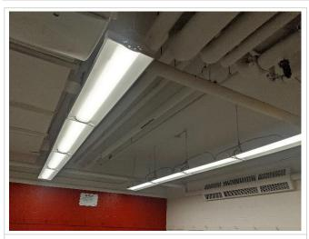
Figure A03.1 – Typical lighting layout in a change room. Occupancy sensor to be place in center of room.
