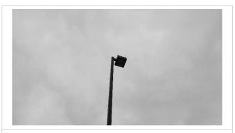
Figure A02.3 – Typical metal halide pole lighting illuminating the parking area
