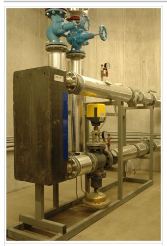
Figure D12.1- Example of District Heating Substation
