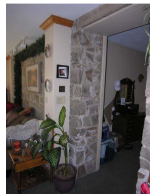
Figure 20: Farmhouse Interior, detail view of former east facade, showing the wall thickness, the rough rubble fieldstone and the doorway converted from the original window for the 1991 addition.
