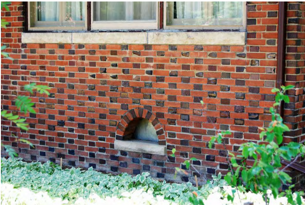
Figure 6: Detail showing the scupper below what might once have been an open porch at the corner of the house near the intersection of Isabella Street and Lorne Avenue. The photo also shows the stone sills found under most structural openings.
