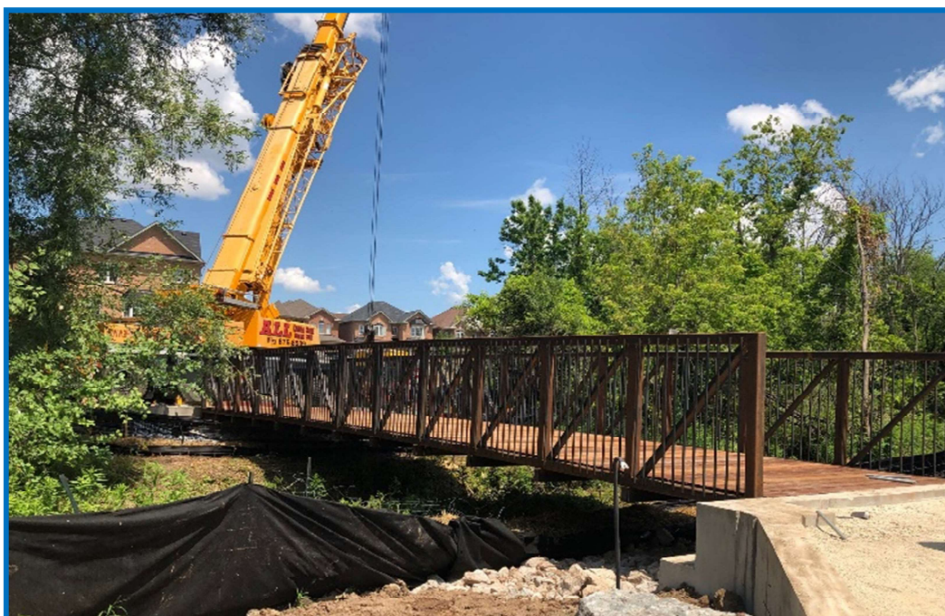
FP BLOCK 5 PHASE 2 PEDESTRIAN BRIDGE INSTALLATION
