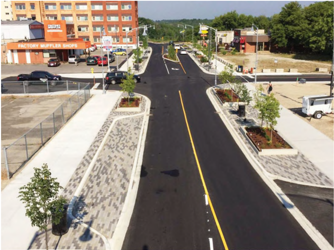
Figure 11: A new street constructed with a number of traffic calming features to improve safety (Credit: WSP)
