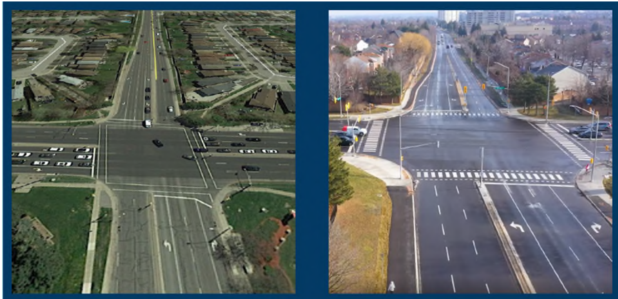
Figure 10: Clarke Avenue in Vaughan reconstructed as a Complete Street, with fully-accessible pedestrian and bicycle crossings, multi-use pathways, cycle tracks, and a transit “queue jump” lane (Credit: WSP)
