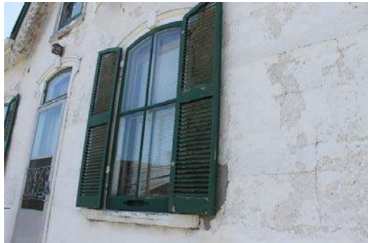
Figure 30 - Deterioration on Exterior Wall & Arched Windows with Cracks
