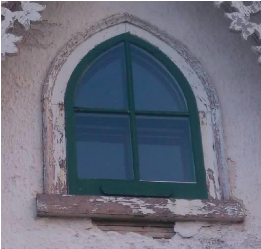
Figure 6: East façade lancet window with wood surround and sill. Wood lathe visible underneath (2017).
