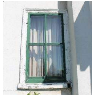
Figure 29 - Peeling Paint on Window Frame
