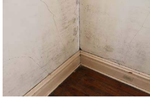
Figure 20 - Hairline Cracks on Interior Walls
