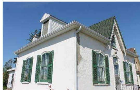
Figure 33 - Paint peeled of Pebble-Stucco Wall
