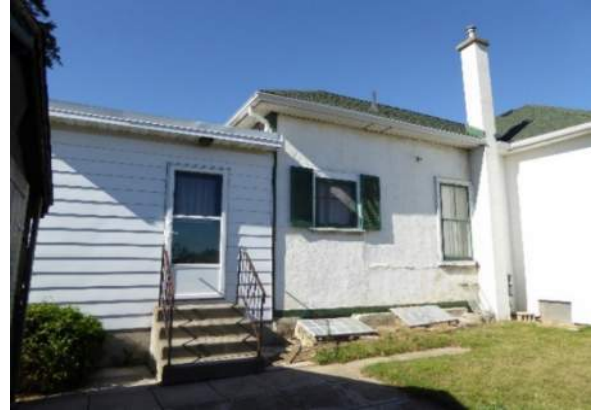
Figure 41 - South Elevation showing "Ell" Addition with metal siding & concrete block chimney
