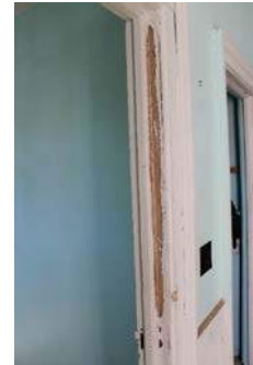
Figure 24 - Cracks & Peeling on Wood Door Frame
