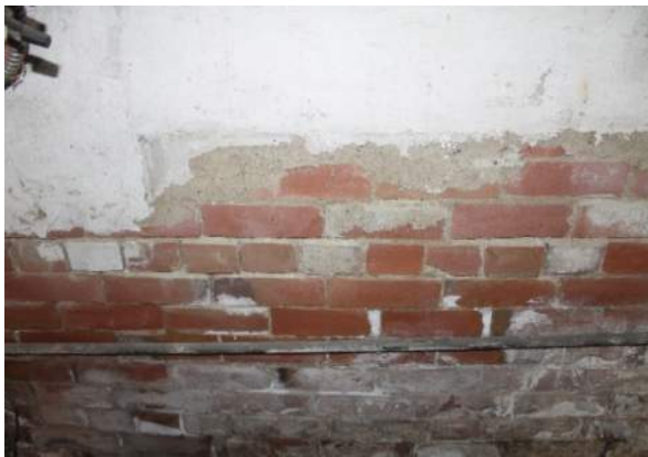
Figure 44 - Partially Painted Brick Foundation Wall facing west
