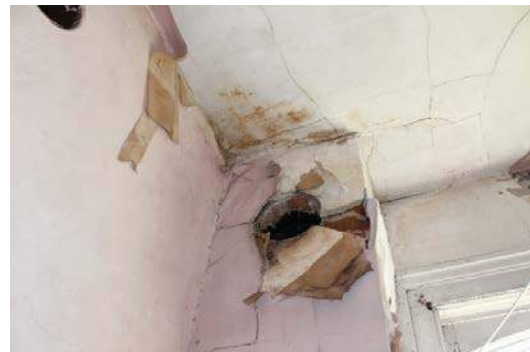
Figure 18 - Visible Hole in Wall Assembly from former (stove) pipe
