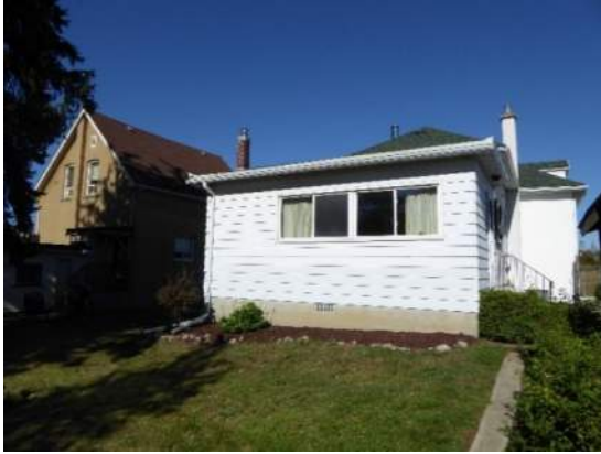
Figure 40 - West Elevation showing enclosed porch clad in metal siding
