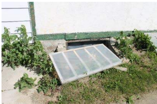
Figure 32 - Detached Window Cover for Basement Window
