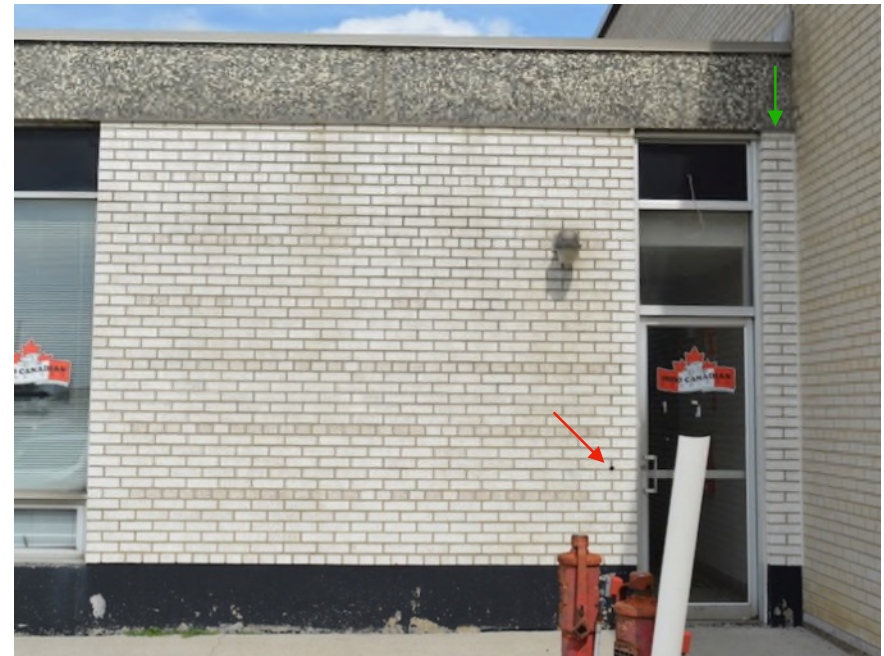
Example of brick panel on the south elevation, adjacent to the existing warehouse building. Dirt from water damage is noticeable at the top and will be cleaned. The lighting fixture will be removed. The hole (red arrow) will be patched. The residual brick pilaster (green arrow) will be removed and rebuilt as it can not be salvaged in one piece and removal of bricks, laid in a cement-based mortar, will damage the edges of the brick.
