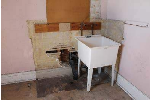
Figure 19 - Exposed Wood Framing & Deteriorated Wall Finishes
