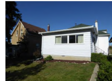
WEST ELEVATION SHOWING ENCLOSED PORCH CLAD IN METAL SIDING (VIEW 8)
