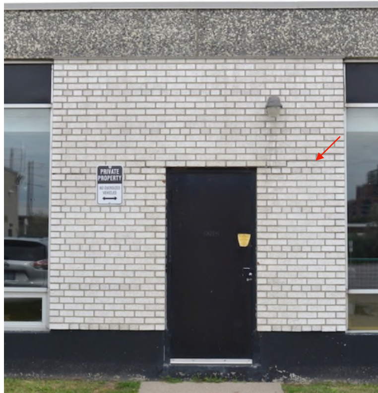
Example of brick panel on the north elevation. Note the stepped cracking (red arrow) which shows that some movement has occurred in the veneer. The untypical opening in this panel will be challenging to safely dismantle and salvage without placing additional stress and strain to the assembly. This panel is proposed to be dismantled and rebuilt with bricks to match.
