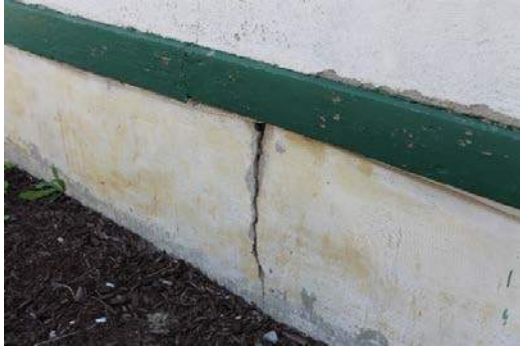
Figure 26 - Cracks in Exterior Wall
