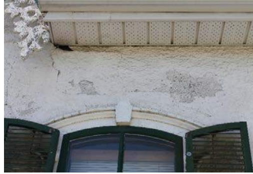
Figure 27- Hairline Cracks & Chipped Paint on Exterior Wall
