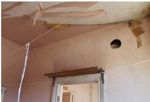
Figure 17 - Peeling Paint Finishes on Ceiling
