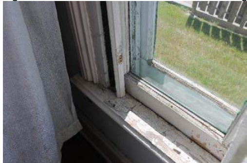
Figure 23 - Chipped & Decayed Window Sills & Frames
