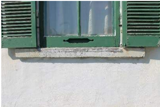
Figure 28 - Peeling Paint on Window Sill & Exterior Shutters
