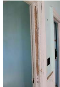
Figure 24 - Cracks & Peeling on Wood Door Frame
