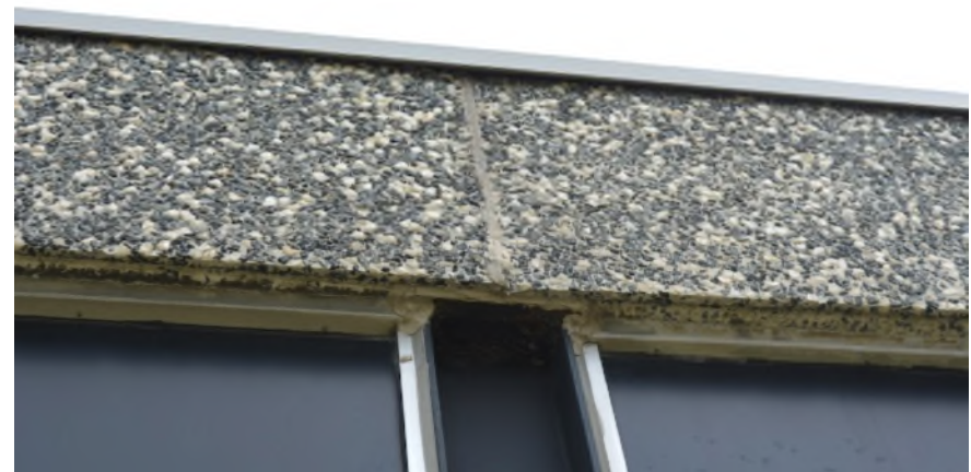
Example of aggregate panels at the main (west) elevation. Underside of the panel shows a thin assembly.
