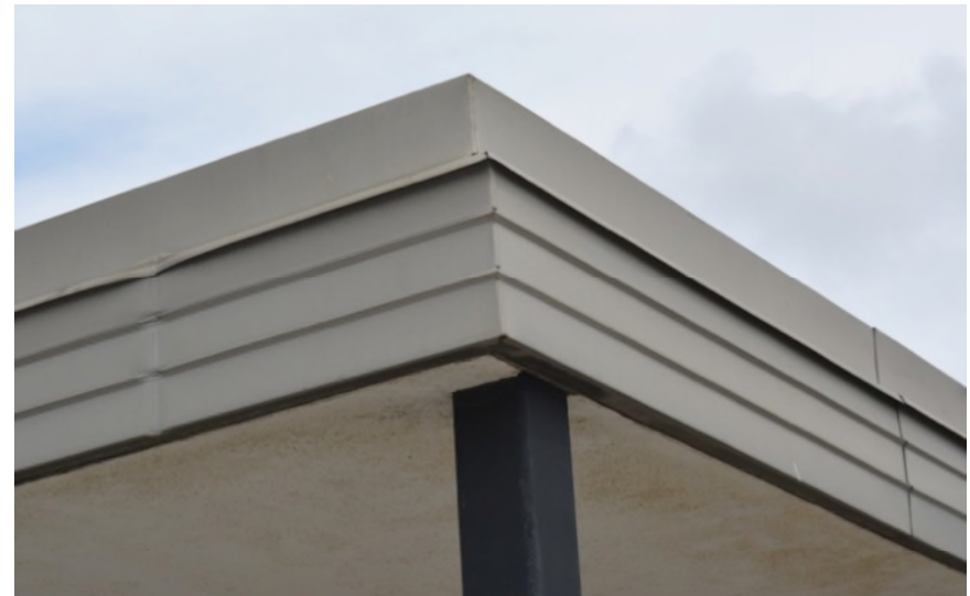
Close-up of canopy metal siding, with horizontal seams
