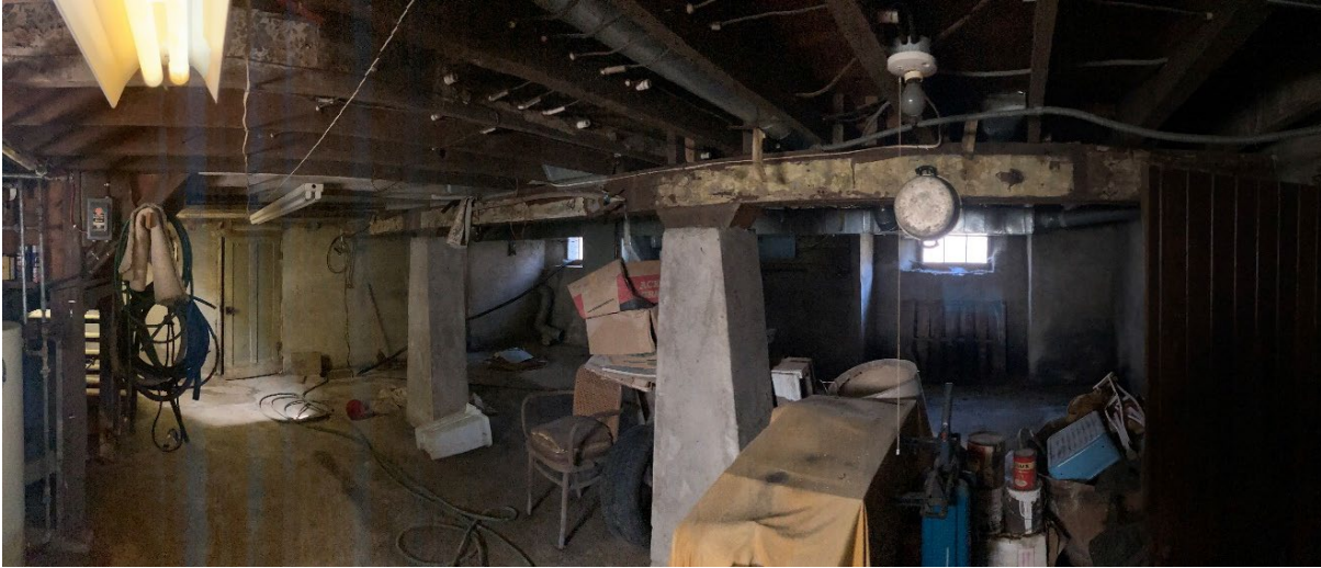
Plate 22: Basement main area showing the machine cut summer beam and concrete pilasters
