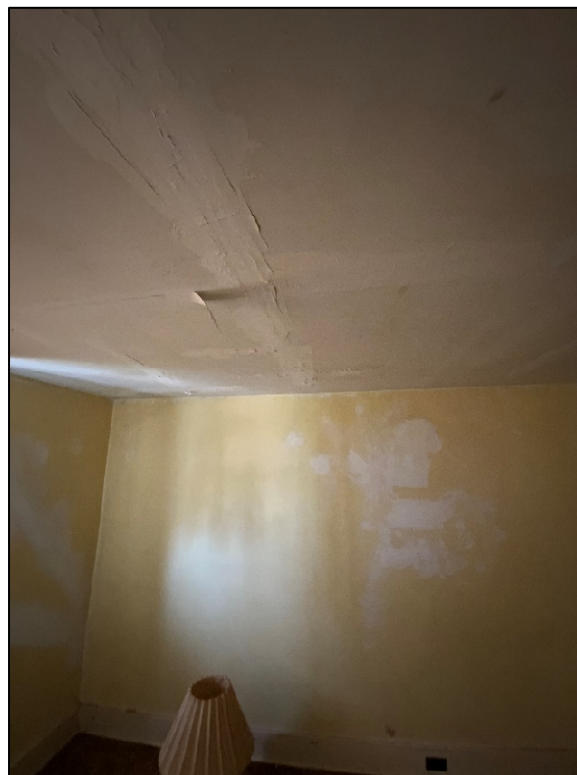
Photograph 2: Previously repaired ceiling damage
