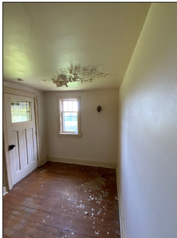
Photograph 1: Minor ceiling damage
