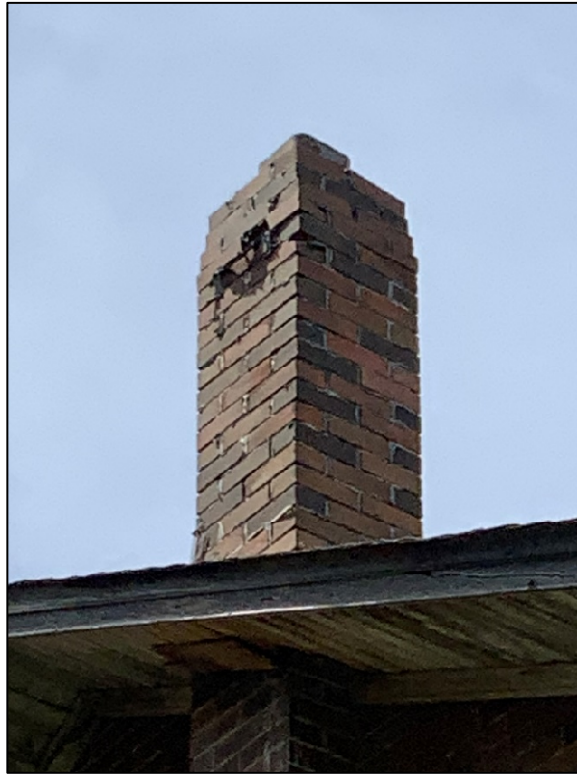
Photograph 4: Damaged masonry at southeast chimney (typical to both chimneys)
