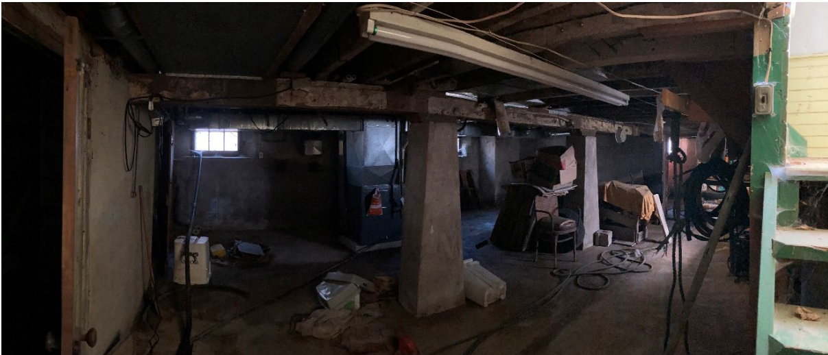
Plate 21: Basement main area including summer beams and concrete pilasters
