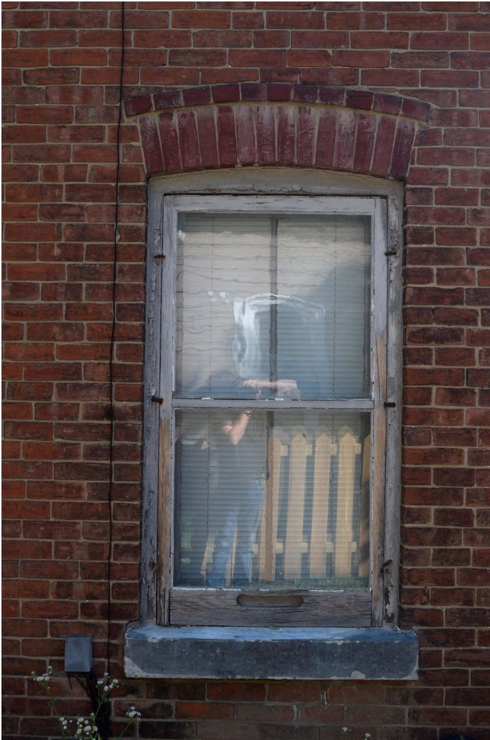
Figure 16: Typical original two over two sash window with replacement cast lug sill (original sills were wood)
