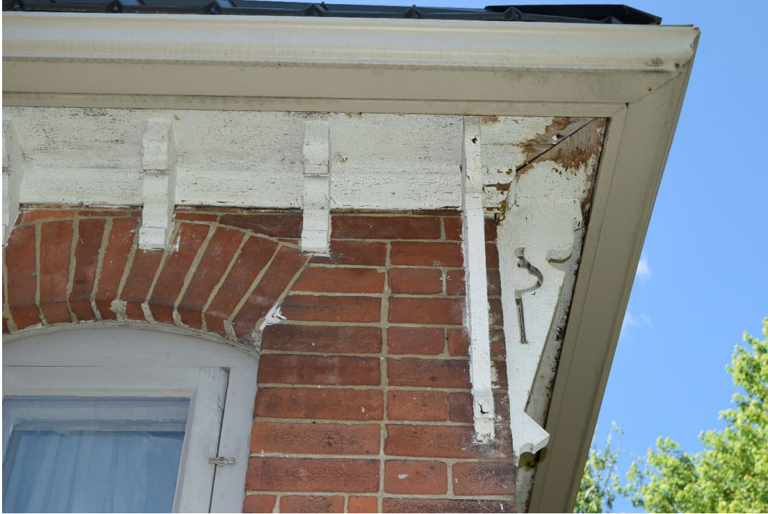
Figure 19: Original brackets on bay window
