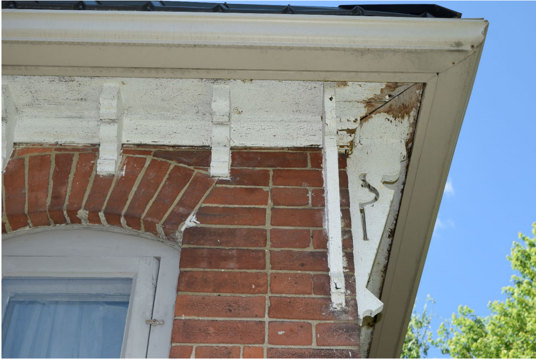
Figure 19: Original brackets on bay window
