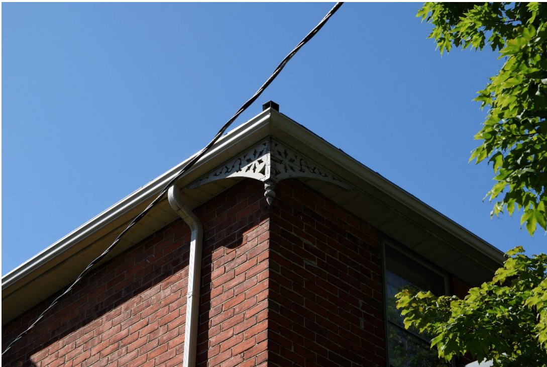
Figure 18: Example of remaining millwork at eaves
