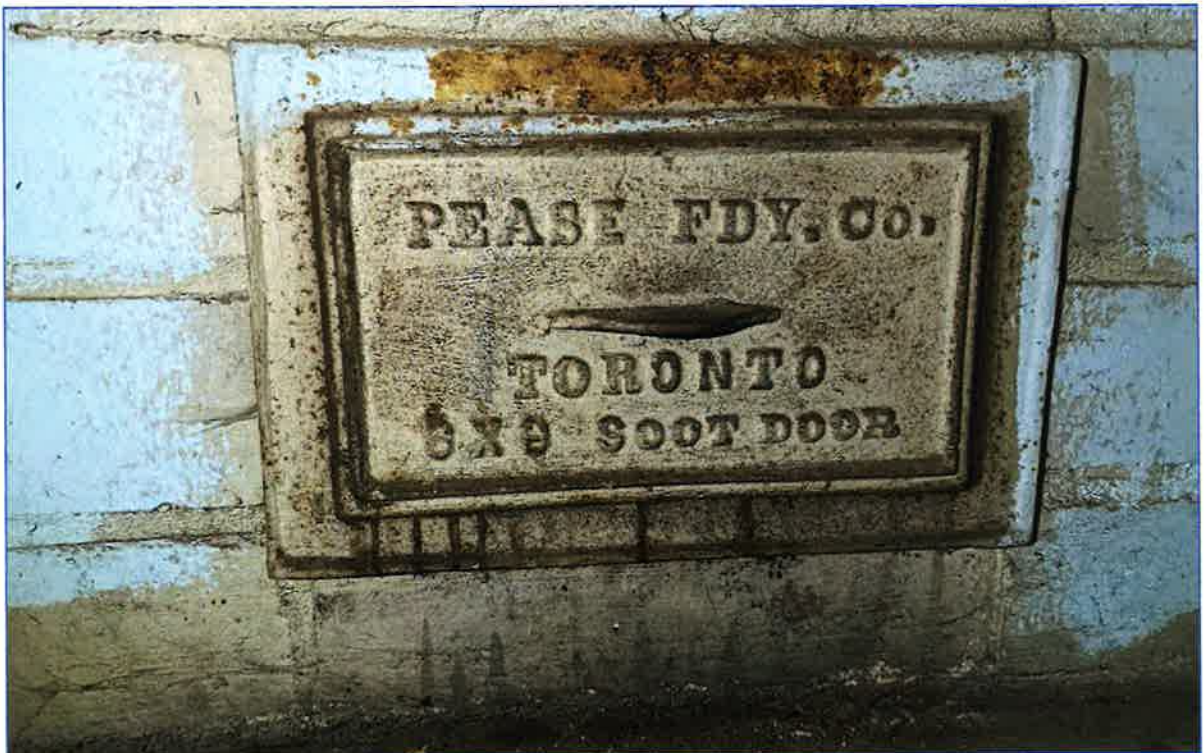
Photo 29: View of soot door on chimney
