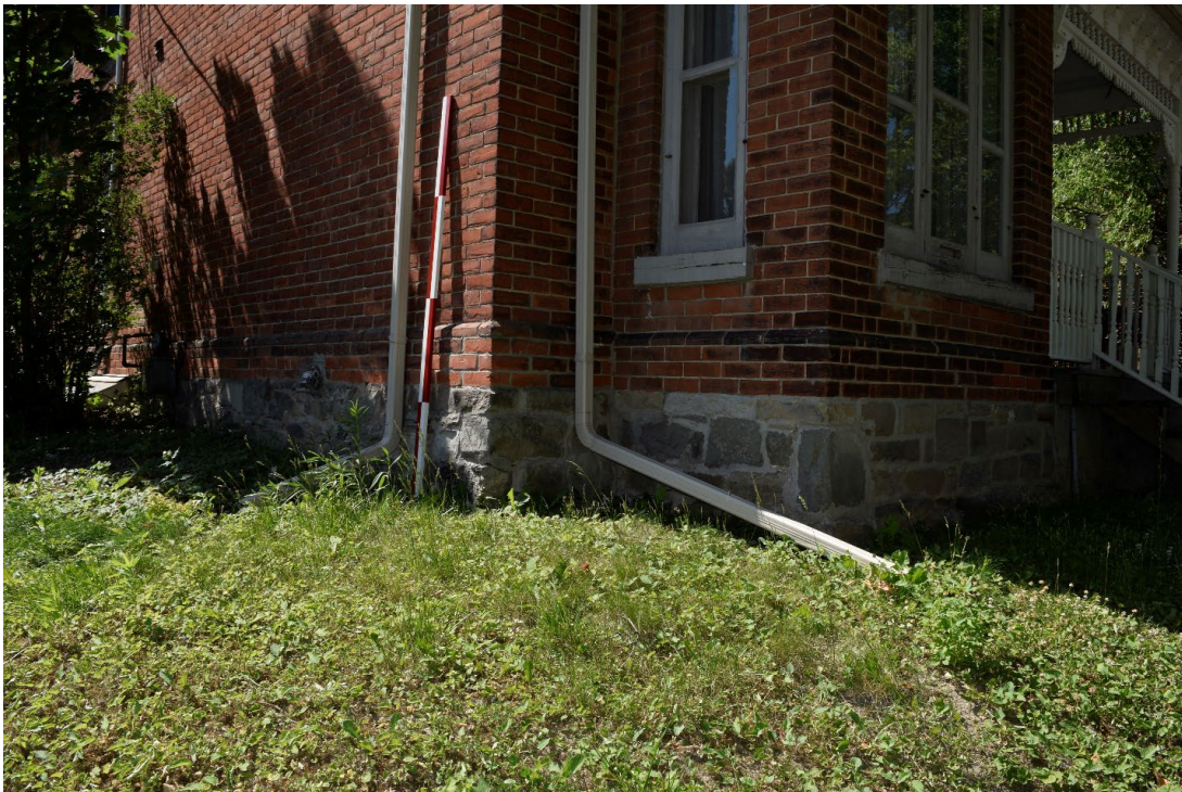
Figure 20: Detail of field stone foundation
