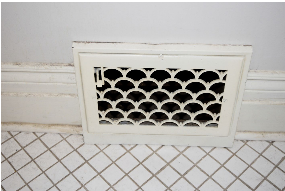
Figure 46: Example of original metal heat register
