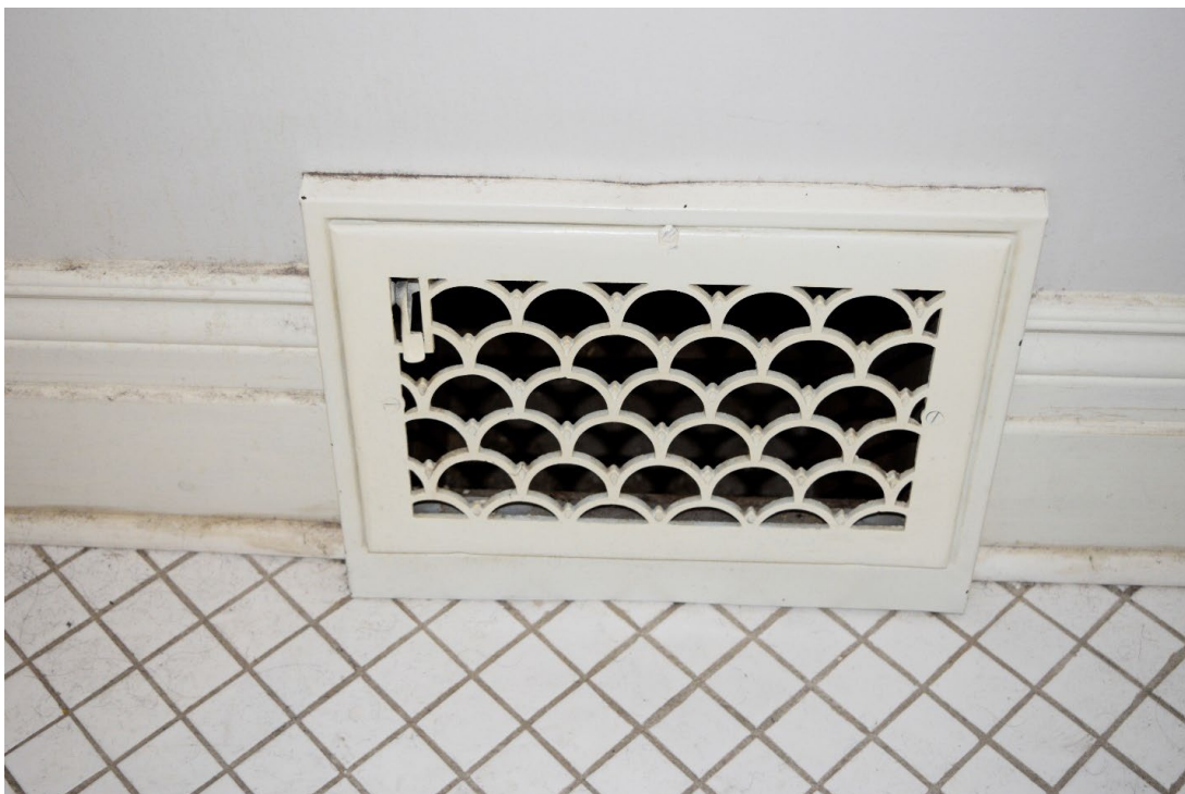
Figure 46: Example of original metal heat register
