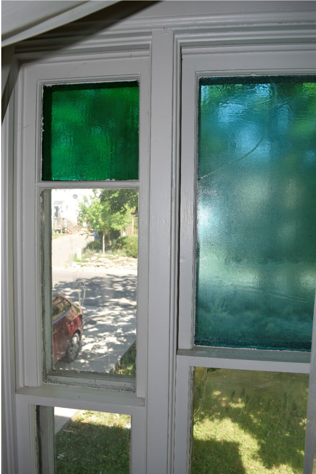
Figure 48: Original multi-coloured glass as seen in original 'Queen Anne' style bay window.
