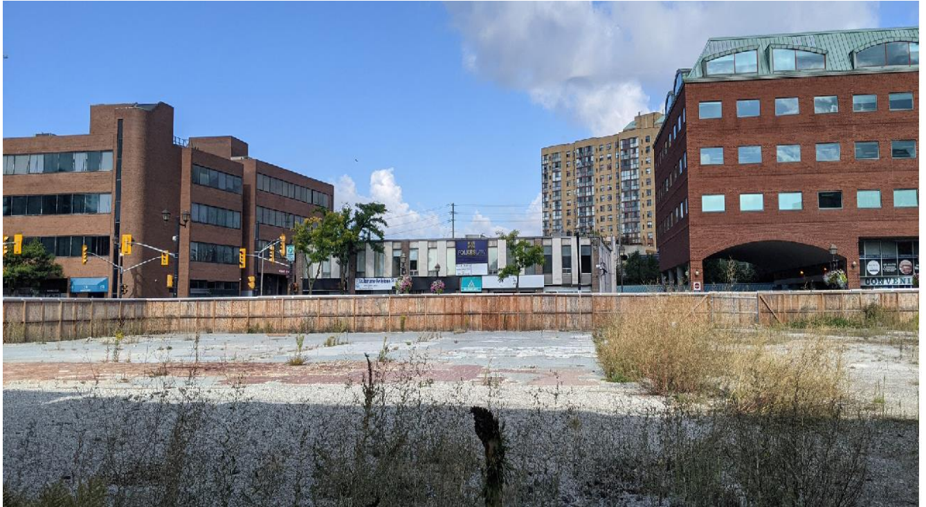
The existing site previously had a commercial building at 21 Nelson which was demolished in 2019 leaving only the foundations and slab on grade.
