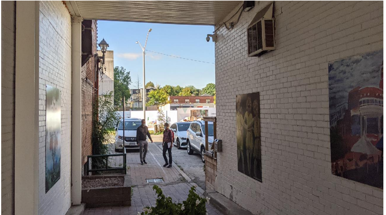
Existing site condition: view from Diplock Lane showing the existing connection through an opening under the shops from Main Street
