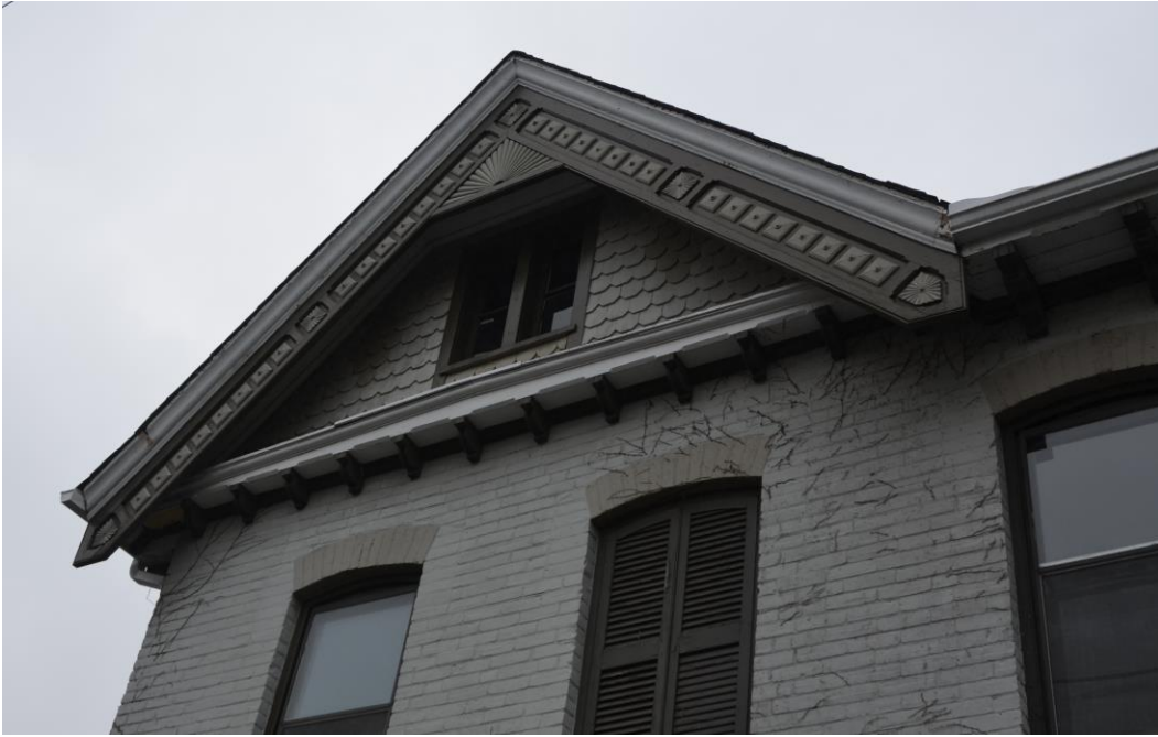
Figure 10: Detailing on front gable (Source: City of Brampton, 2019)
