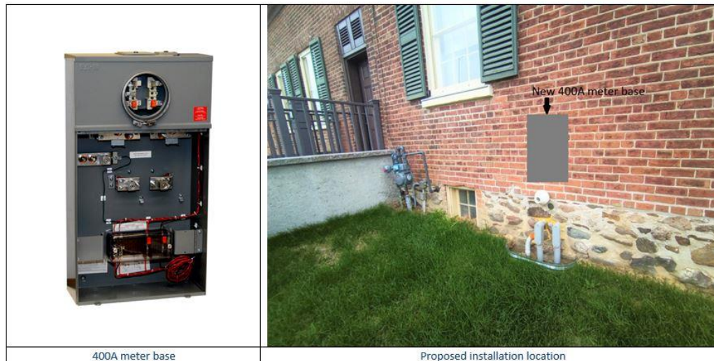
Figure 1: North Elevation, Bovaird House. Installation of a 400-meter hydro base
