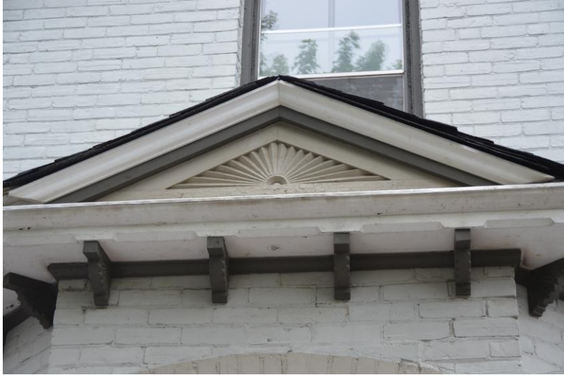
Figure 12: Sunburst detail on gable above bay window, east elevation (Source: City of Brampton, 2019)
