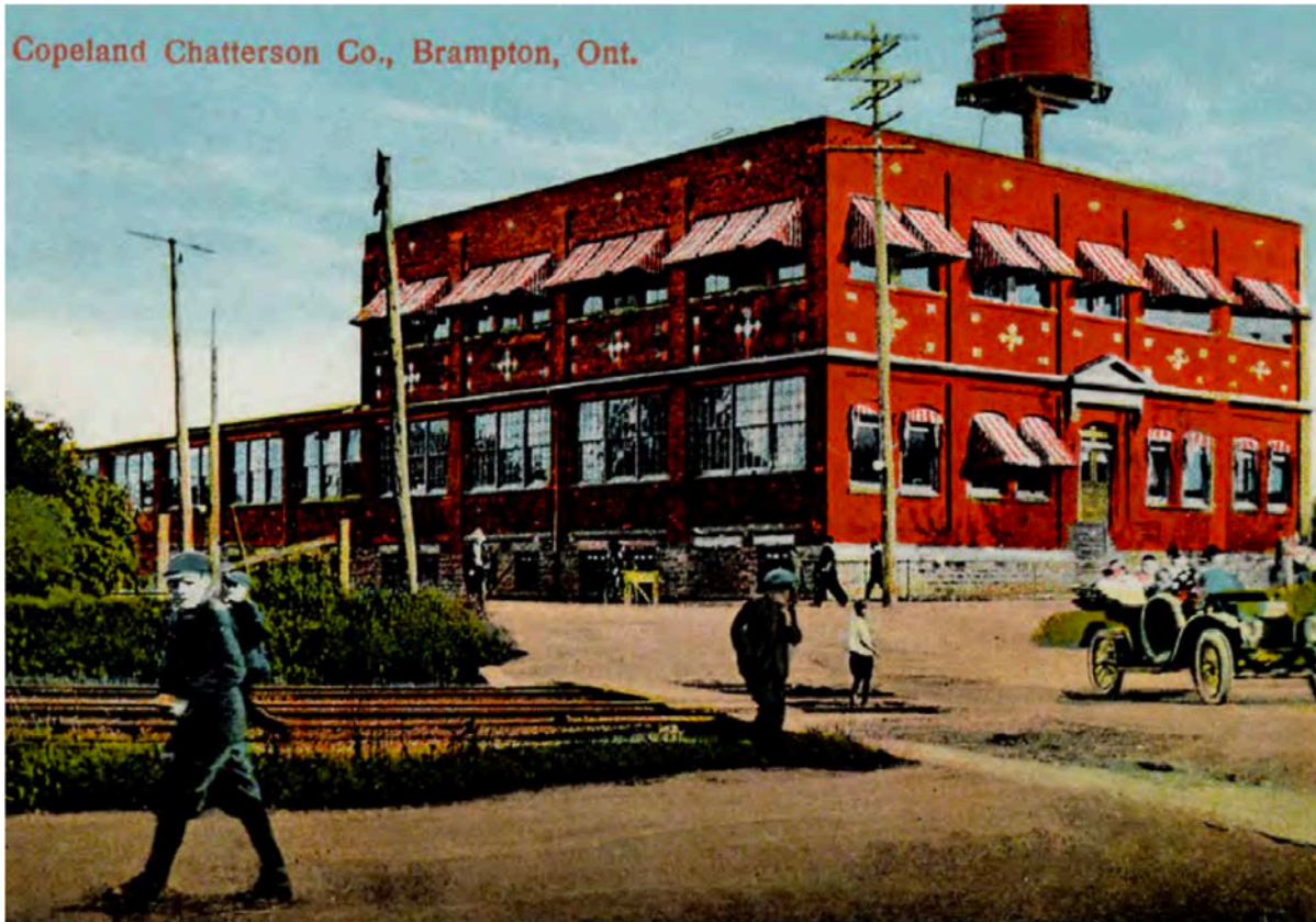
Postcard image of the building with 1914 addition (Source: Peel Archives).
