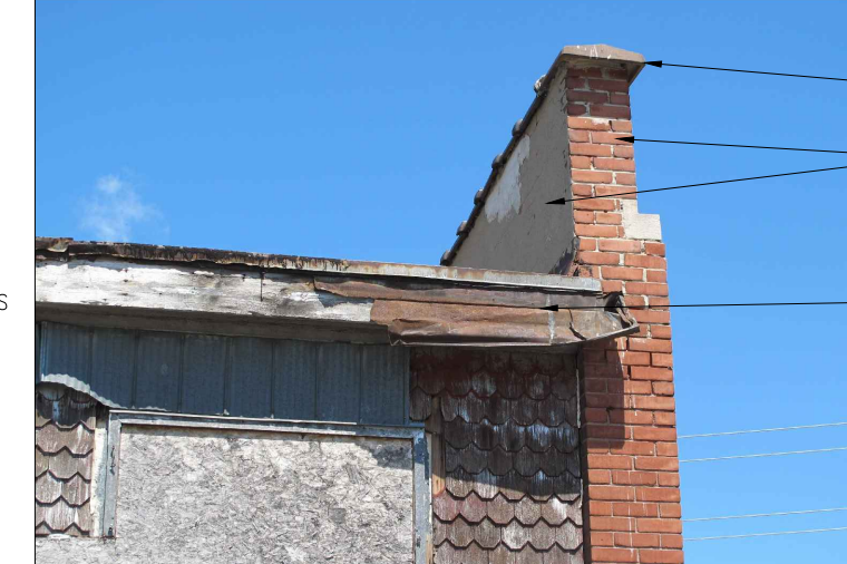
South Facade @ Parapet 3 HA202
