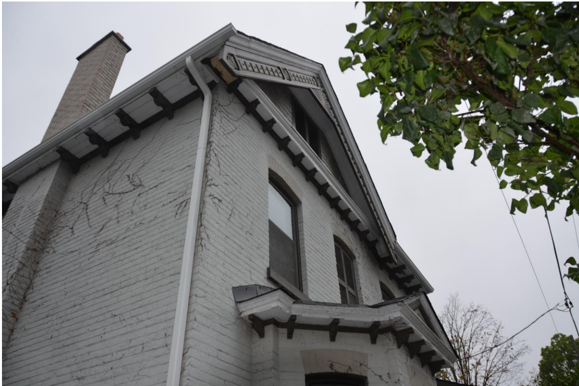
Figure 7: Brackets on eaves. Front and east elevations (Source: City of Brampton, 2019)
