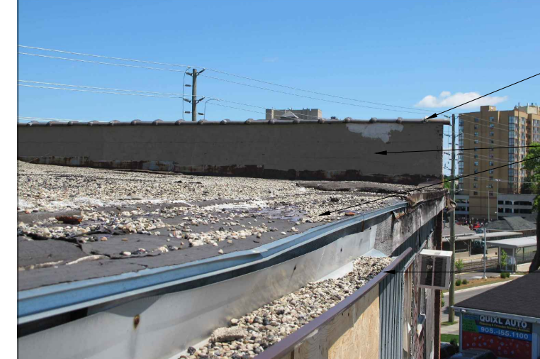
Parapet Roof 4 HA202
