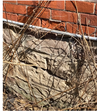
Severe deterioration of the stone foundation (ERA, 2023).
