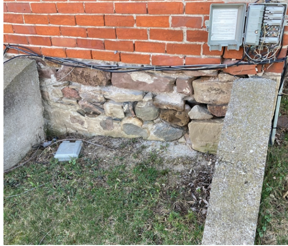
Severe deterioration of foundation pointing (ERA, 2023).
