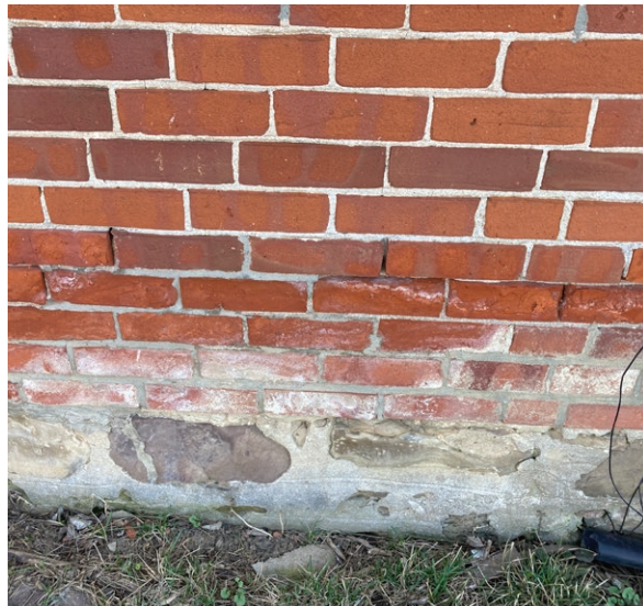
Efflorescence and spalling (ERA, 2023).
