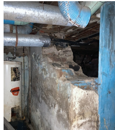
Damaged rubble foundation wall (ERA, 2023).
