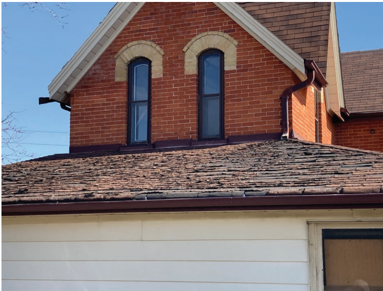
Defective shingles on the rear addition (ERA, 2023).
