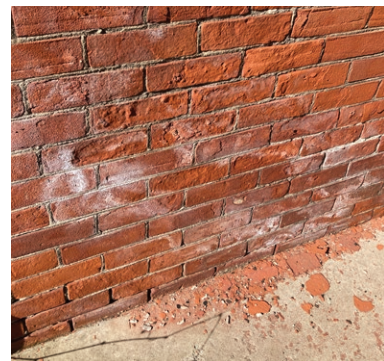
Masonry spalling on the porch level (ERA, 2023).
