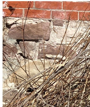
Severe deterioration of the stone foundation (ERA, 2023).
