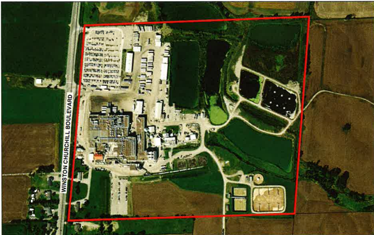
Figure 1 – Air Photo Poultry Processing Plant
