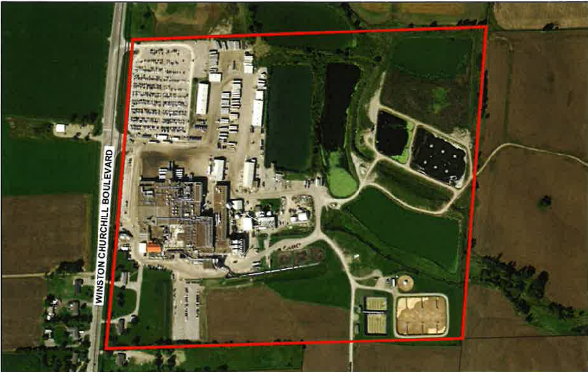
Figure 1 – Air Photo Poultry Processing Plant
