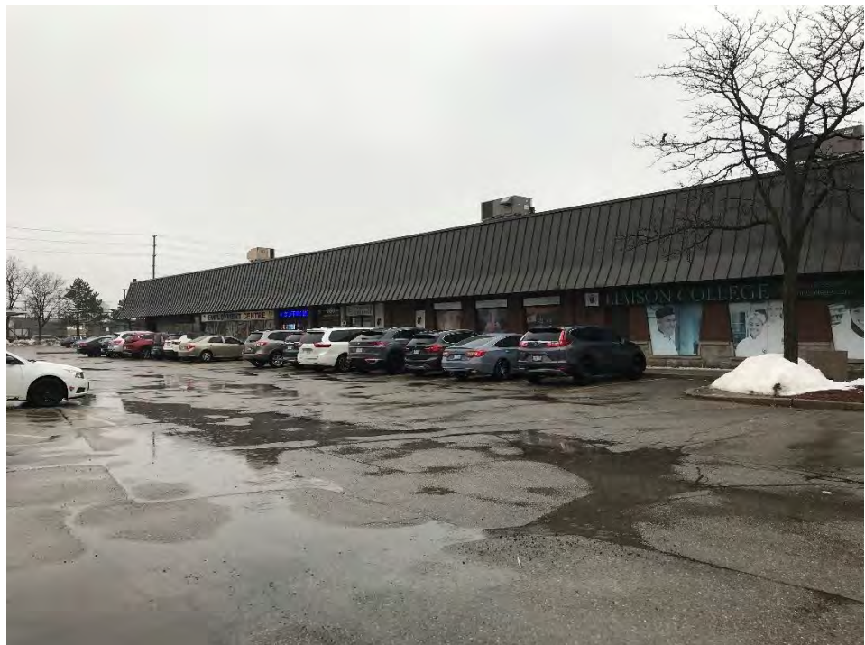
Image #4 Looking southwest along the east side of the building
