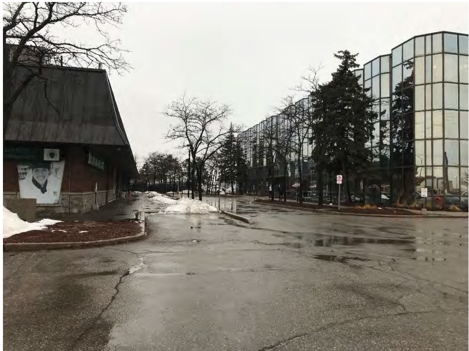
Image #5 Looking west at the exterior northeast corner of the building
