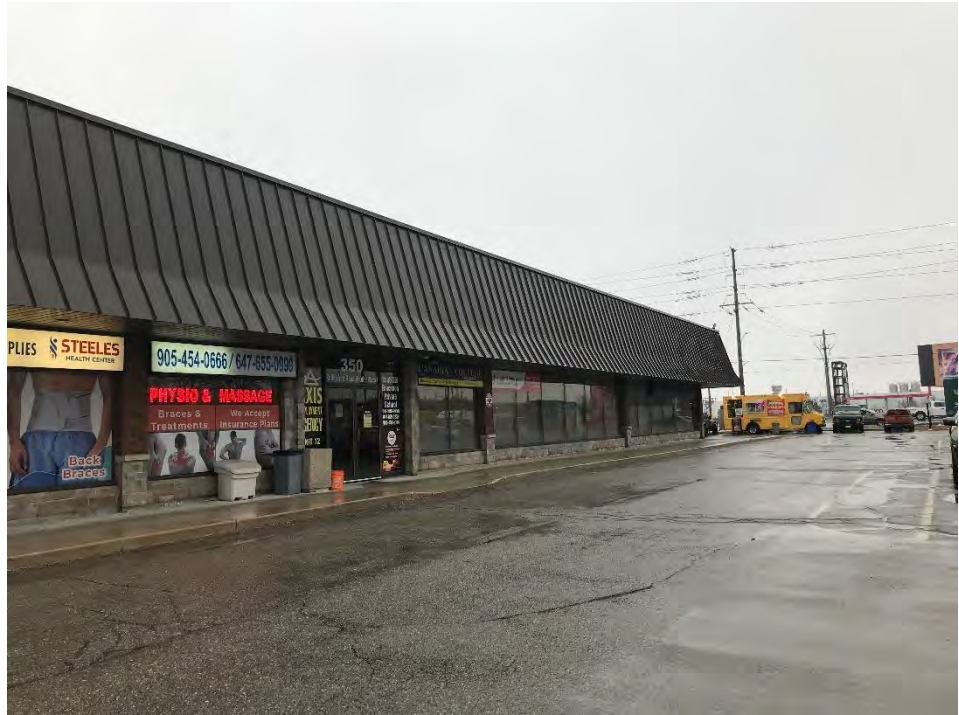
Image #3 Looking northeast at the south side of the building
