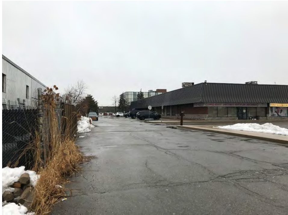
Image #7 View looking north along the west side of the building
