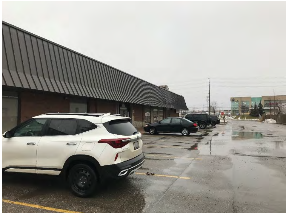
Image #6 View looking south along the west side of the building
