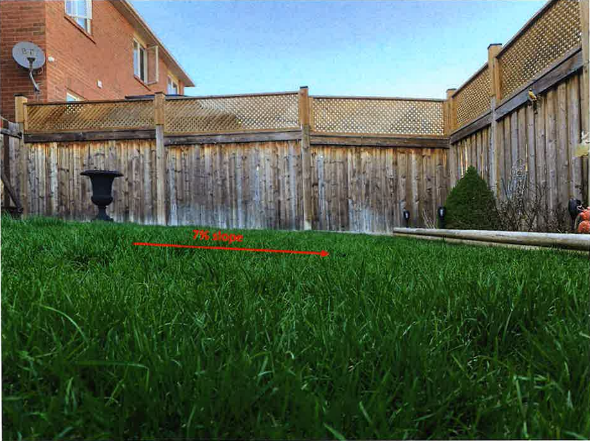
Picture 4: Slope of backyard grade towards rear fence (7% avg. slope approximately)
