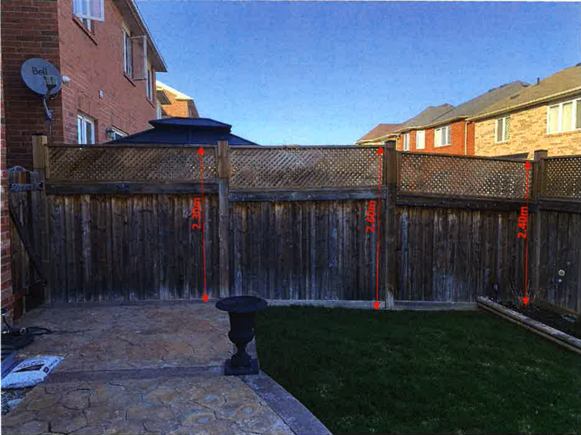
Picture 3: Side fence – East
