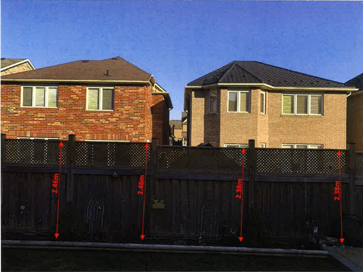
Picture 1: Rear fence - South
