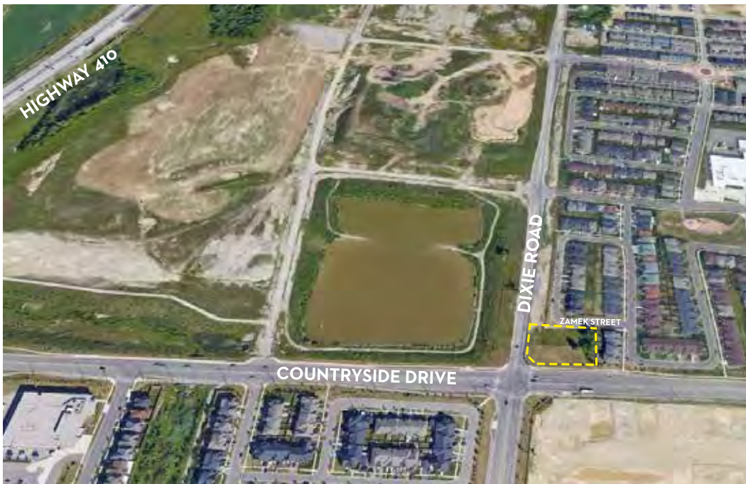
Aerial view of site with buildings that are subject to the Heritage Interpretation Plan in dashed outlined (annotated by Somerville Planning).
