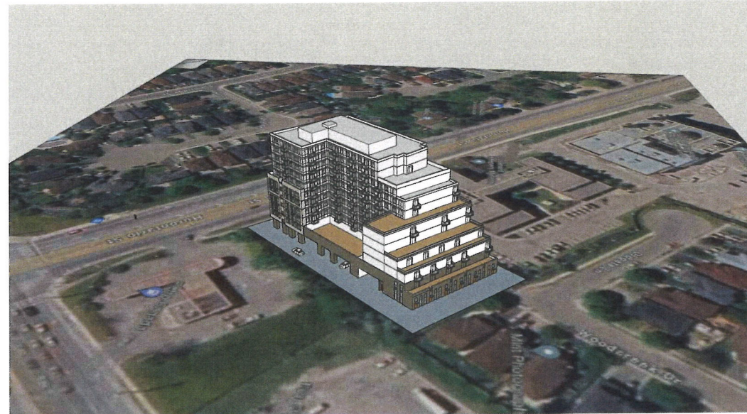
AERIAL VIEW - SOUTH EAST
