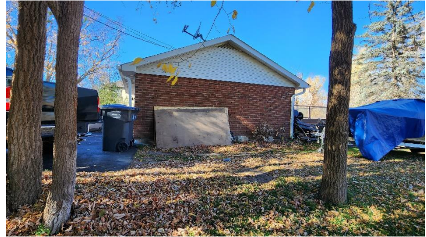
Figure 14 - East elevation showing the brick wall with siding filled gable a ridge vent of the end wall of the garage. (RHC 2022)
