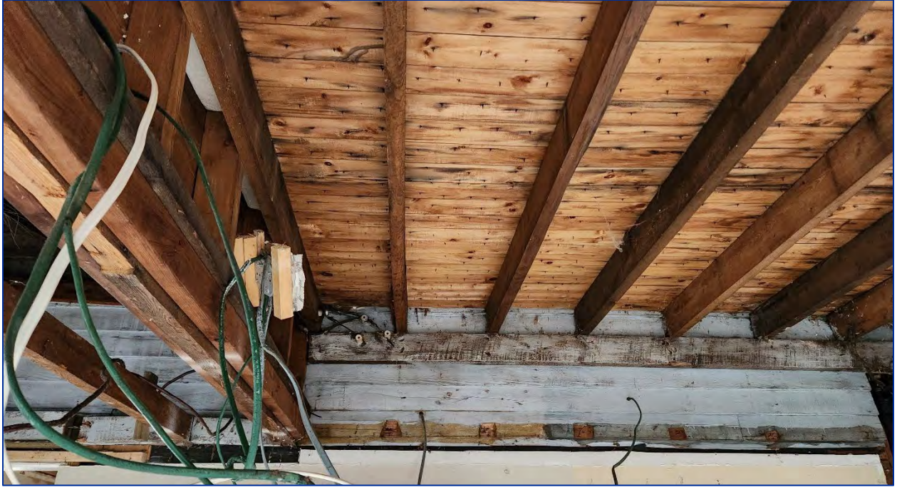
Photo 16: View of the basement showing wooden beams and joists supporting floorboards.
