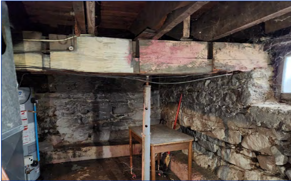
Photo 37: View of the basement showing the fieldstone foundation and a large sawn timber beam supporting wooden joists.
