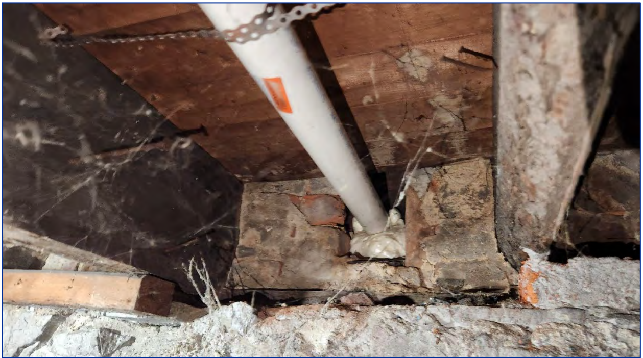
Photo 40: View of piping through a hewn section of a large timber beam.
