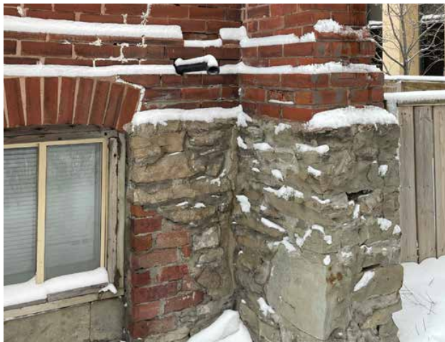
Fig. 2.14. Incompatible repairs of foundation walls and open joints.
