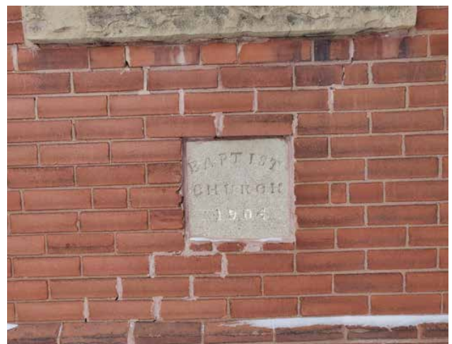
Fig. 2.23. Cornerstone in fair condition with minor chipping around the edges.
