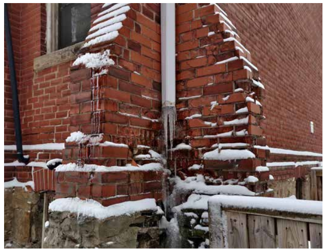
Fig. 2.10. Significant deterioration at buttresses due to water ingress.
