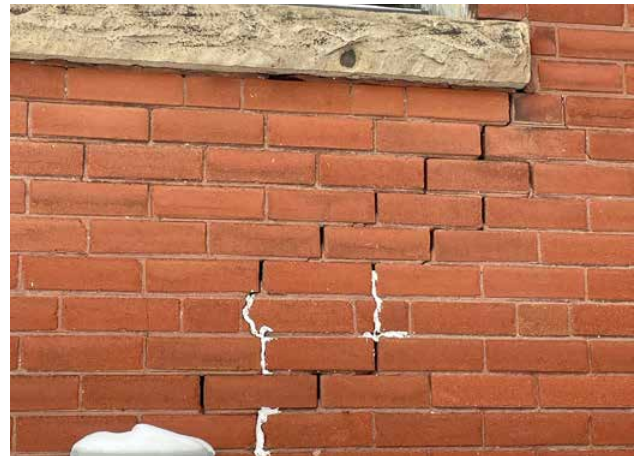
Fig. 2.2. General condition of brick throughout, displaying signs of deterioration, structural cracks, open joints and incompatible repairs.
