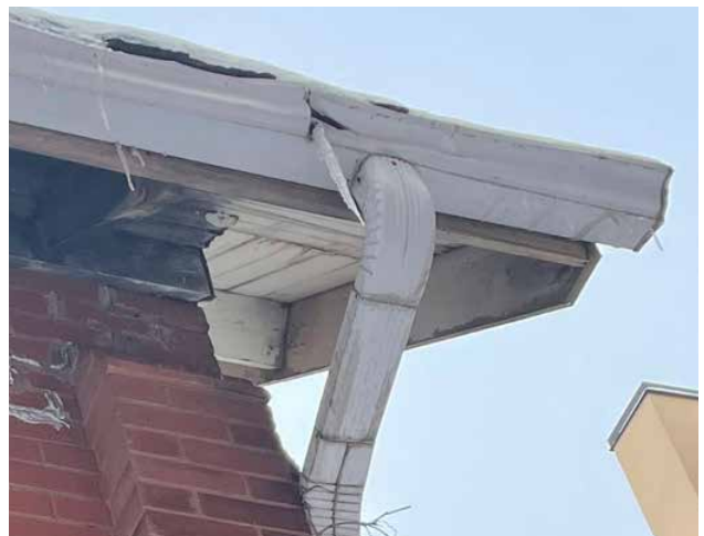
Fig. 2.35. Gutters and downspouts in fair condition.
