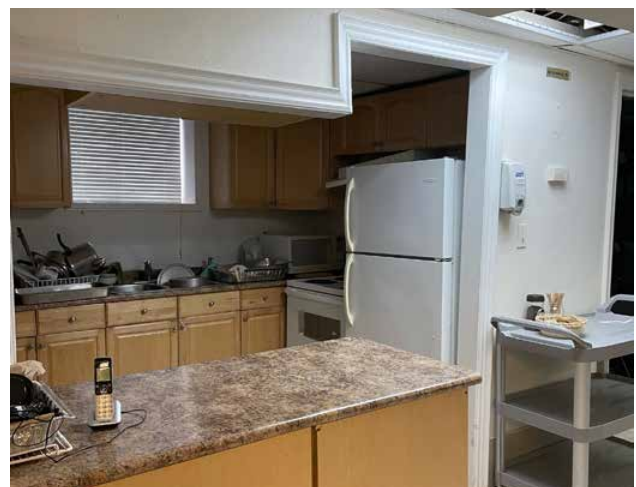
Fig. 2.41. Finished kitchen in the basement.
