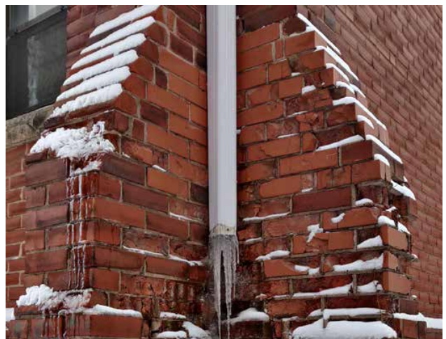
Fig. 2.27. Condition of brick at southeast corner, which requires repair or replacement.
