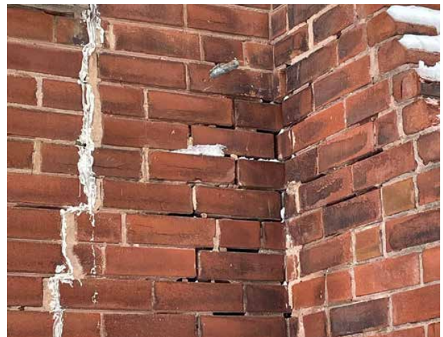
Fig. 2.3. General condition at inside corners: open joints, deteriorated mortar, incompatible repairs.
