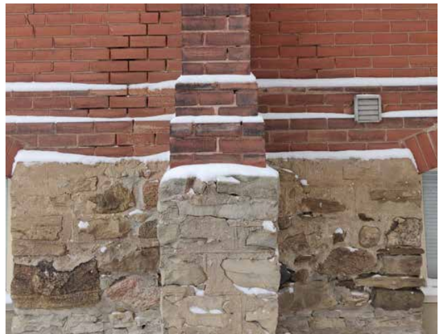
Fig. 2.17. General condition of foundation walls: open joints and incompatible repairs.
