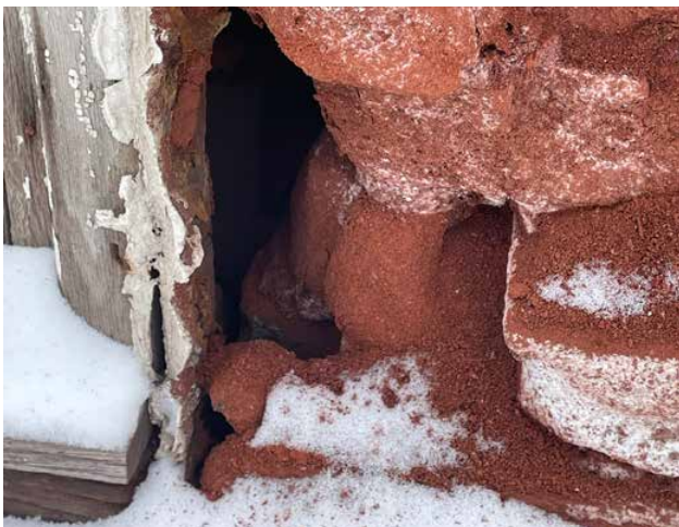
Fig. 2.7. Severe deterioration of masonry at lower portion of front entrance wall.
