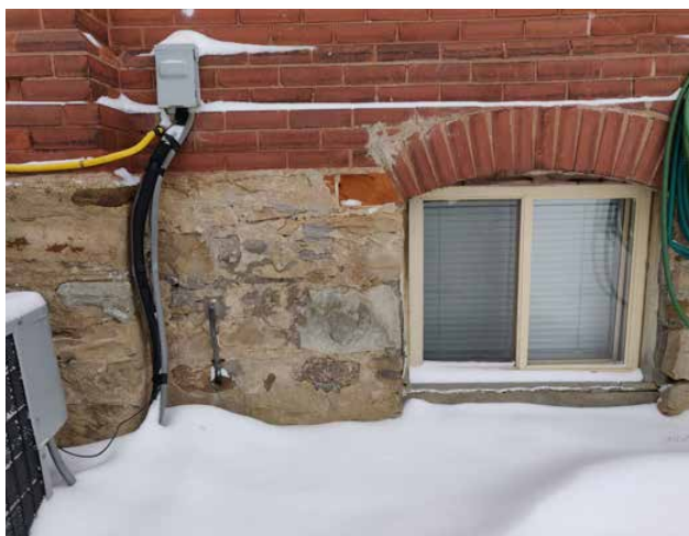
Fig. 2.15. Foundation walls at basement window: incompatible repairs and spalling.
