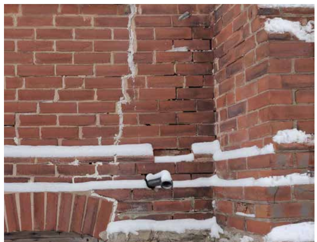
Fig. 2.9. General condition of masonry condition at inside corners. Deteriorated mortar, structural cracks, and incompatible repairs.
