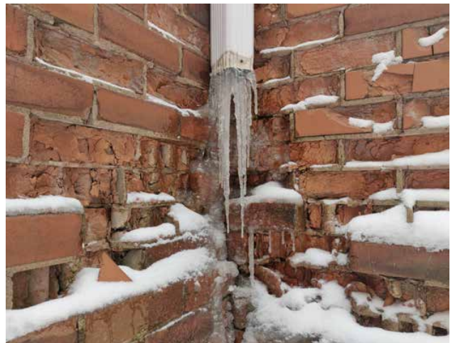
Fig. 2.11. Close-up of inside corner at buttresses: damaged masonry due to water ingress.
