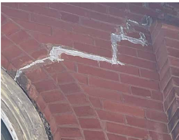
Fig. 2.20. Typical condition at window openings: structural cracks and incompatible repairs.
