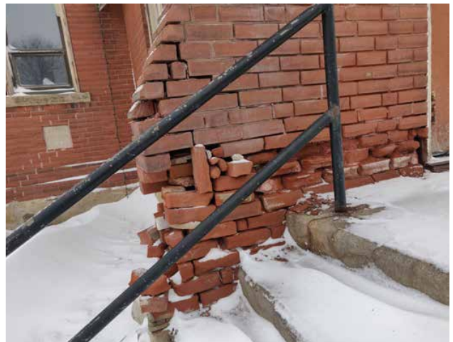
Fig. 2.26. Condition of brick at front façade and buttress, which requires reconstruction.
