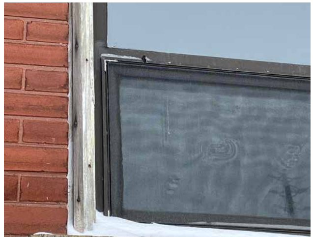
Fig. 2.29. Windows have been replaced throughout.
