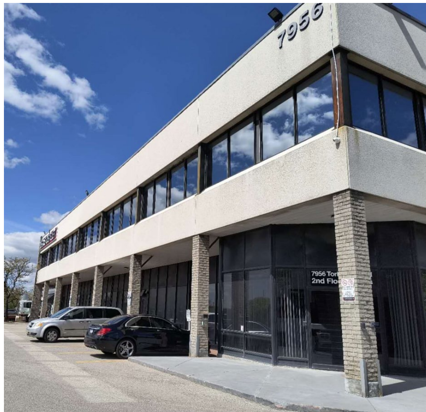
7956 Second floor entrance
