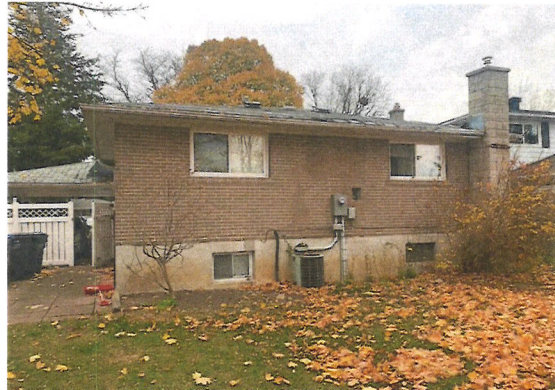
Figure 2: Rear View of Existing House
