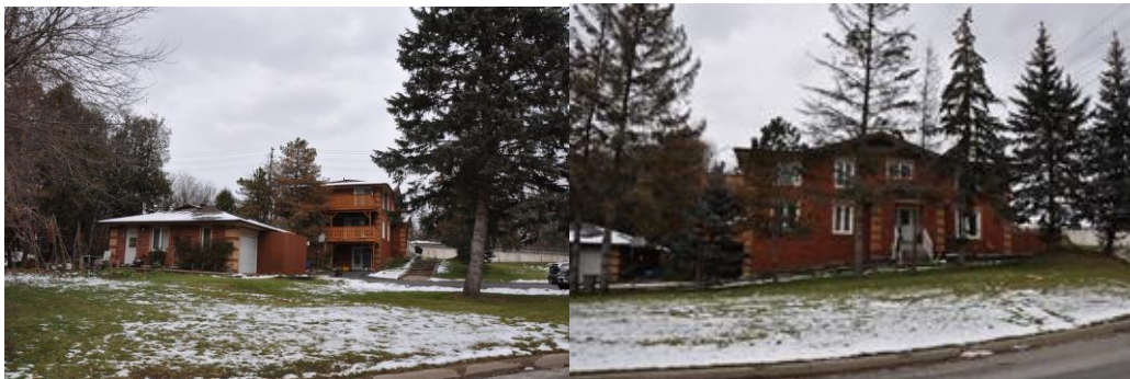
4.1.6.H - 22 River Road – (RR CHL Zone 1) Credit River exposure
