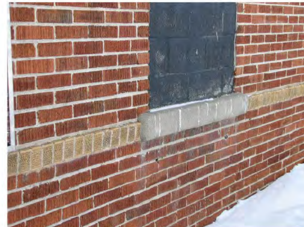
Details showing wire cut buff brick course providing dichromatic decorative relief on front façade.
