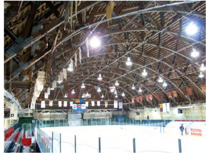
Views of the timber frame arena roof system designed by Norman Otto Hipel.
