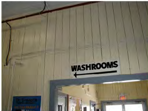
Detail showing beaded tongue in groove wood paneling throughout main hallways and lobby area, along with simple planks used as door surrounds. This photo is taken near the east entrance.
