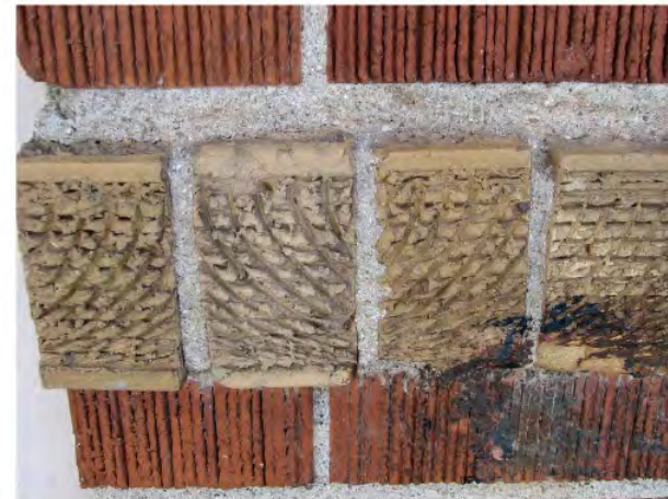
Details showing wire cut buff brick course providing dichromatic decorative relief on front façade.
