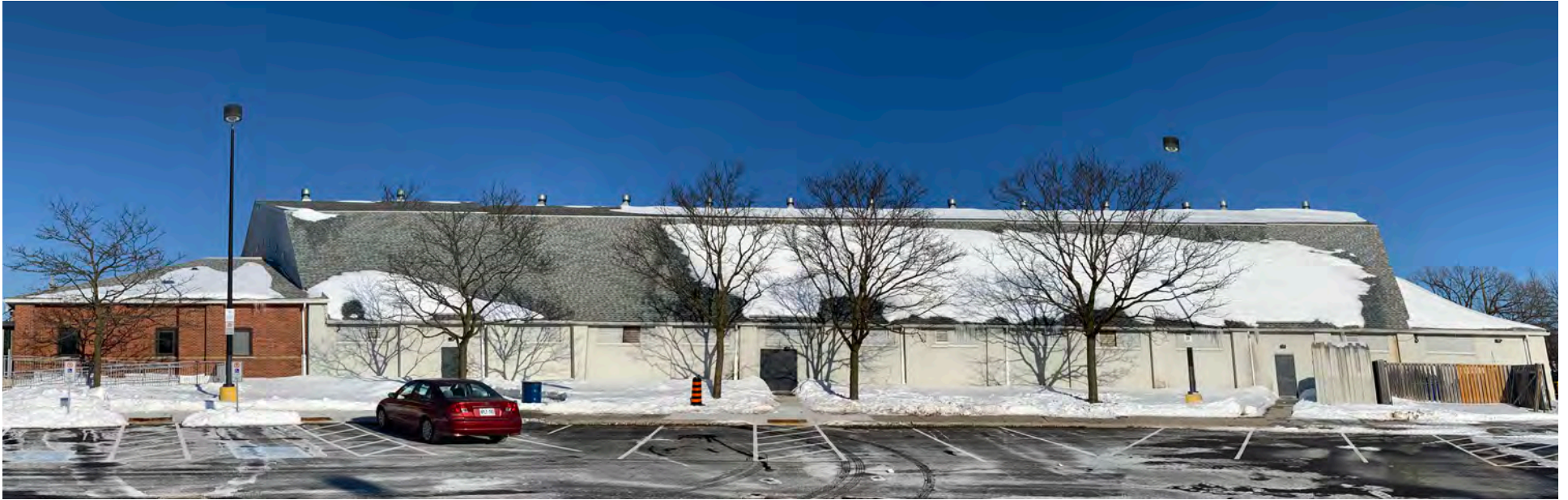
View of West Elevation from Parking Lot Source: ATA Architects, 2022
