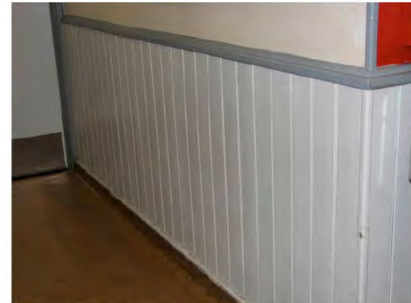
Detail of the tongue in groove wood wainscoting located throughout main hallways and lobby area.
