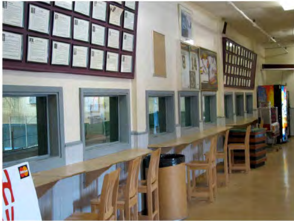
Detail in main lobby showing counter and spectator windows facing the ice rink.
