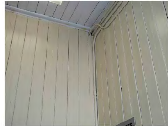
Detail of beaded tongue in groove wood paneling on walls and ceiling in main hallways. (east entrance).
