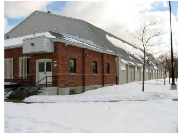
Views of west side of building showing barn-like roof profile and side elevation with repeating buttresses.
