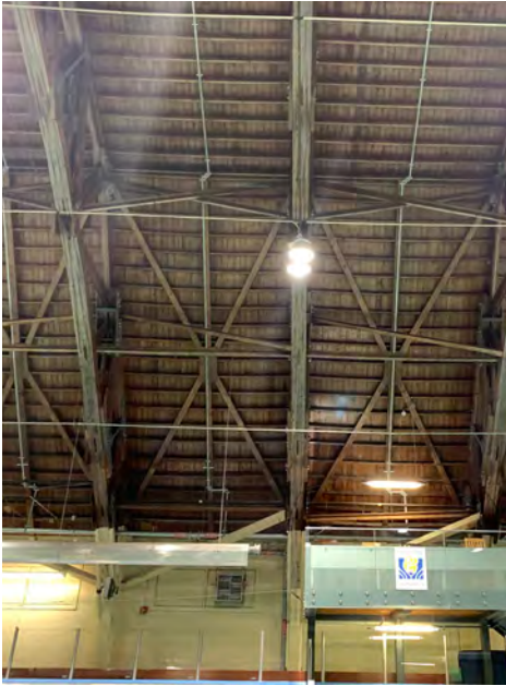
View of Detail of the roof structure Source: ATA Architects, 2022
