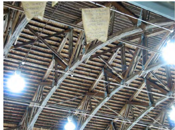
Views of the timber frame arena roof system designed by Norman Otto Hipel.
