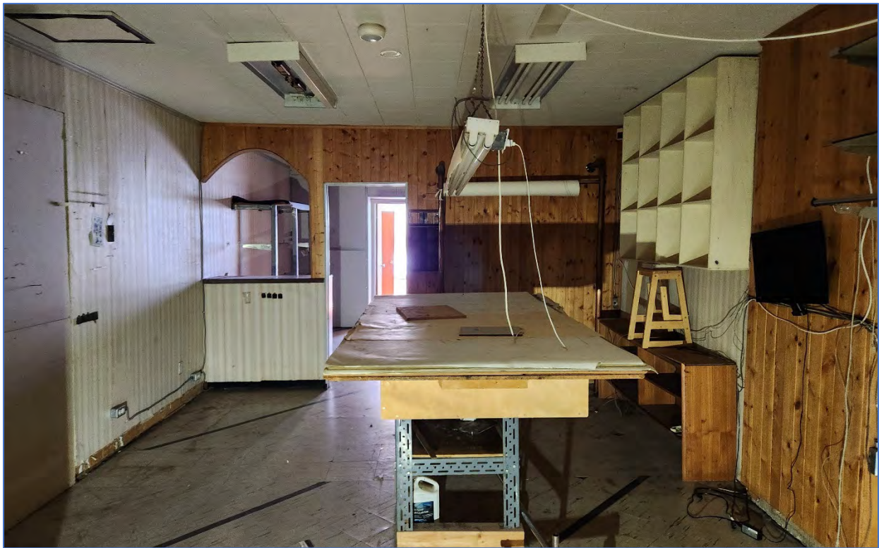
Photo 36: View southwest showing the workroom
