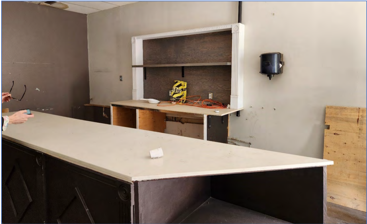
Photo 42: View north showing the open storefront at the southwest side of the building
