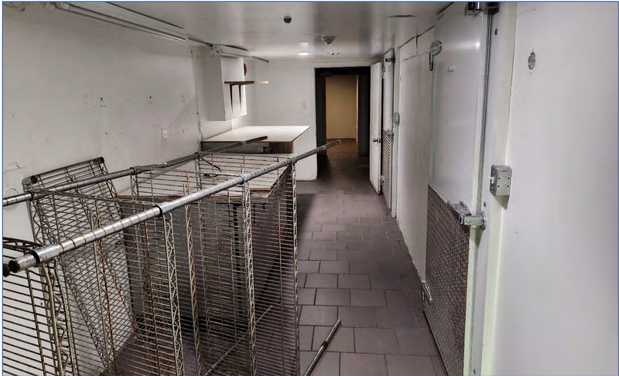
Photo 28: View southwest showing the basement hallway
