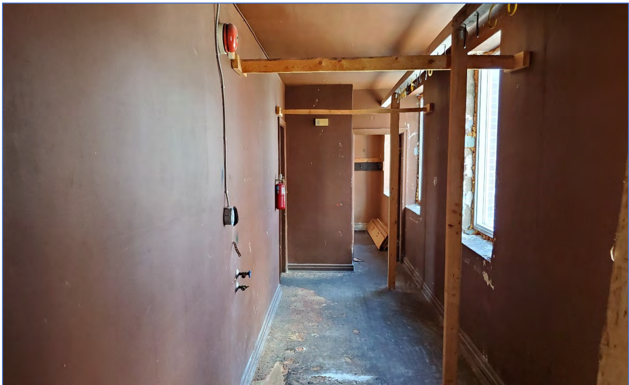
Photo 72: View northwest showing the second storey hallway
