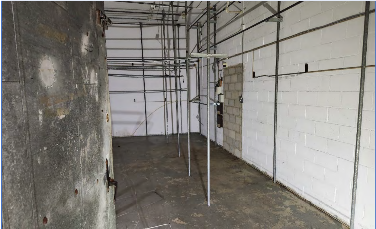
Photo 35: View northeast showing the eastmost storage room
