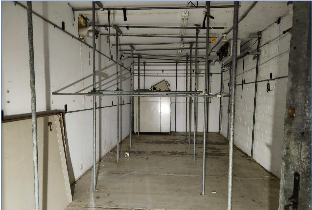
Photo 39: View northeast showing the eastmost storage room
