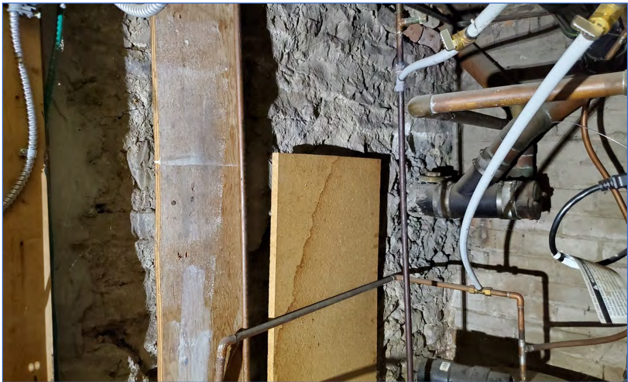
Photo 51: View showing part of the building's stone and brick foundation
