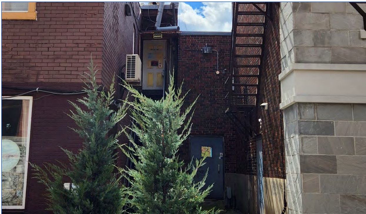
Photo 53: View southwest showing the building at 54 Main Street North's northeast (rear) elevation
