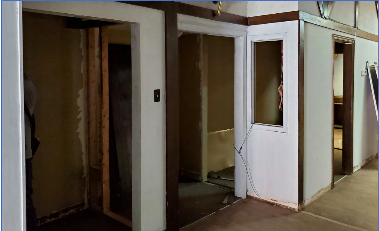
Photo 13: View southeast showing the office (right) and storage room (left)
