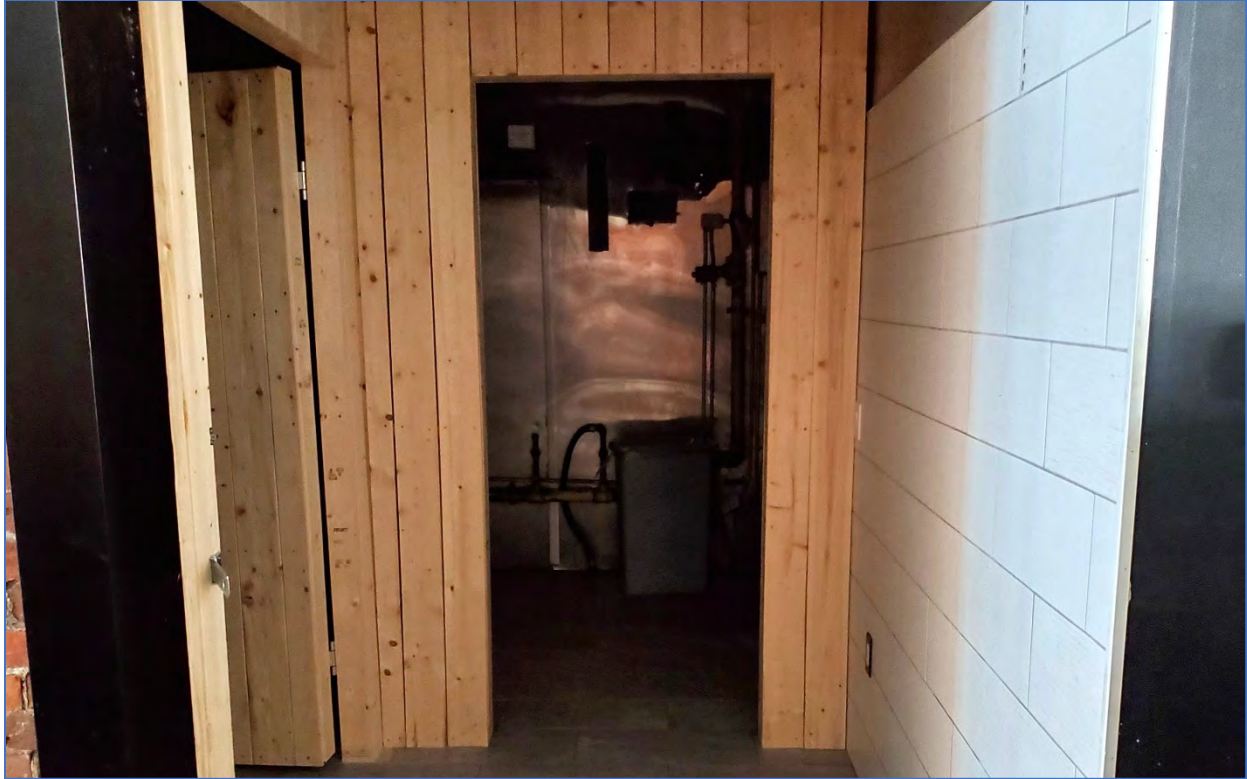
Photo 20: View northwest showing the room in hallway's southmost corner
