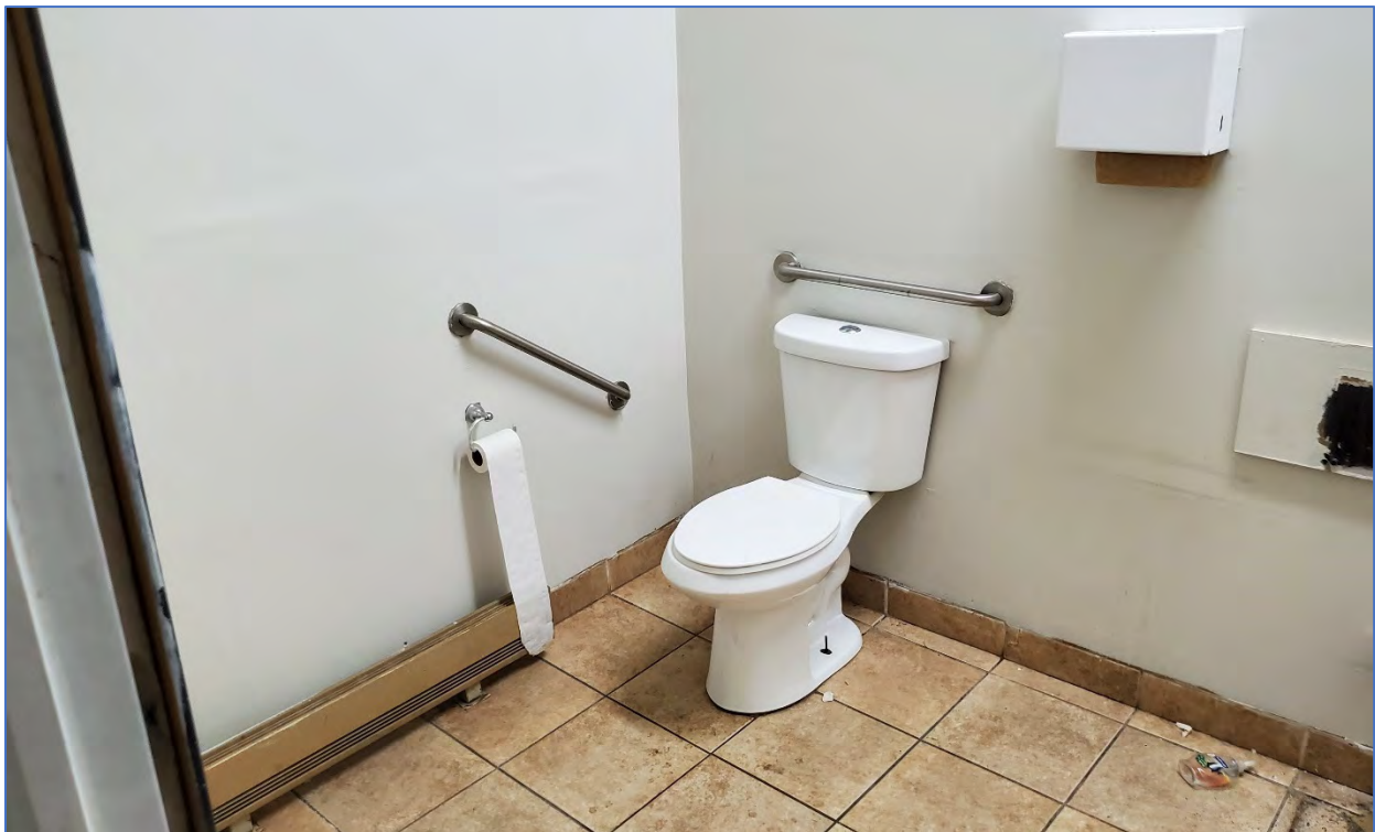
Photo 45: View southeast showing the washroom
