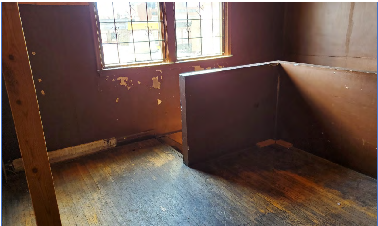
Photo 68: View southwest showing the west suite's landing
