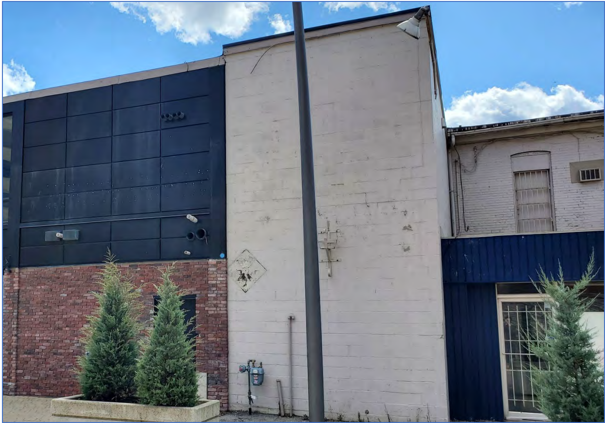
Photo 31: View southwest showing the building at 42 Main Street North's northeast (rear) elevation
