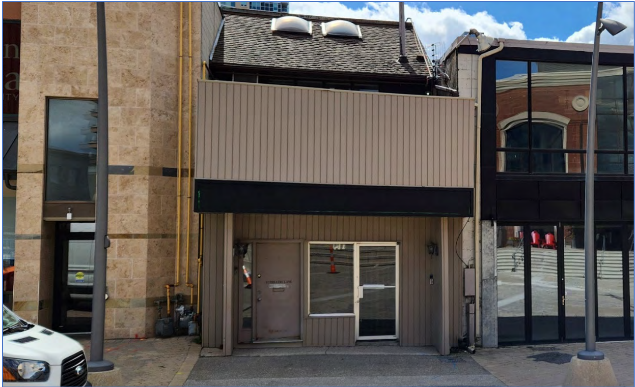
Photo 10: View southwest showing the building at 30 Main Street North's northeast (rear) elevation
