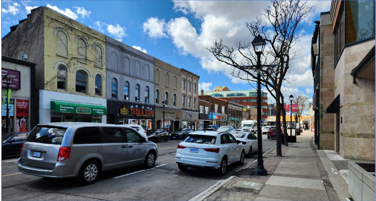
Photo 1: View northwest showing properties on the southwest side of Main Street North
