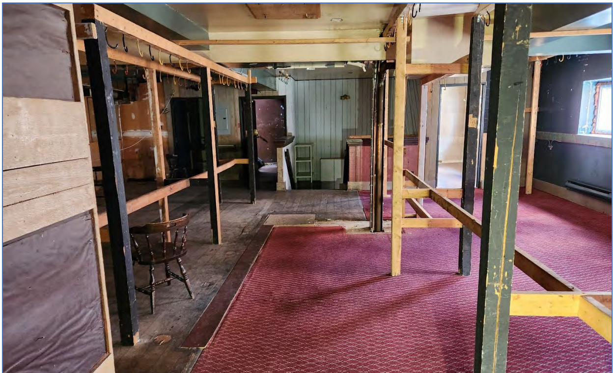
Photo 66: View northwest showing the mezzanine
