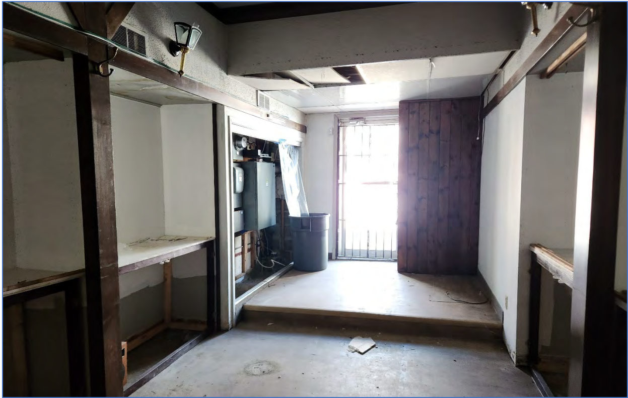
Photo 12: View northeast showing the northeast section of the main, open area
