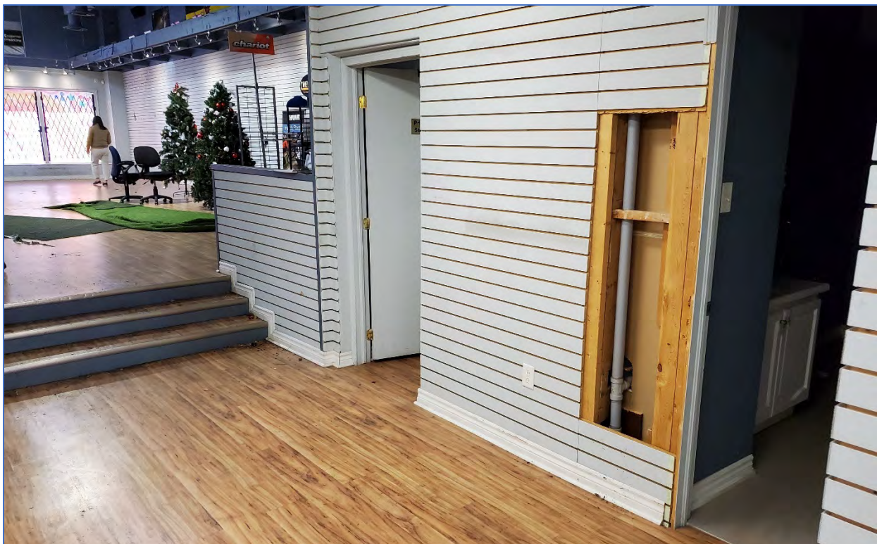
Photo 64: View southwest showing the office door (left) and washroom door (right)
