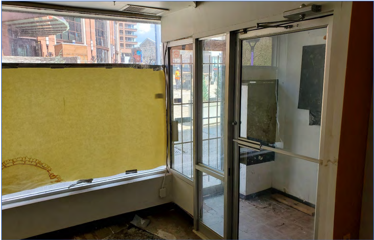
Photo 44: View north showing the vestibule
