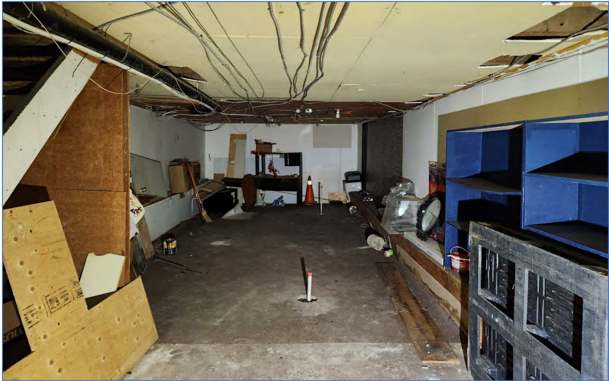
Photo 50: View southwest showing the basement
