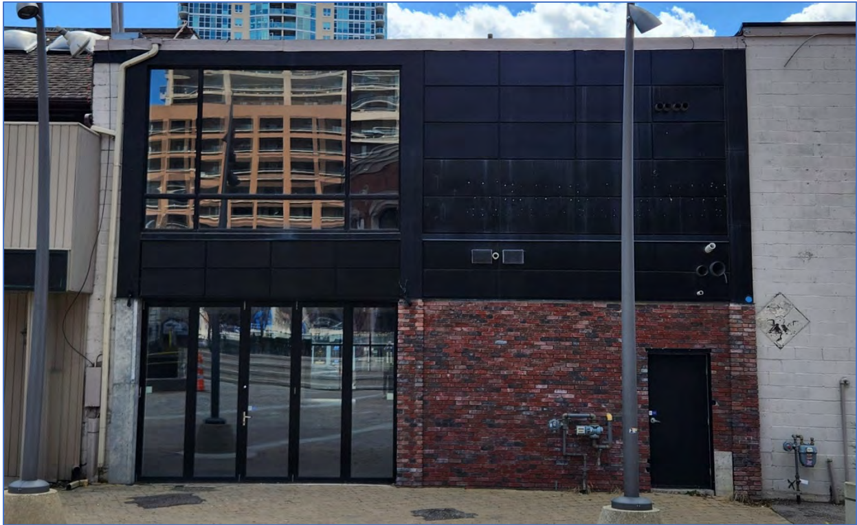
Photo 16: View southwest showing the building at 36-38 Main Street North's northeast (rear) elevation
