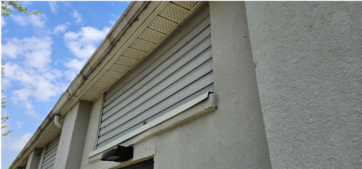
Fig. 5.3: View of infilled horizontal windows and metal sills. Image: +VG Architects
