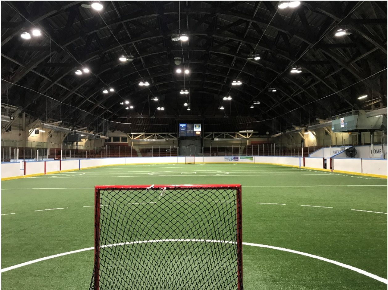
Fig. 2.1: View of arena playing surface with clear span Hipel Roof Truss. Image: +VG Architects
