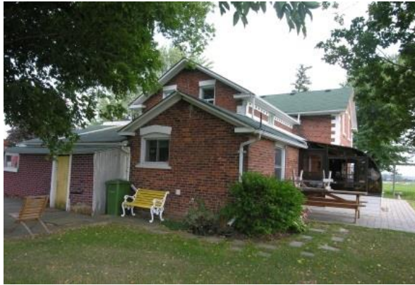
Figure 36 West elevation showing the numerous additions to the rear 'ell' of the side shed-roof additions (north and south), a glass greenhouse (south), the garage (north-west) and 1-storey gable-roof shed (south-west).
