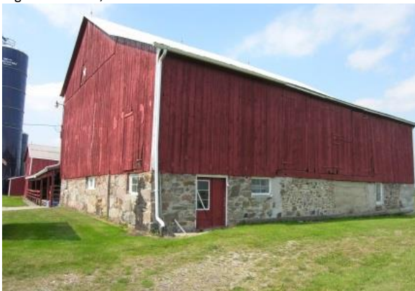
Figure 29 E-GS, east wall
