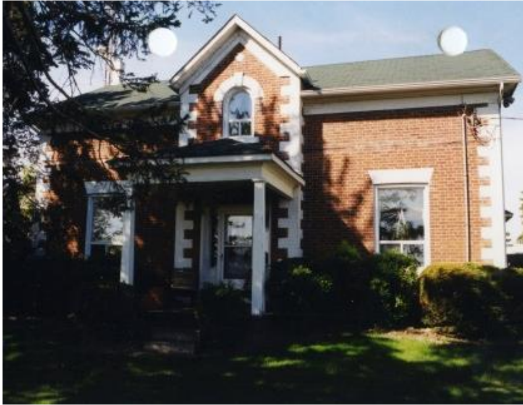
Figure 33 East elevation historically the formal main entry façade.
