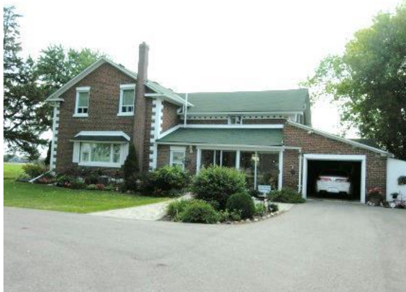
Figure 34 North elevation currently the front entrance showing numerous alterations/additions behind the original house form including the 'ell', an enclosed porch and garage.
