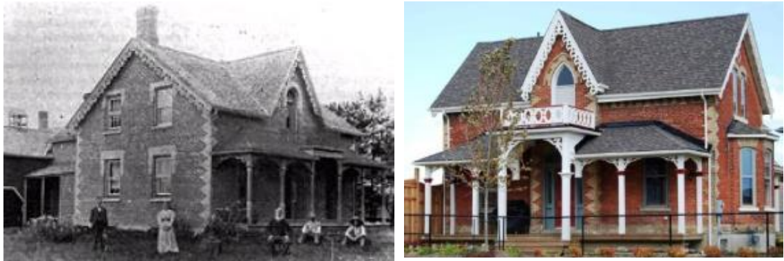
Figure 42 George Elliot Farmhouse (c.1860s), 120 Sled Dog Road, Brampton , example of Ontario Gothic Cottage
