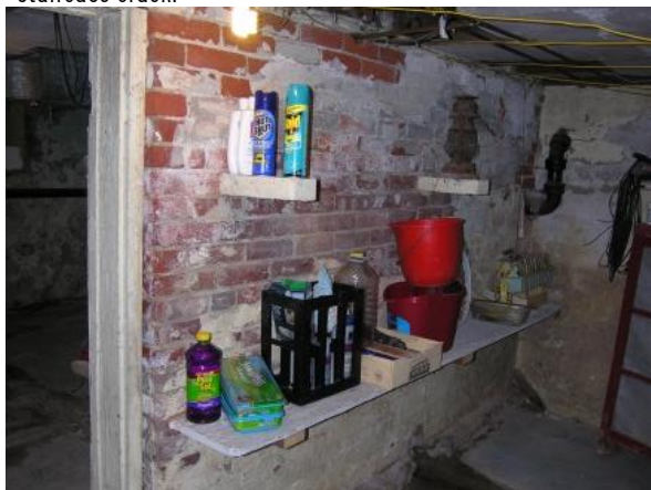
Figure 40 Basement interiors showing combination of wall construction in fieldstone and brick.
