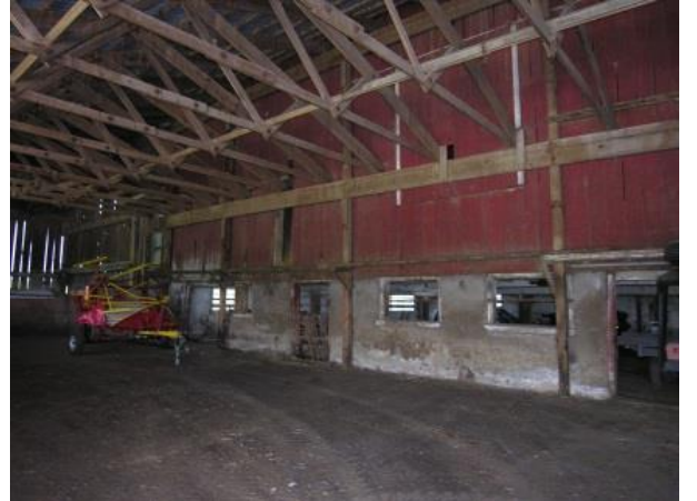
Figure 26 N-GS, south wall
