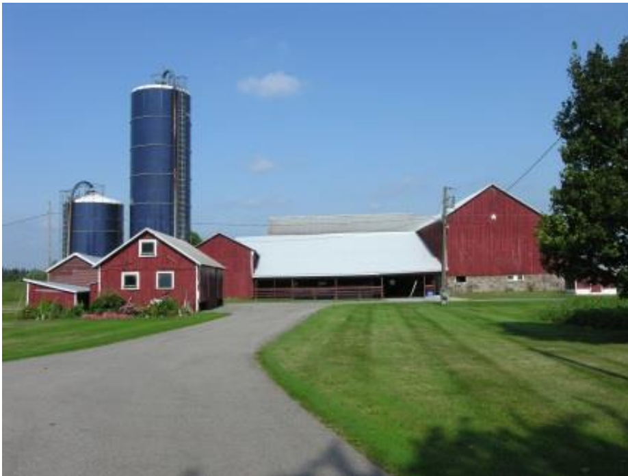
Figures 20 to 31 Barn Complex, Farm Structure-A, various views
