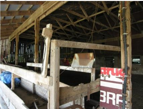
Figure 23 Central stall barn, interior framing
