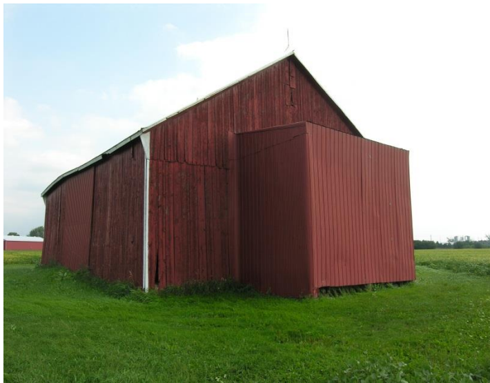
Figure 19 Farm Structure-6, Drive Shed
