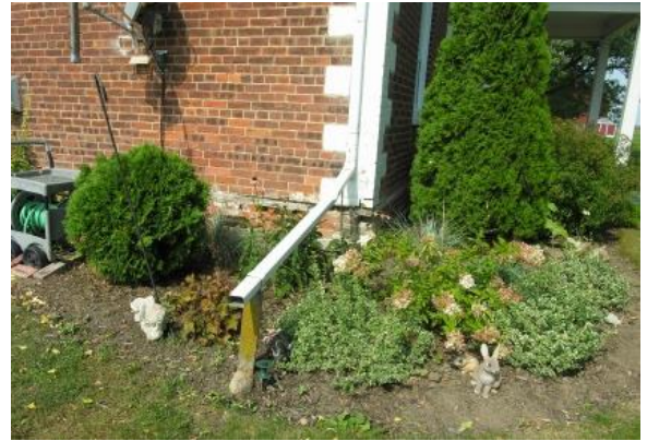
Figure 37 South-east corner, detail showing exposed wood plate at ground floor.
