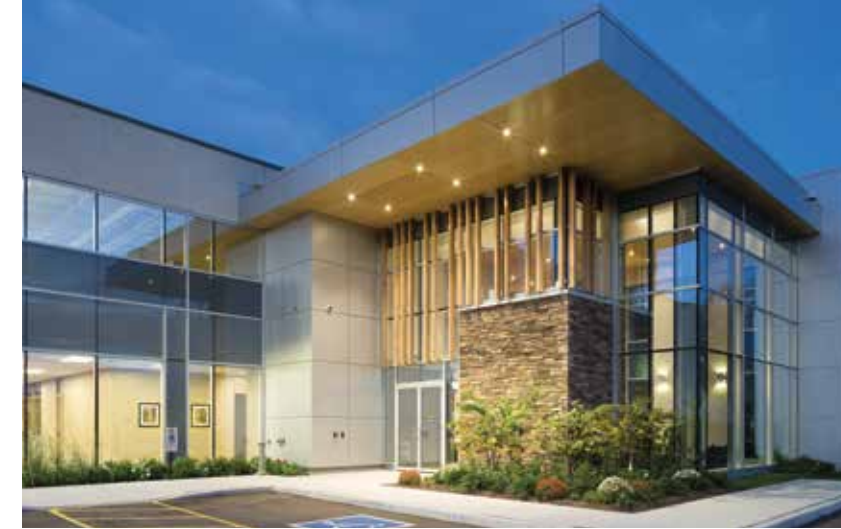
Fig 4.6.2 Building Entrance - Trailcon
