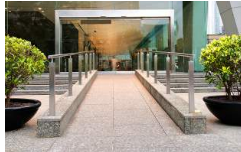
Fig 4.6.1 High Rise Accessible Entrance
