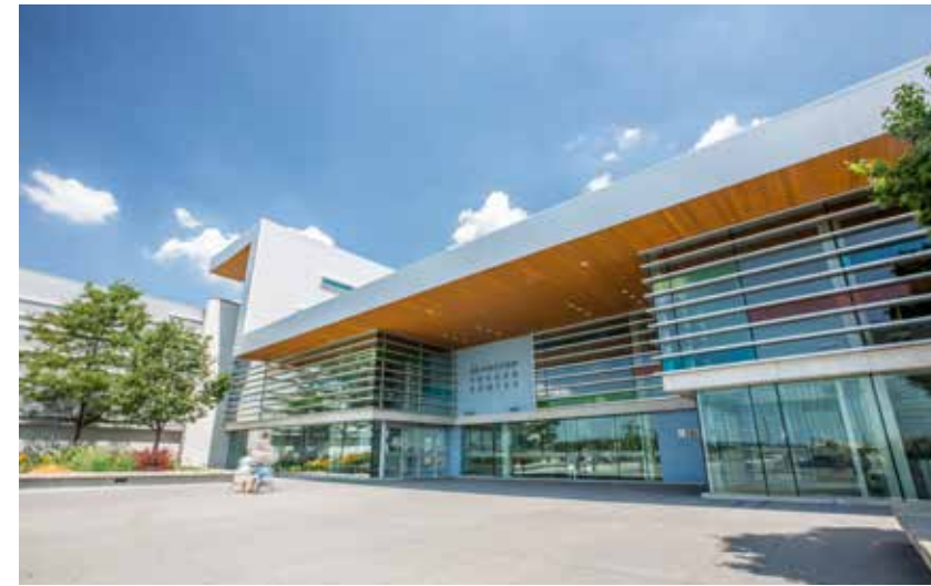
Fig 4.6.1 Brampton Soccer Centre Entrance
