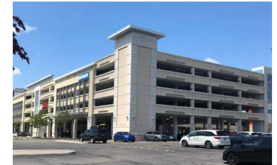
Fig 4.6.6 Aboveground Parking Garage, Bramalea City Centre
