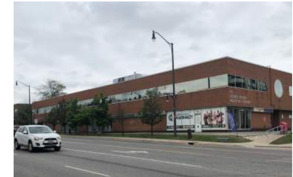
Fig 2.1.6 Office Building Along Centre Street
