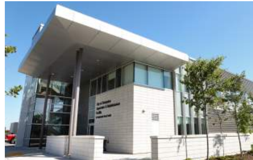
Fig 4.6.2 Brampton Apparatus and Maintenance Facility Entrance
