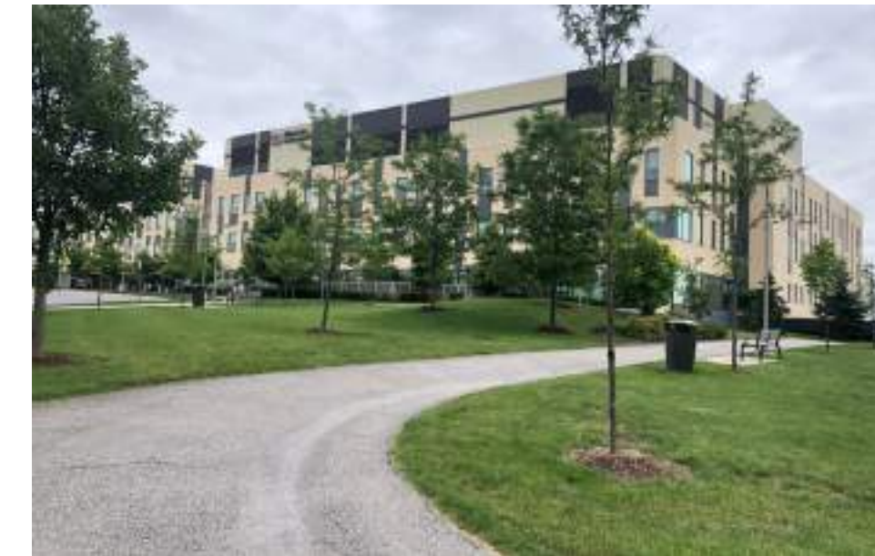
Fig 2.1.5 Peel Memorial Hospital
