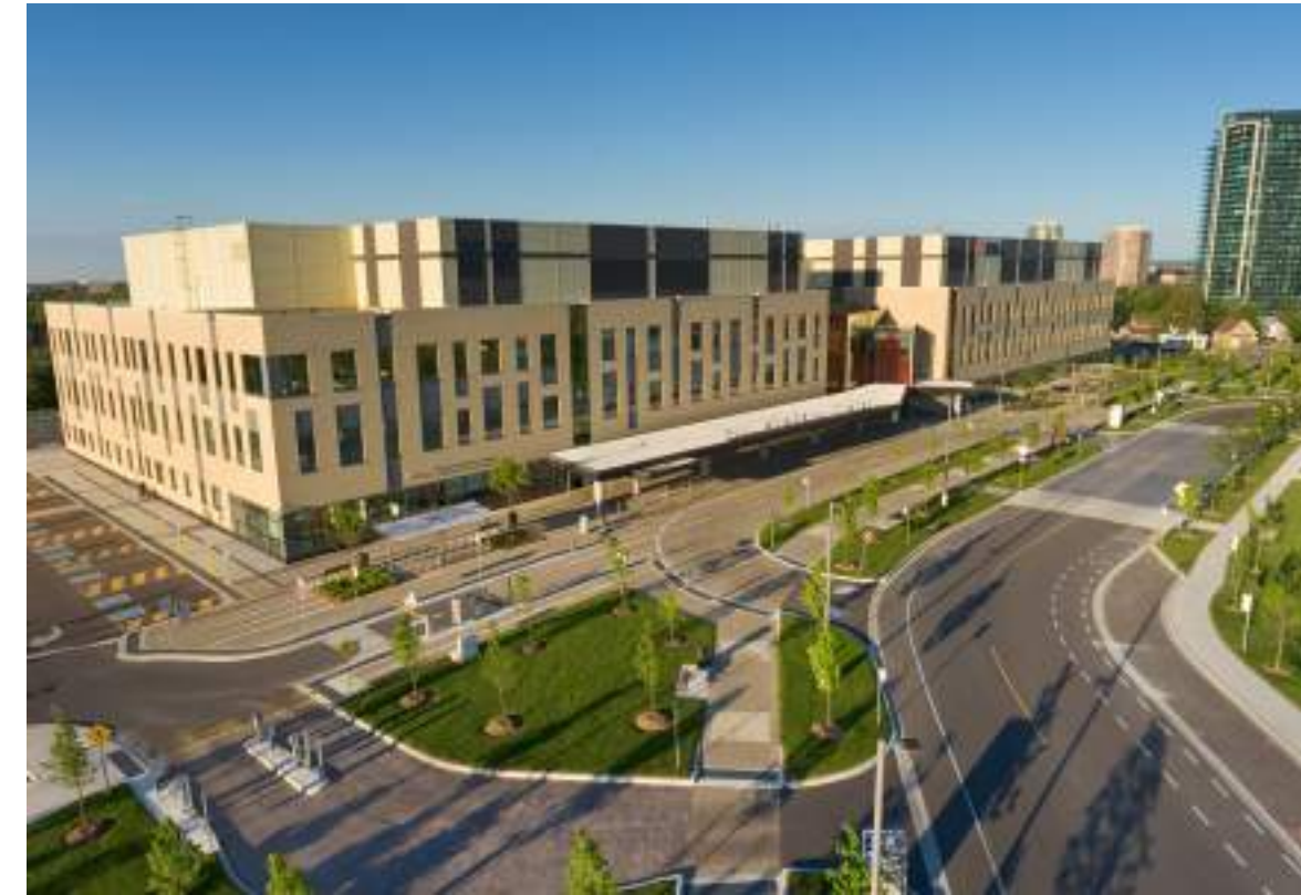
Fig 5.1.1 Peel Memorial Hospital
