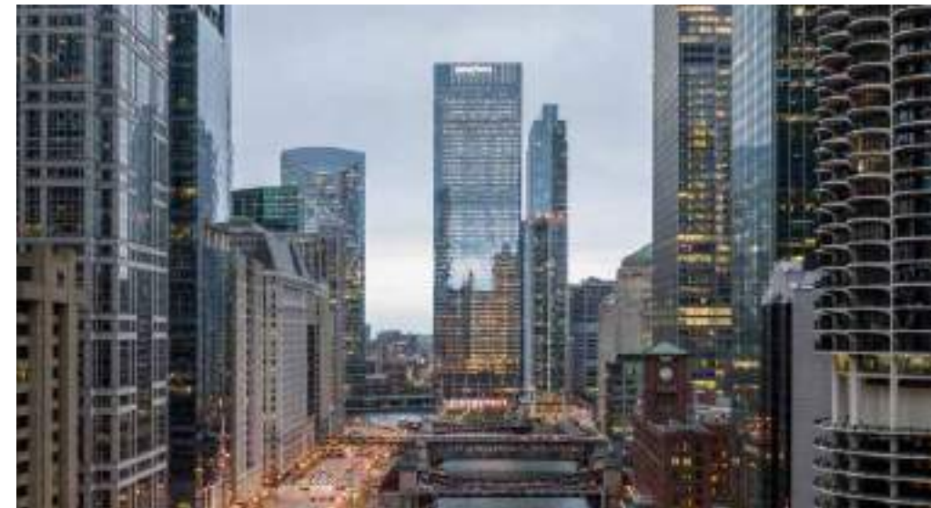
Fig 4.3.4 Salesforce Tower, Chicago, Goettsch Partners
