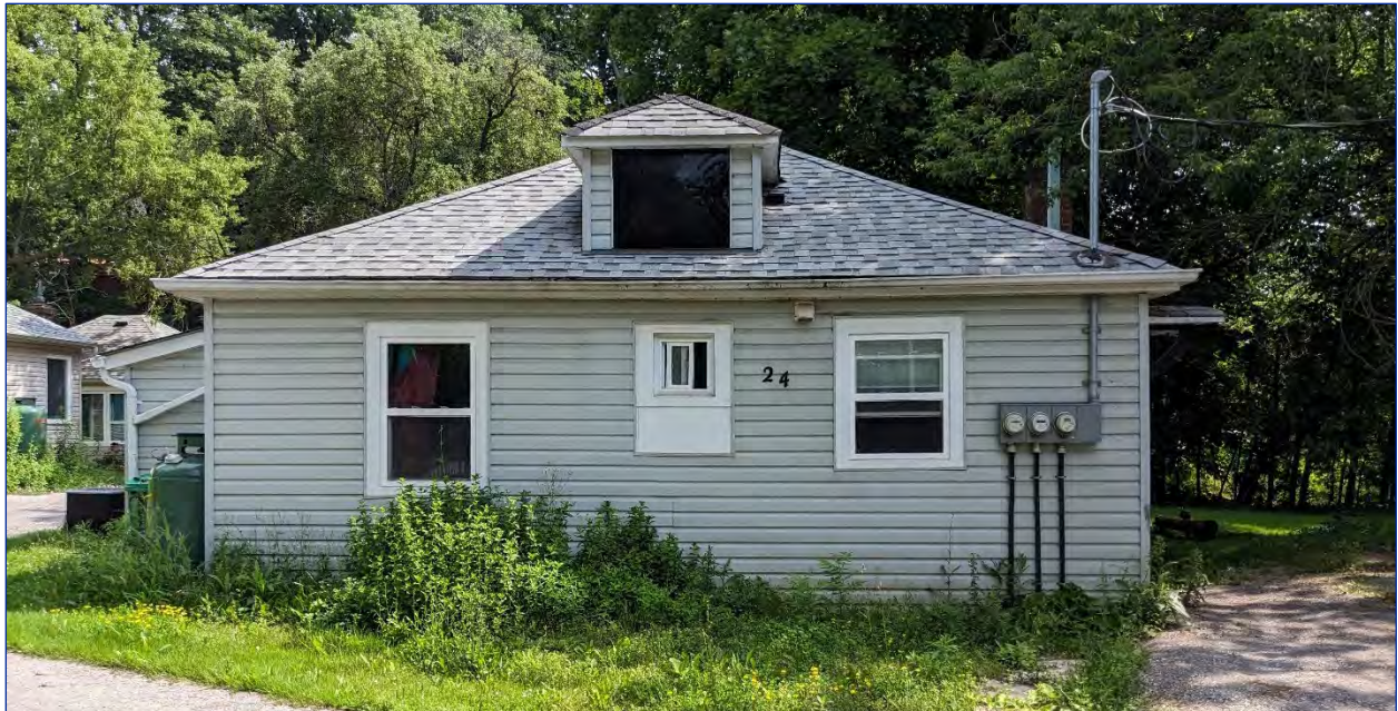
Photo 43: View of the south elevation
