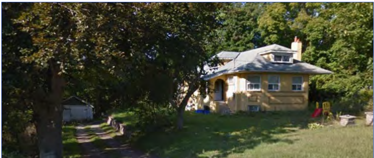
Photo 2: View of the house in 2014 86
