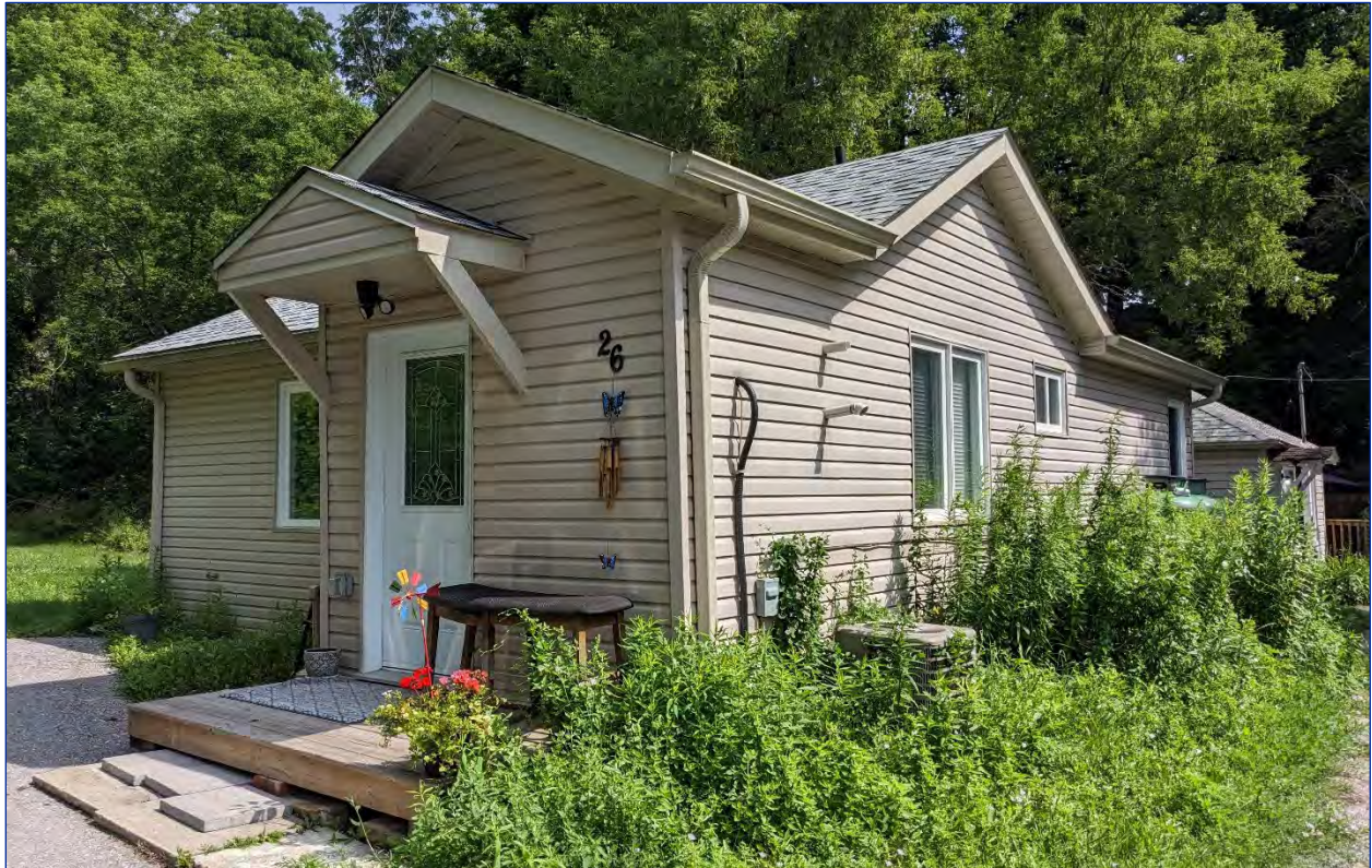
Photo 47: View of the south and east elevations
