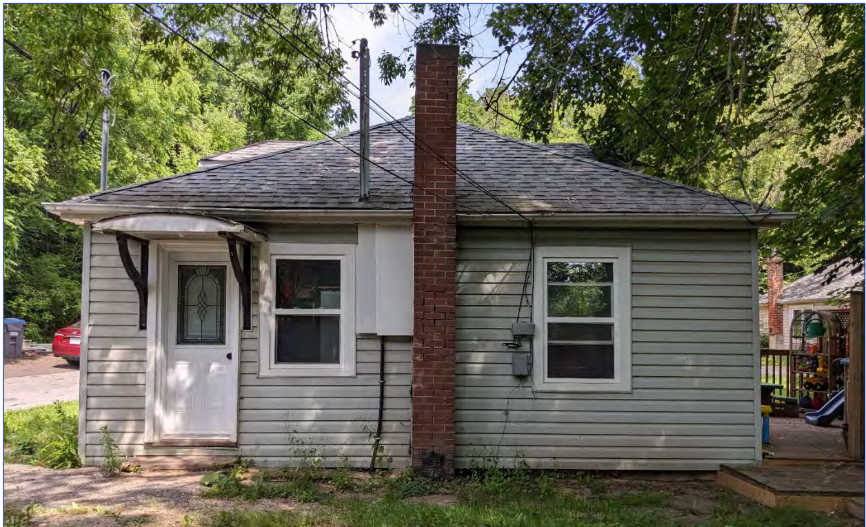
Photo 44: View of the east elevation
