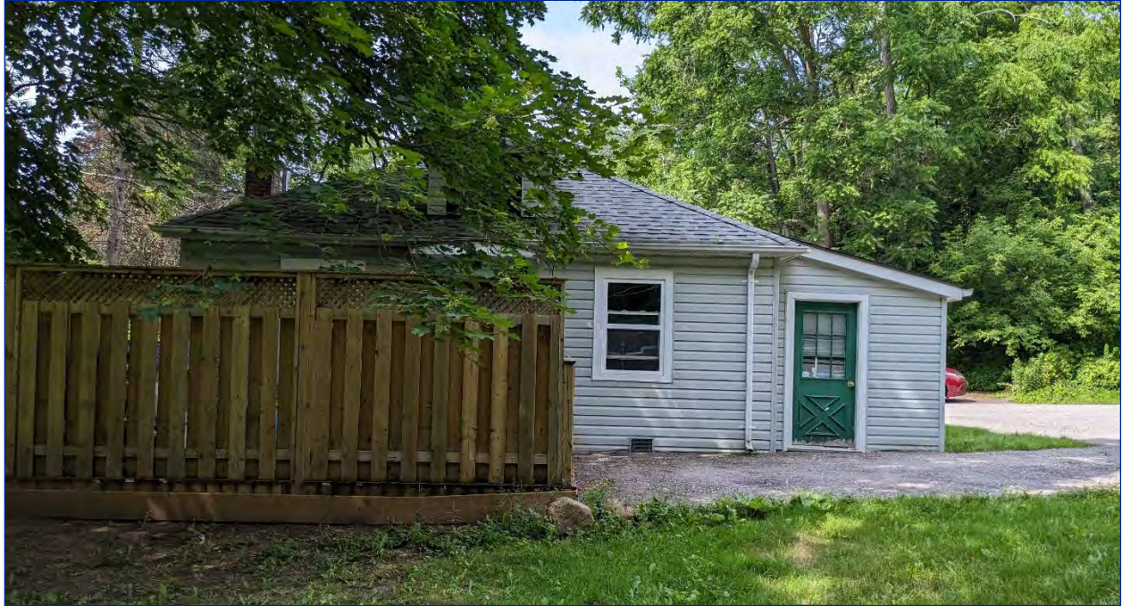
Photo 45: View of the north elevation
