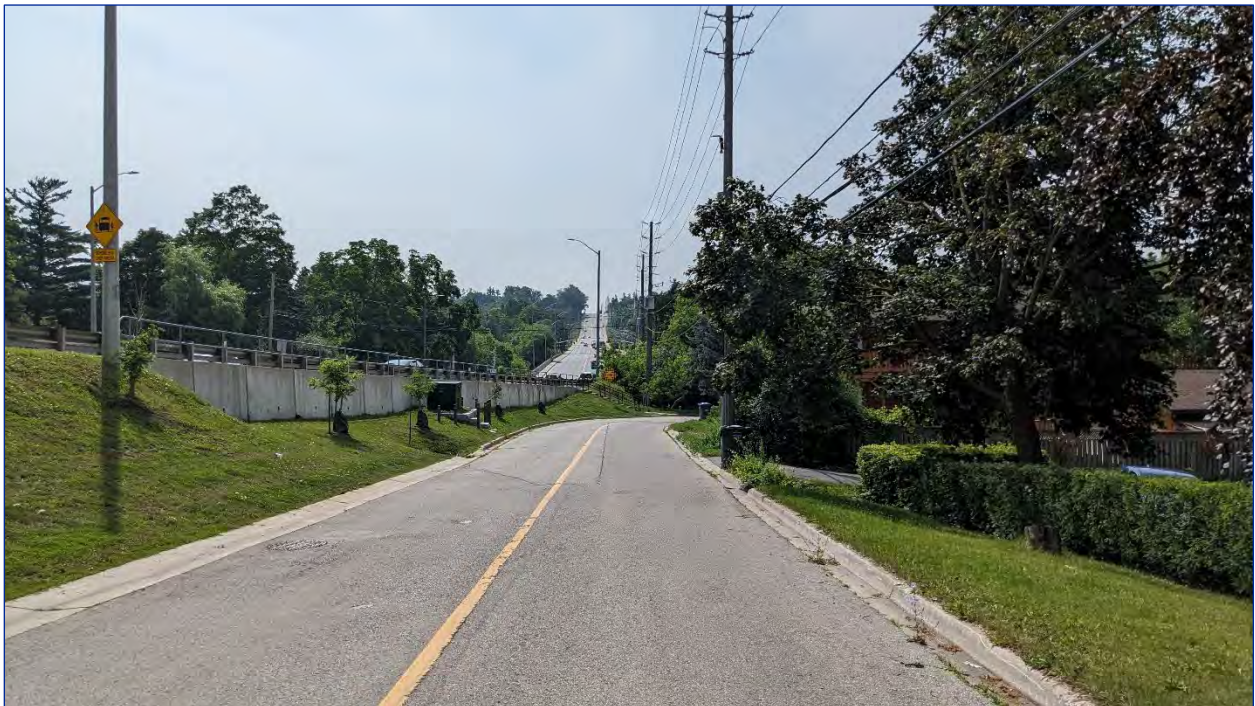
Photo 5: View southeast along River Road from the Property
