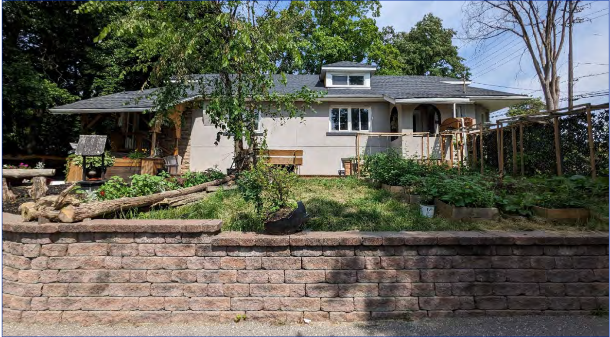
Photo 17: View northwest of the east elevation
