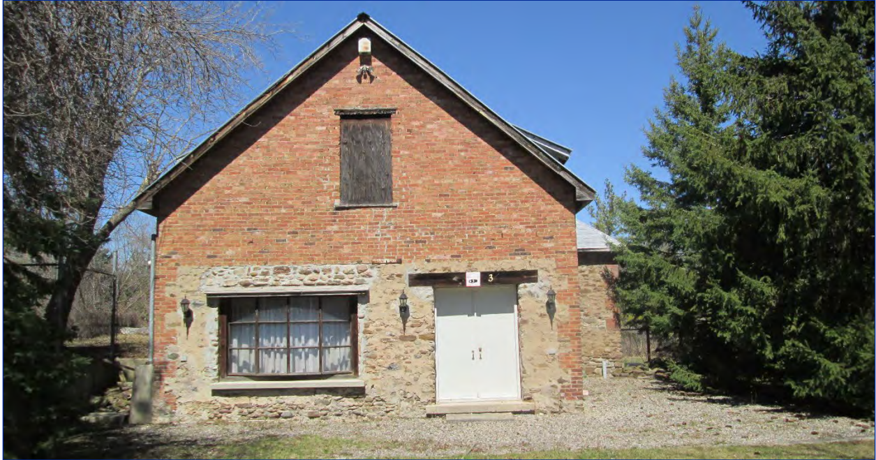
Photo 13: Photograph of the McMurchy Powerhouse 99
