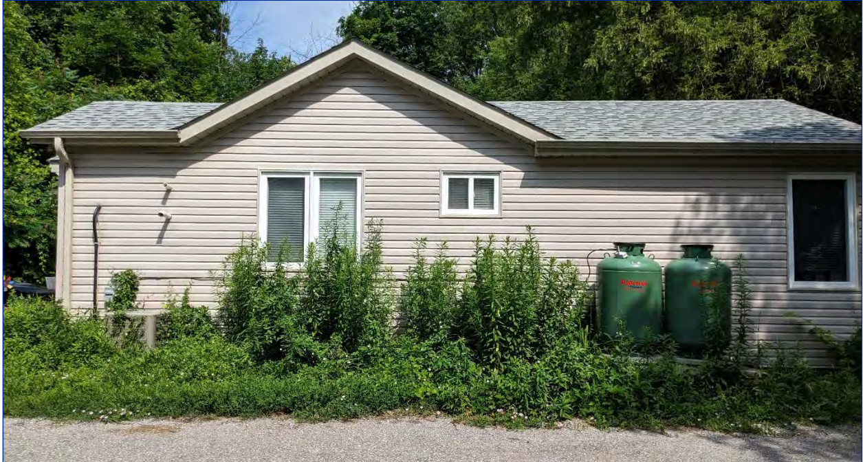
Photo 48: View of the east elevation
