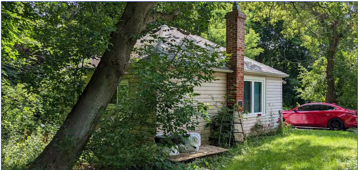
Photo 52: View of the north and west elevations
