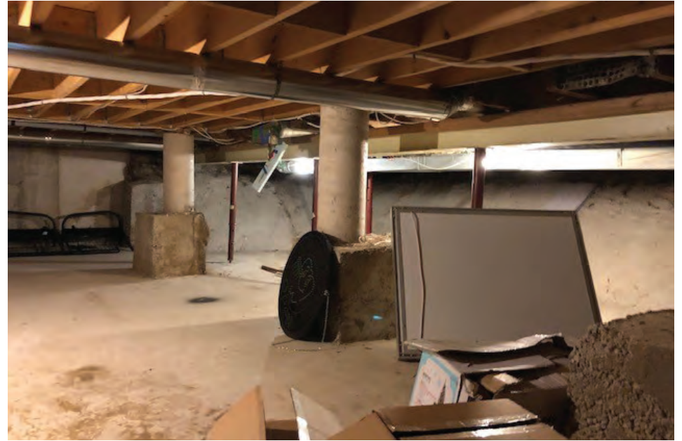
Crawl space 1st and 2nd addition Source: ATA Architects Inc. 2021
