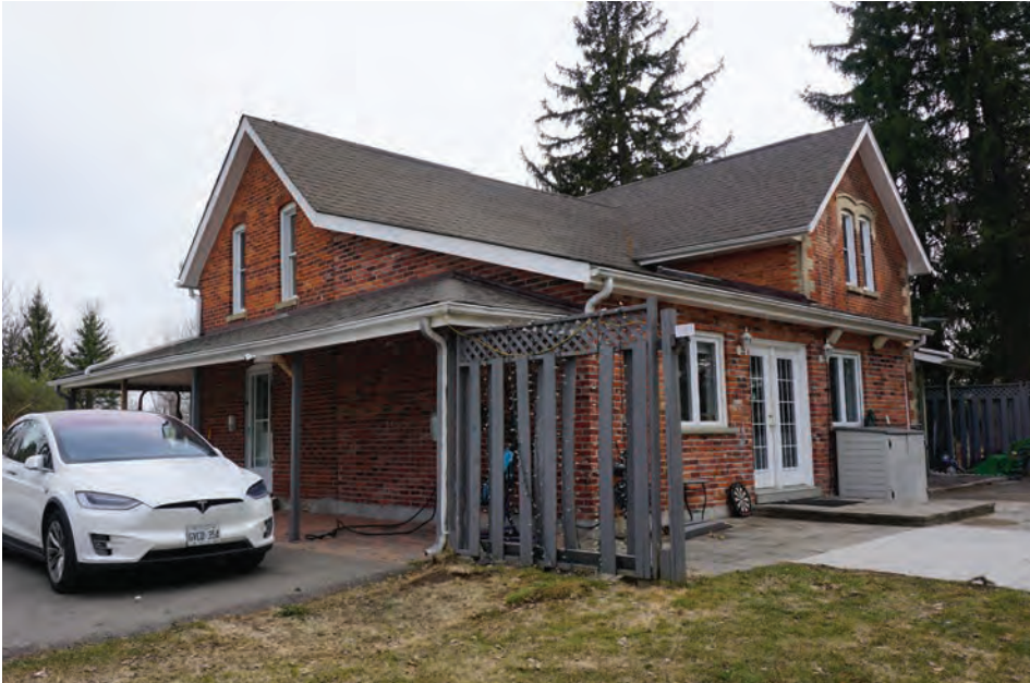
View towards the north corner of facade. The connection between the 1st and 2nd addition are visible to the left. The gable end of the original farmhouse is at the right.
