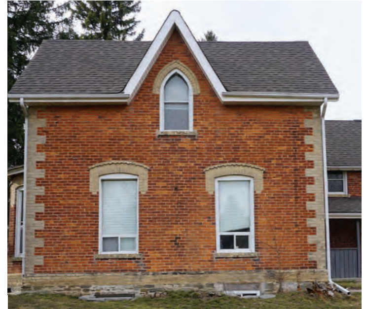
Southeast facade, original house
