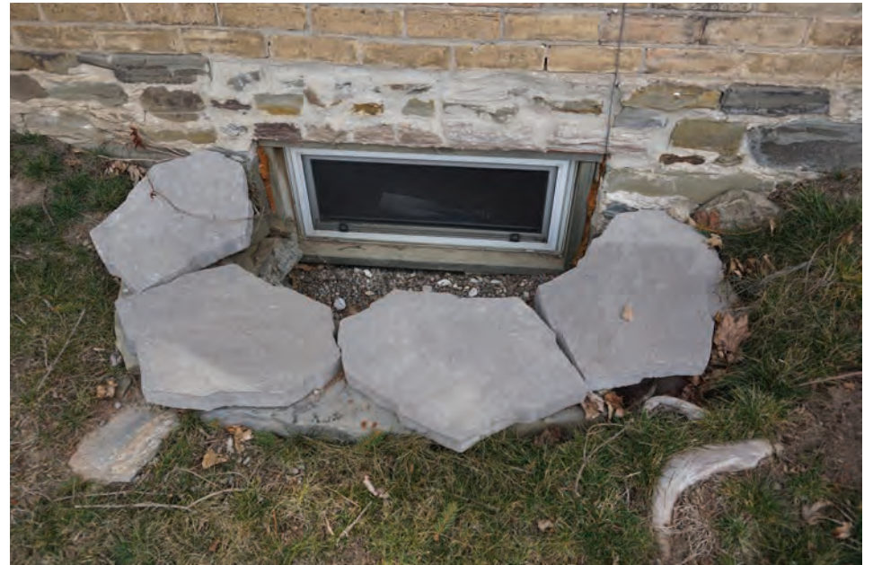
Pressure treated wood framing / drystone light well.
