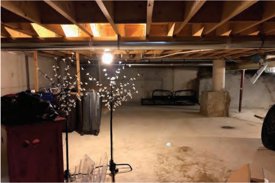
Crawl space 2nd addition Source: ATA Architects Inc. 2021
