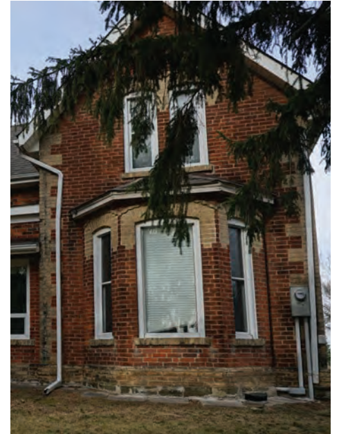
Detail view of Front Facade gable end.
