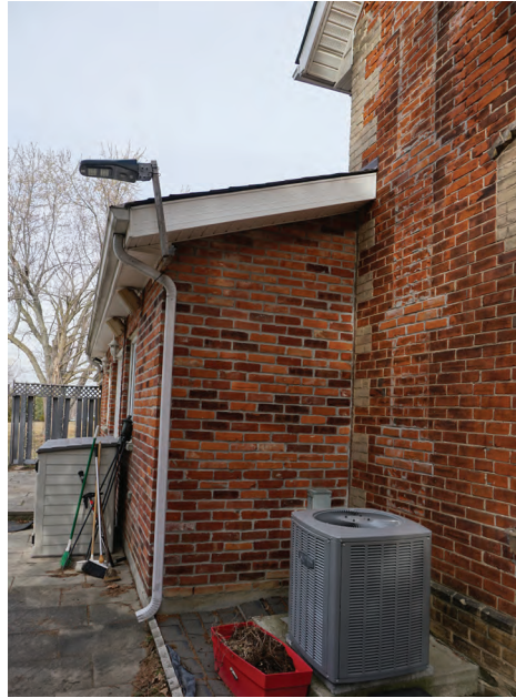
Latest addition, masonry repair visible on the brick gable.
