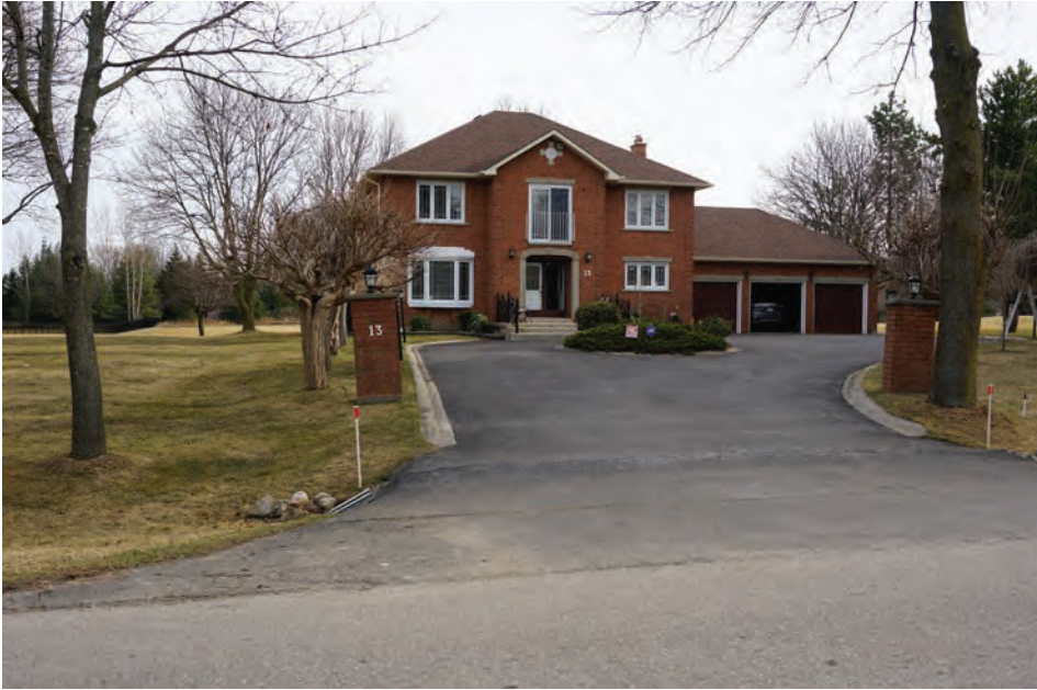
Exterior View of 13 Rosegarden Drive.
