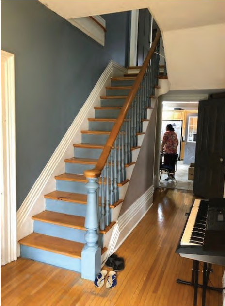
Centre original staircase
