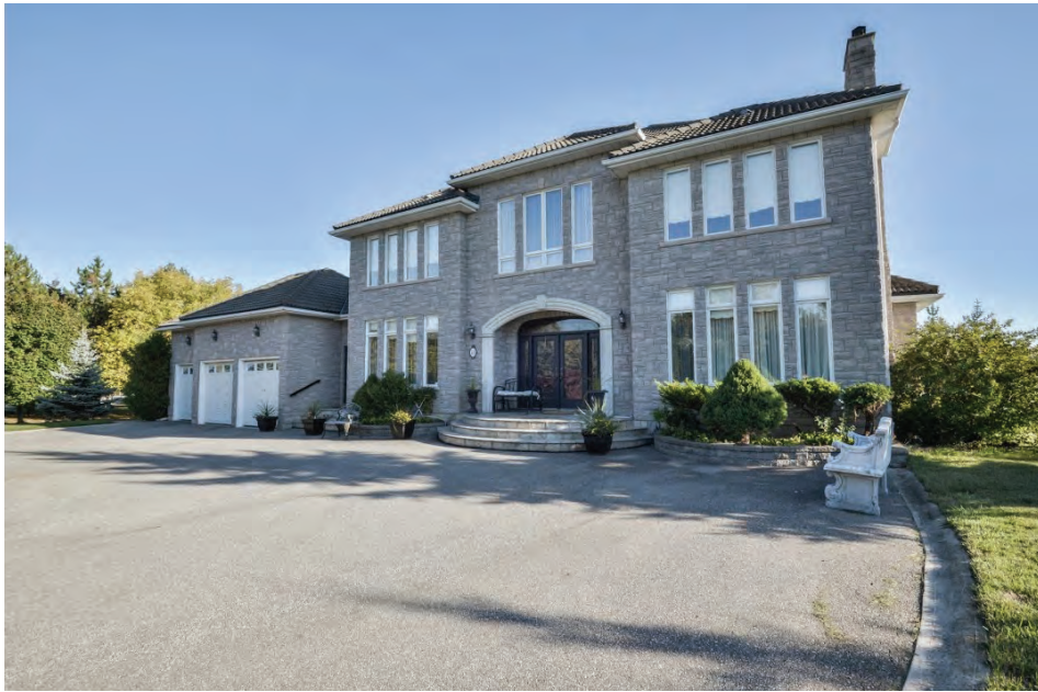
Exterior View of 11 Rosegarden Drive
