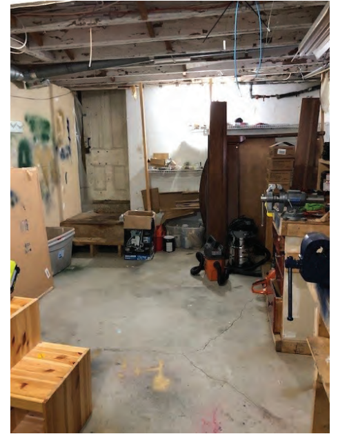
Basement, original house Source: ATA Architects Inc. 2021
