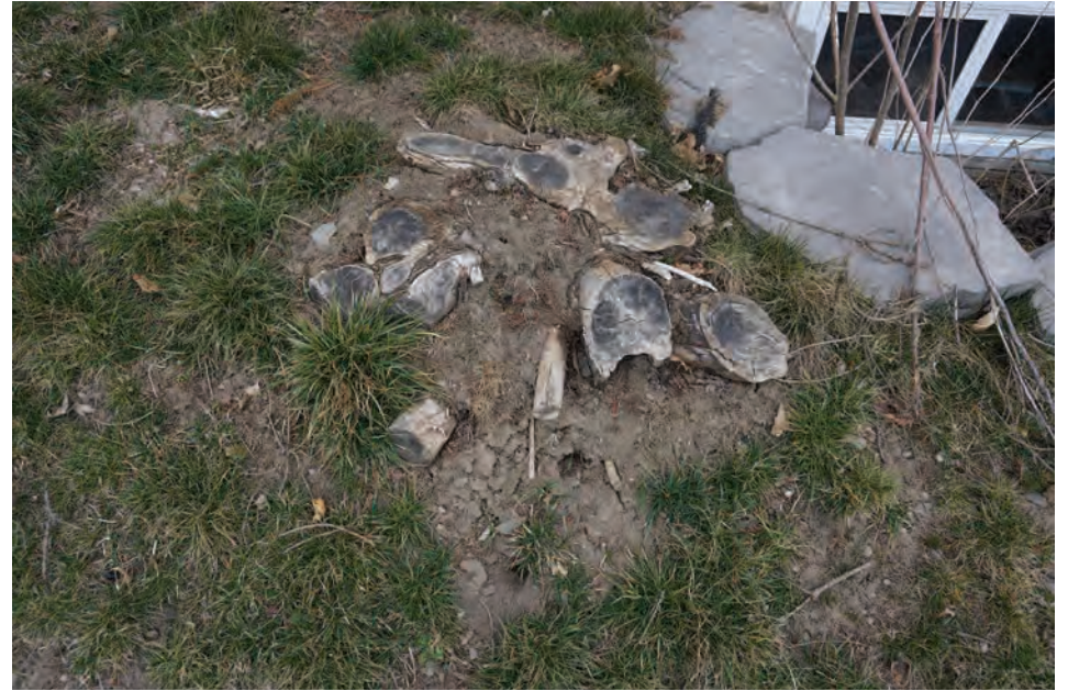
Trees located near the foundations have been removed.
