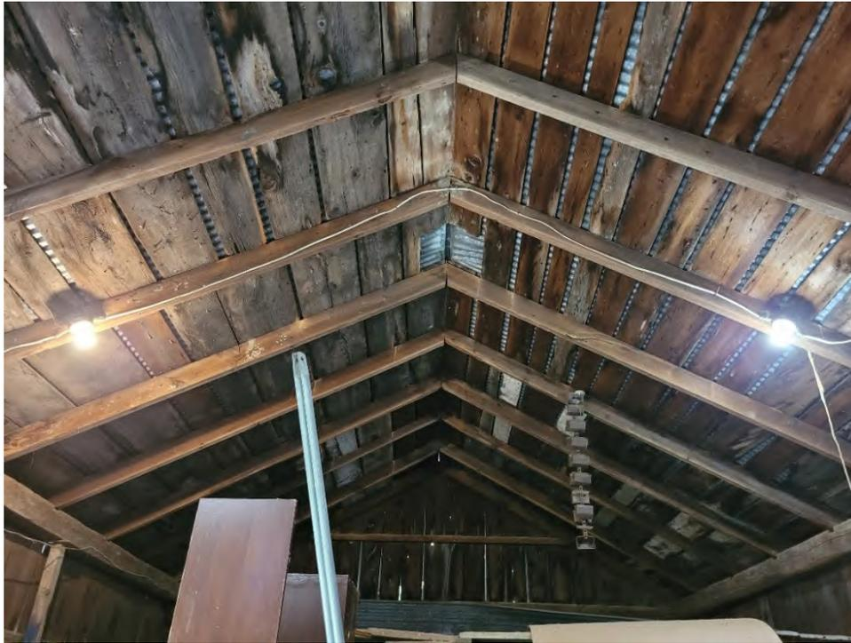
**Figure 68: Dimensional cut rafters**
