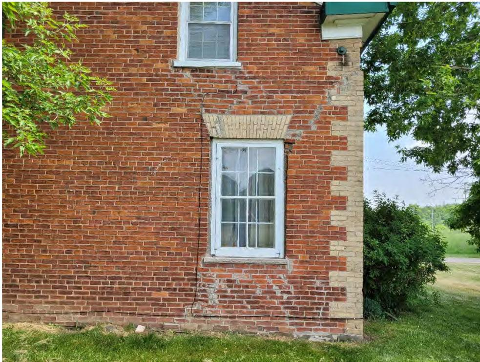
**Figure 71: Evidence of cracks radiating from the first level window on the north end wall.**
