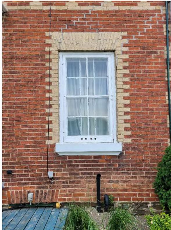
**Figure 24: Six-over-six window with wood storm, buff gauged or rubbed brick voussoirs and quoins, and a lug sill with aluminum covering**
