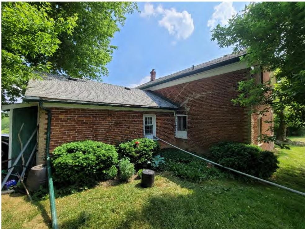
**Figure 72: Evidence of cracks on the east facade of the main block.**
