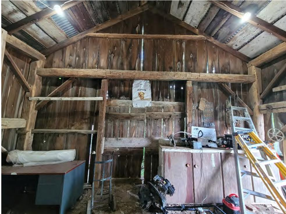
Figure 67: Interior of the driveshed with drop tie-beam, hand-hewn posts and plates and east doorway, facing east
