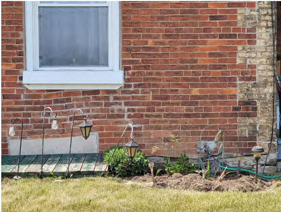
**Figure 73: Settlement and movement of load-bearing brick masonry on south end wall**
