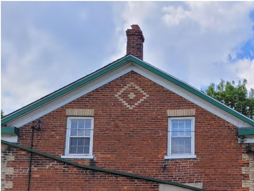
**Figure 22: Cornice returns and single-stack brick chimney**
