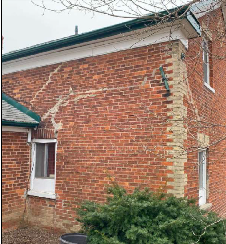
Photograph 8: Typical condition of exterior walls
