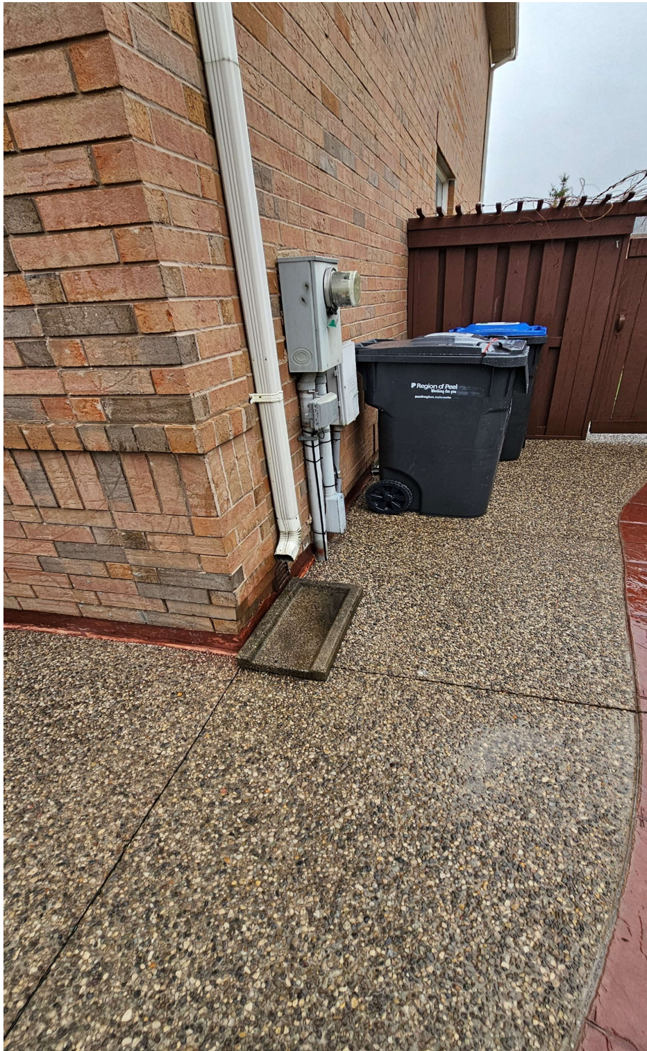
Figure 10 Front Yard Eave and Concrete Splash Pad Adjacent to the Landscaped Area
