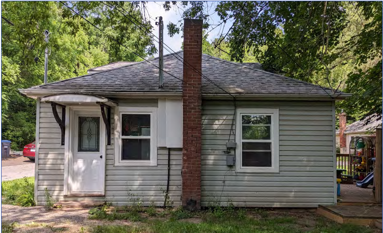
Photo 44: View of the east elevation
