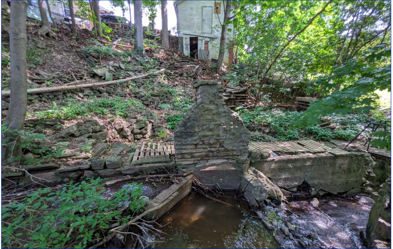
Photo 40: View north across the creek to the shed
