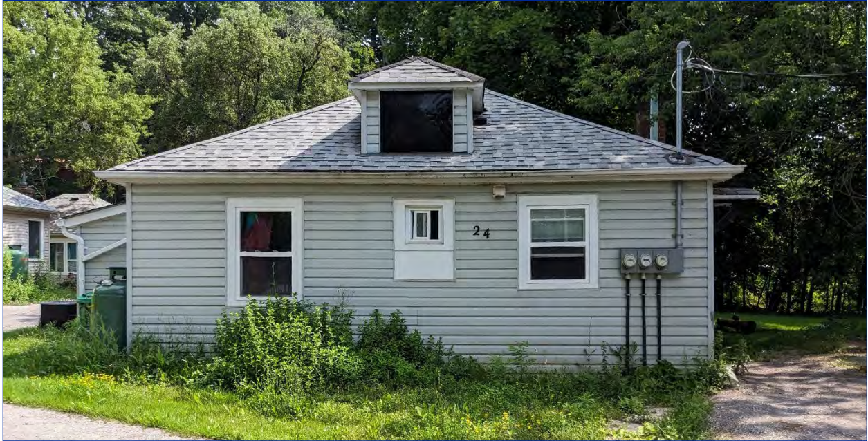
Photo 43: View of the south elevation
