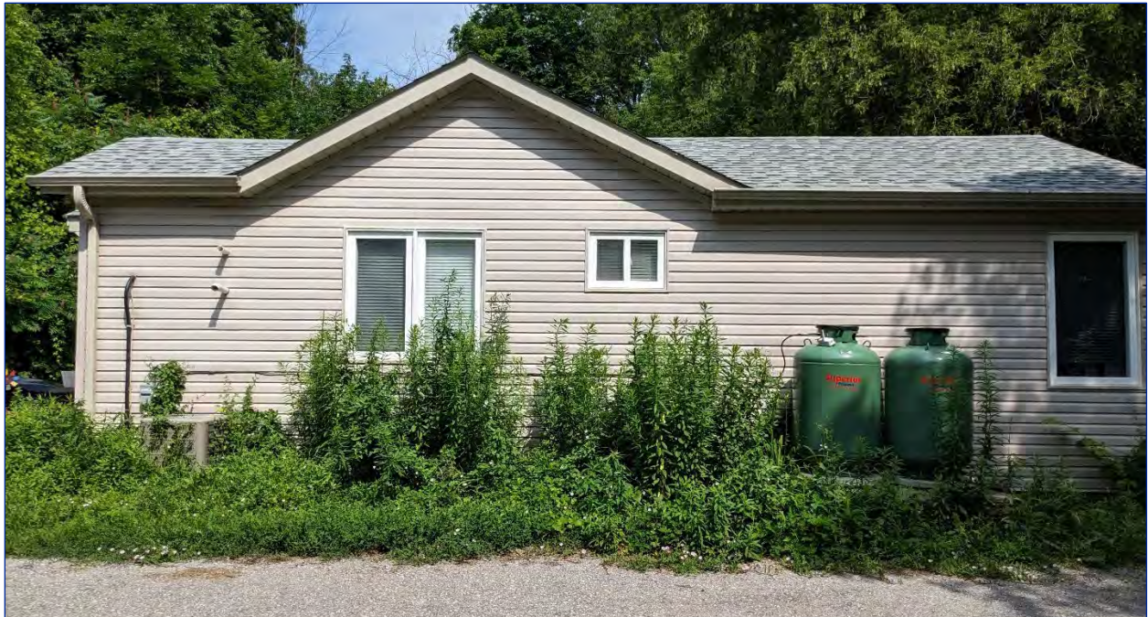
Photo 48: View of the east elevation
