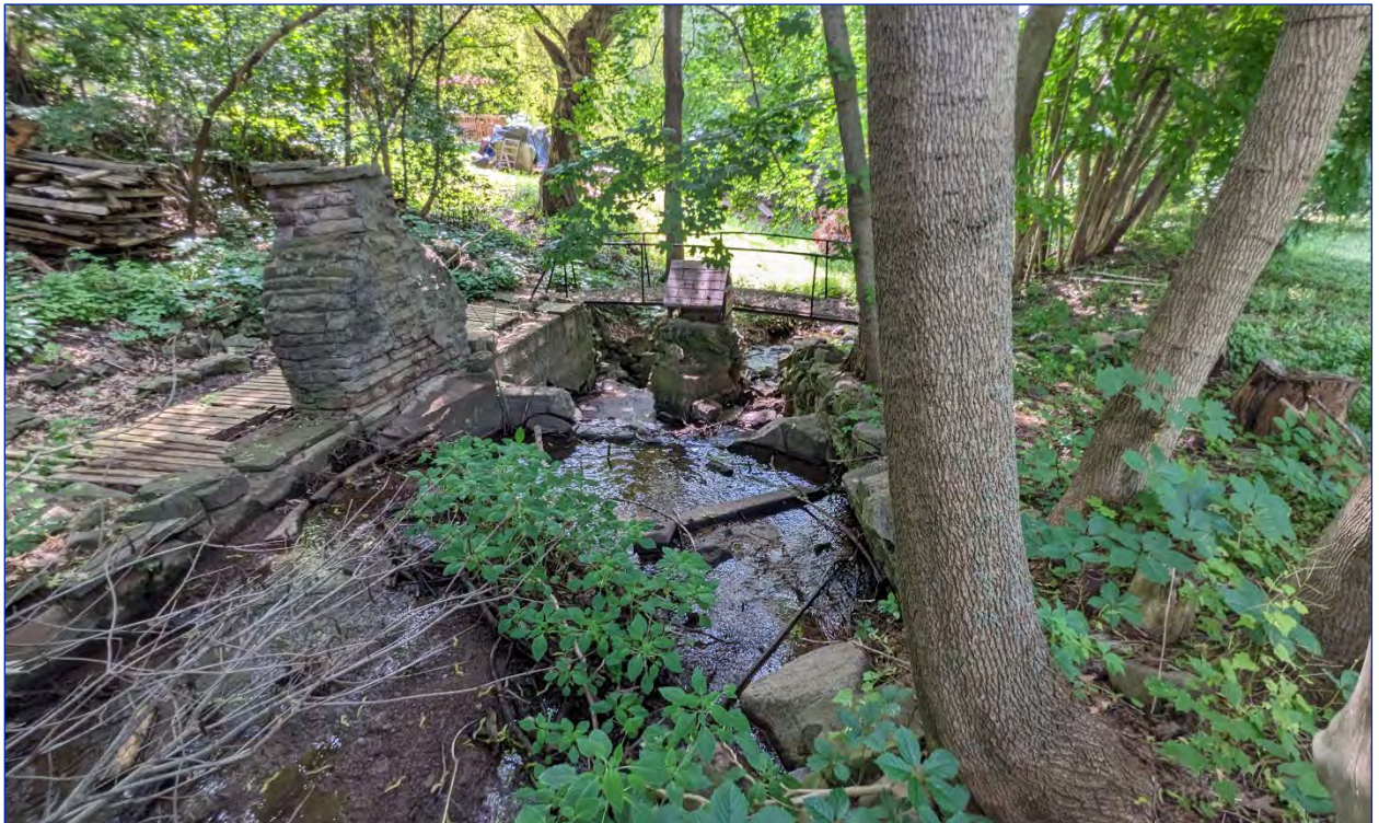
Photo 41: View east of the bridge over Duke Creek from the main house to the cottages
