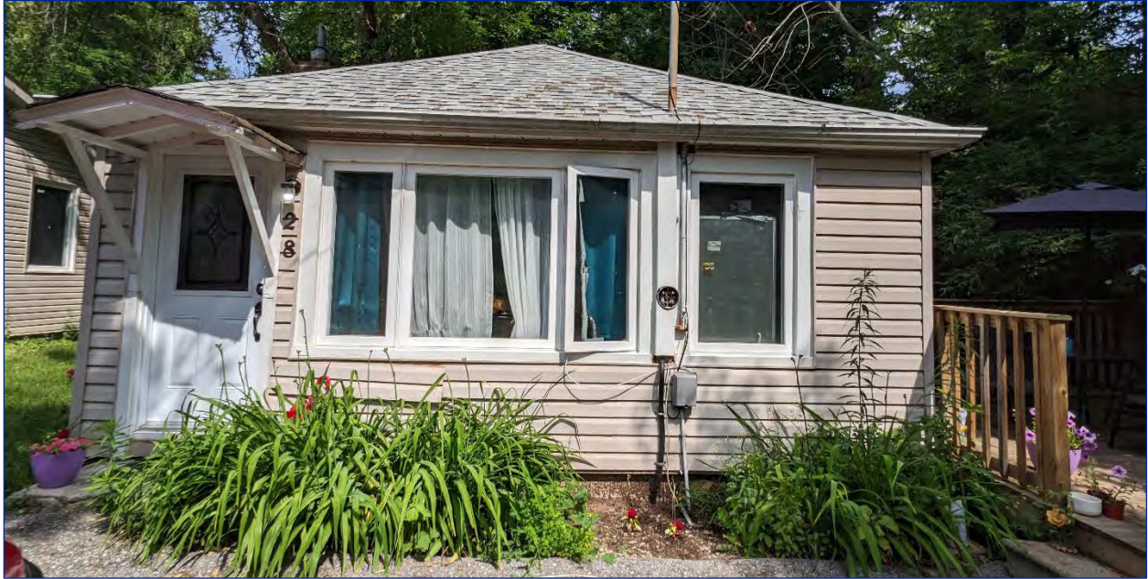
Photo 51: View of the east elevation
