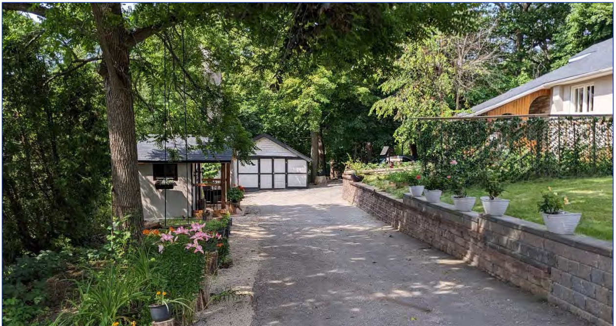
Photo 39: View southwest of additional accessory buildings
