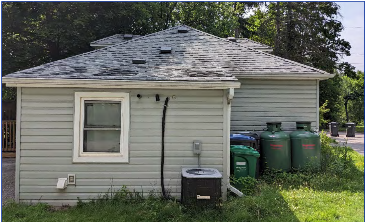
Photo 46: View of the west elevation
