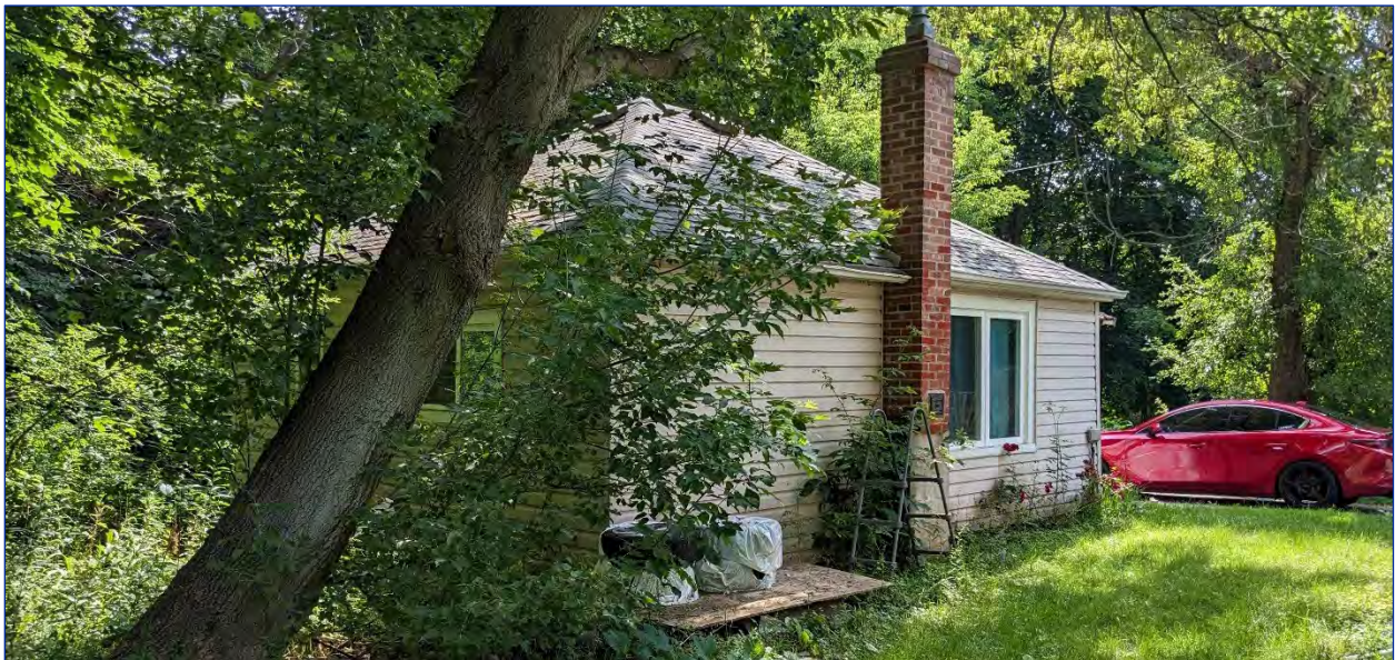
Photo 52: View of the north and west elevations
