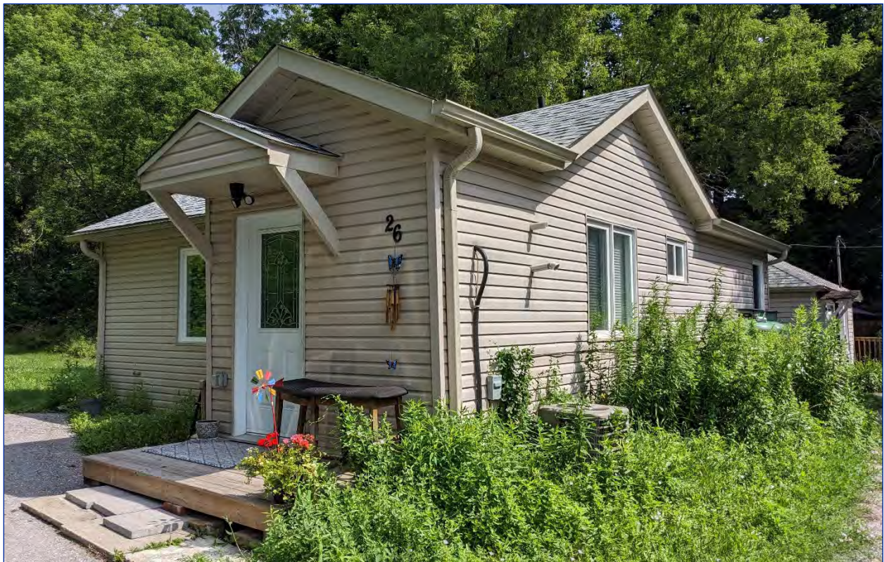
Photo 47: View of the south and east elevations
