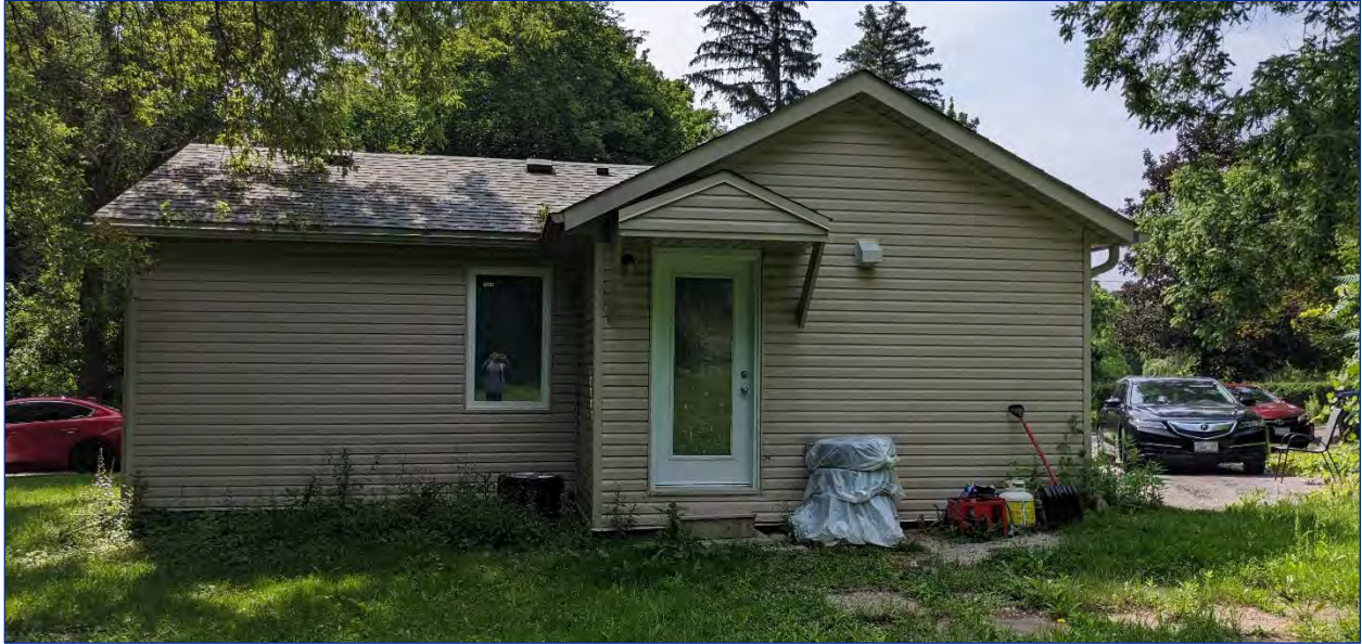
Photo 50: View of the west elevation
