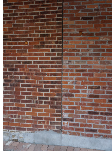
Junction visible between the 1st and 2nd additions.
