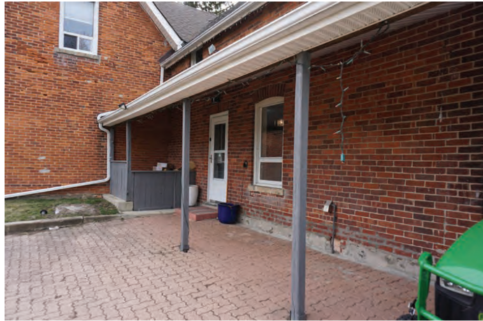
Side door entry to second addition (porch likely added).
