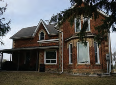
445 Hazelhurst Road. Source: ATA Architects Inc. (2023)
