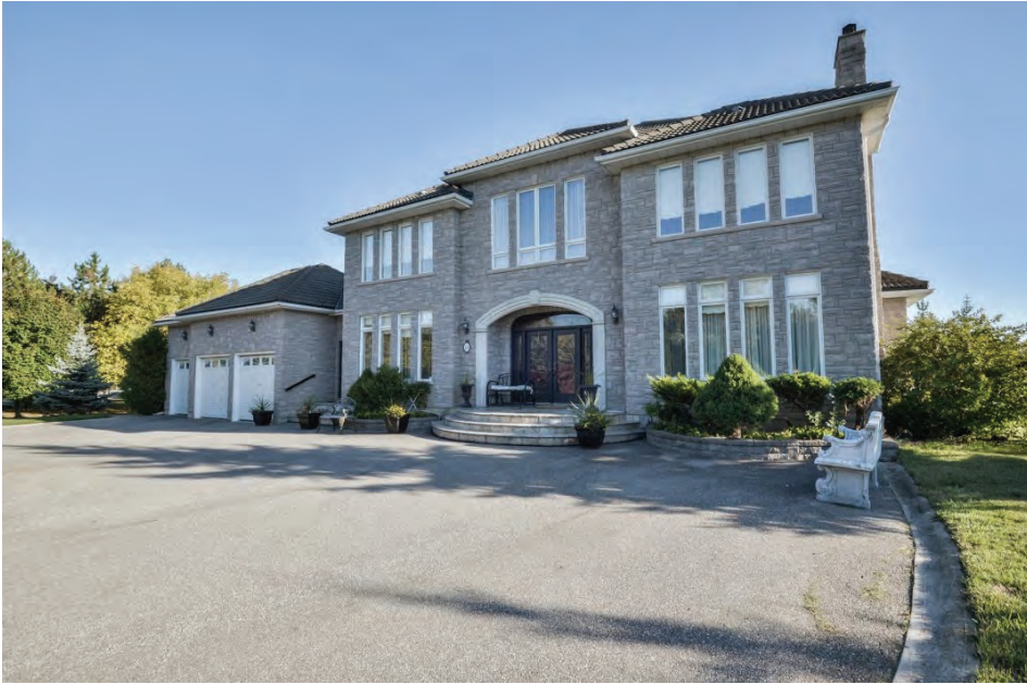
Exterior View of 11 Rosegarden Drive
