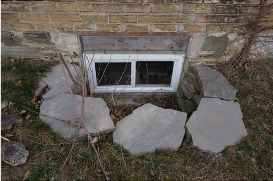
New basement window and wood lintel.
