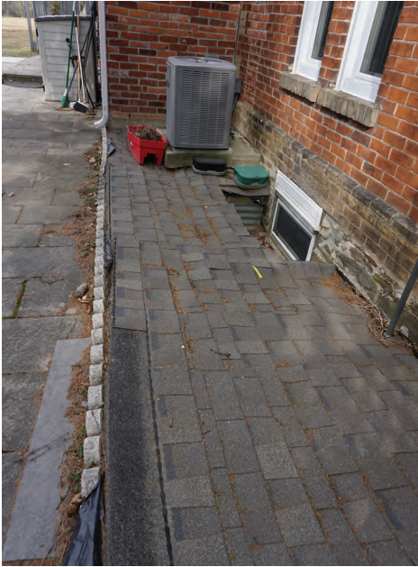
Asphalt single apron and precast curb.
