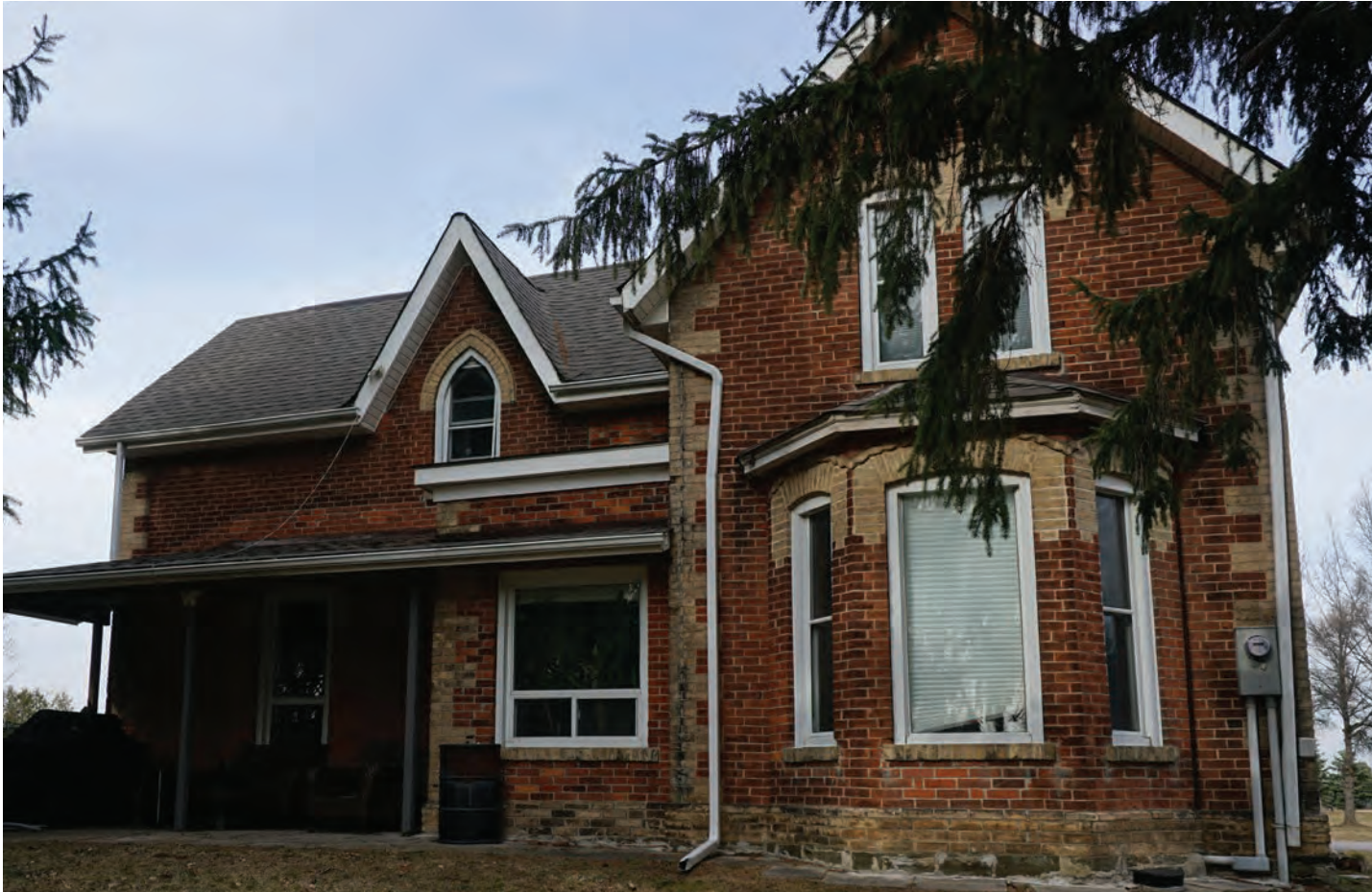
Southwest facade exterior; the original farmhouse Source: ATA, 2021
