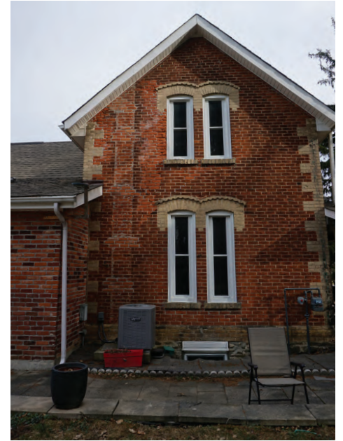
Gable end to porch wing.
