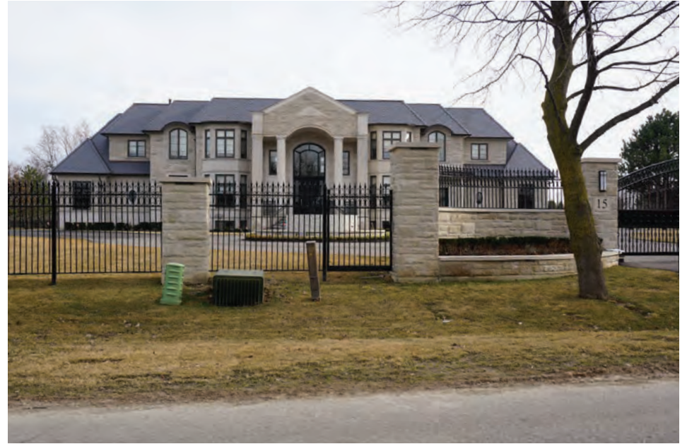
Exterior View of 15 Rosegarden.
