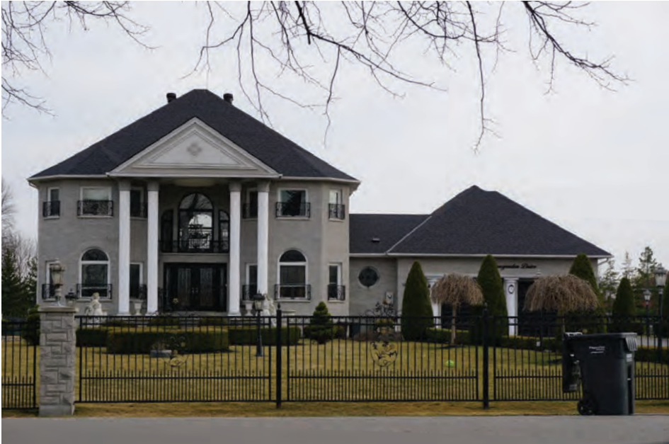
Exterior View of 9 Rosegarden Drive.
