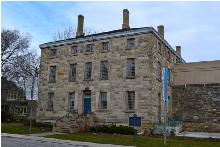
Building 9 (The Old Brampton jail)
