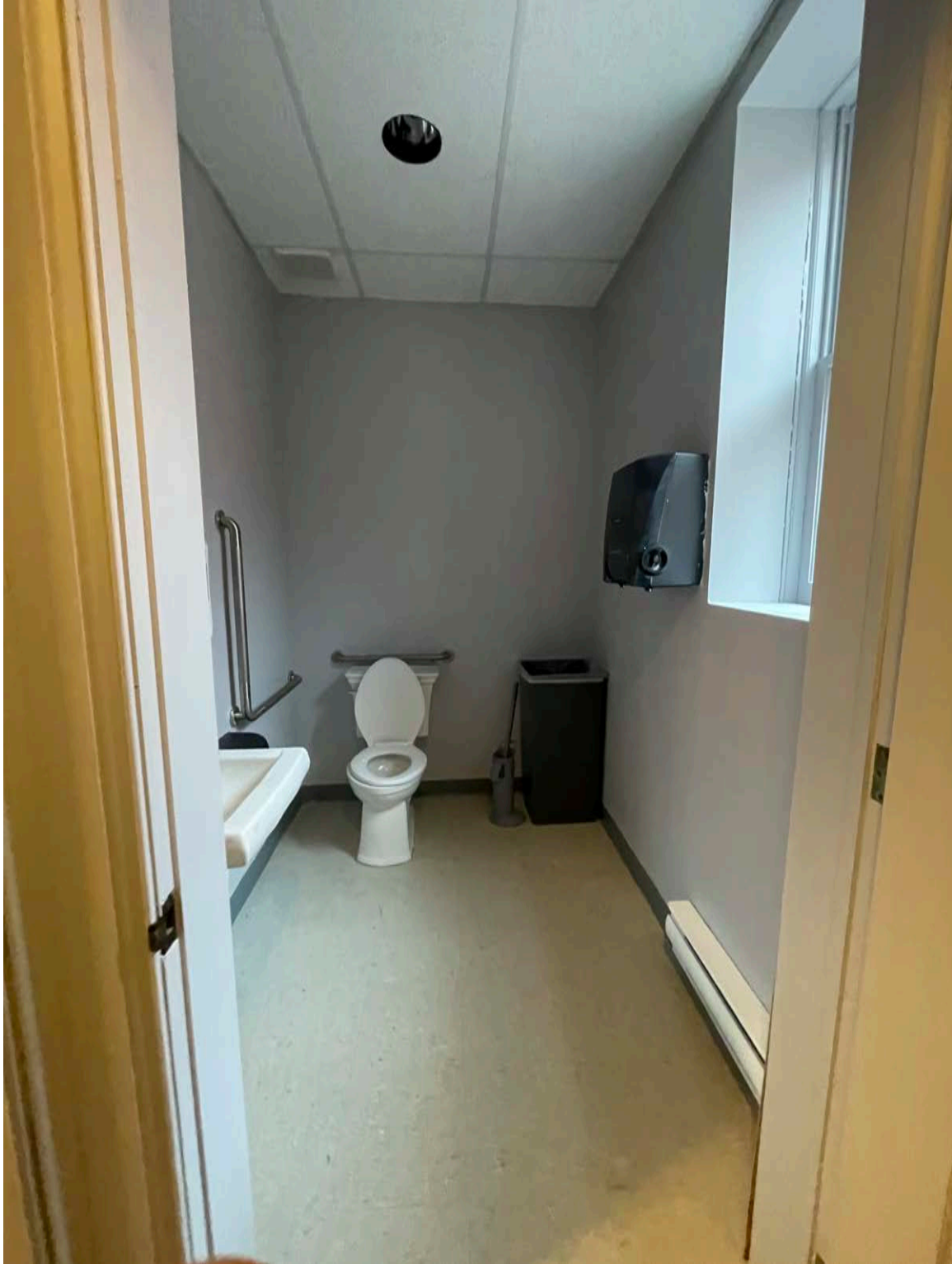
WASHROOM – existing two-piece washroom on the lower level – no original finishes or features - modern fixtures, drywall, vinyl flooring & acoustic tile ceiling – door casing on outer side may be original
