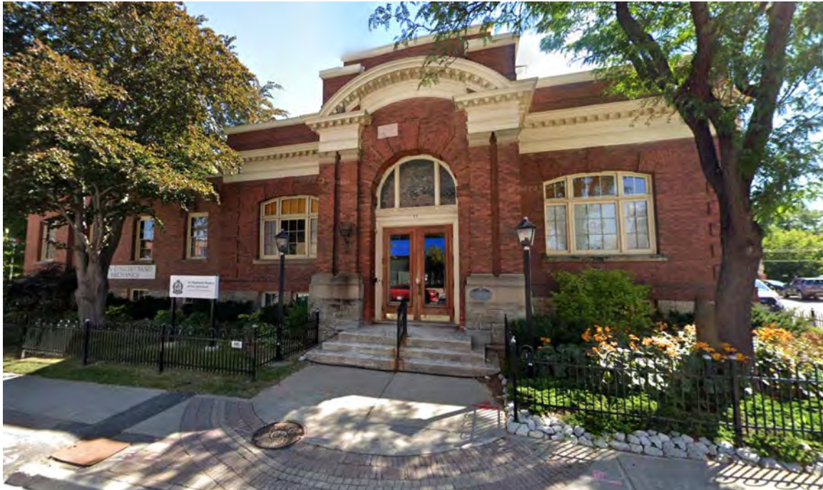
FRONT ENTRANCE ON QUEEN STREET – accessibility upgrades are proposed for the main entrance to the building
