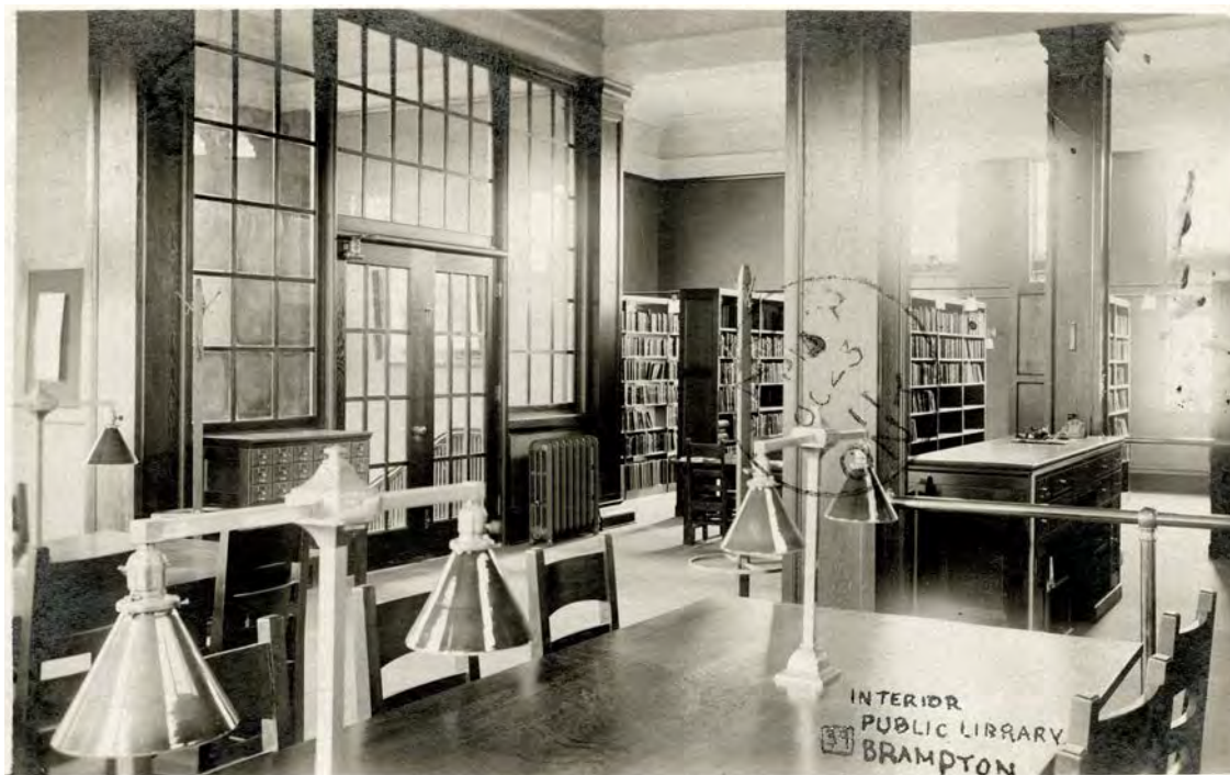
HISTORIC PHOTO – INTERIOR (1911): the original interior of the Carnegie Library – the glazed partition wall remains
