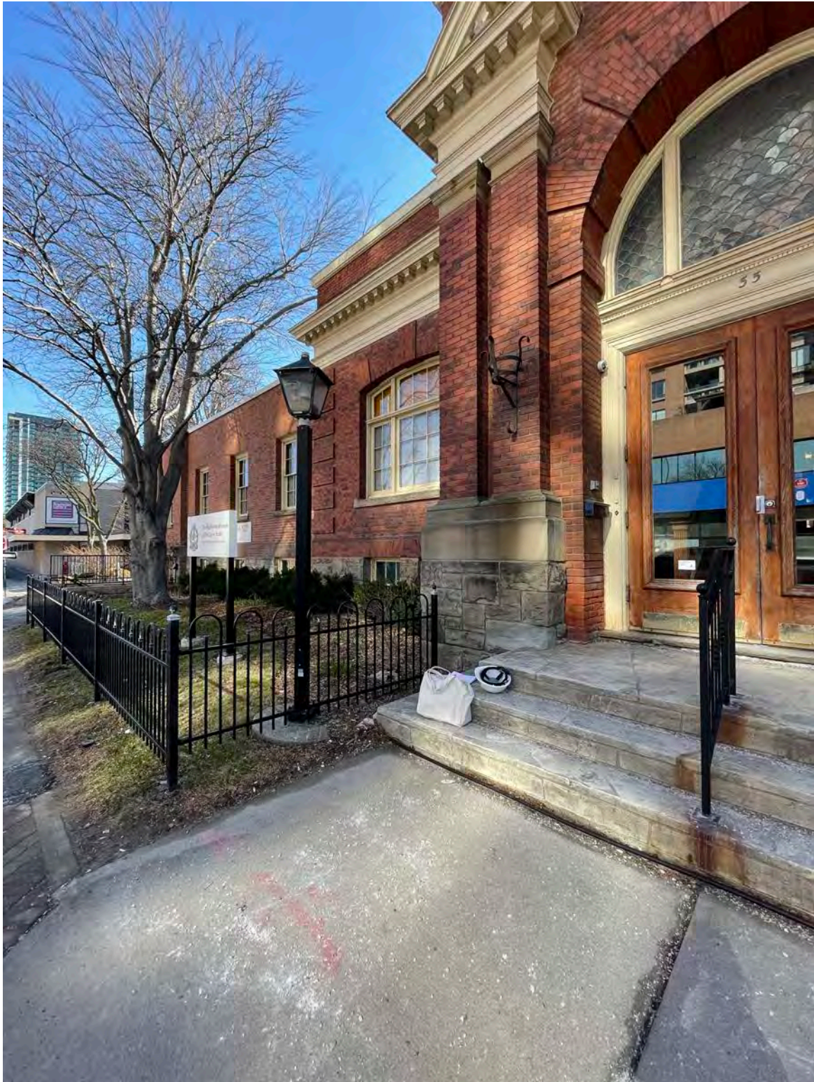
EXTERIOR – MAIN ENTRANCE: stone steps, paved path & sidewalk, landscaped area enclosed by a wrought iron fence
