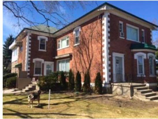
Figure 6: Southwest corner views of Learment-C. Armstrong House in 2016 (AREA, HIA, 2016, figs. 16)
