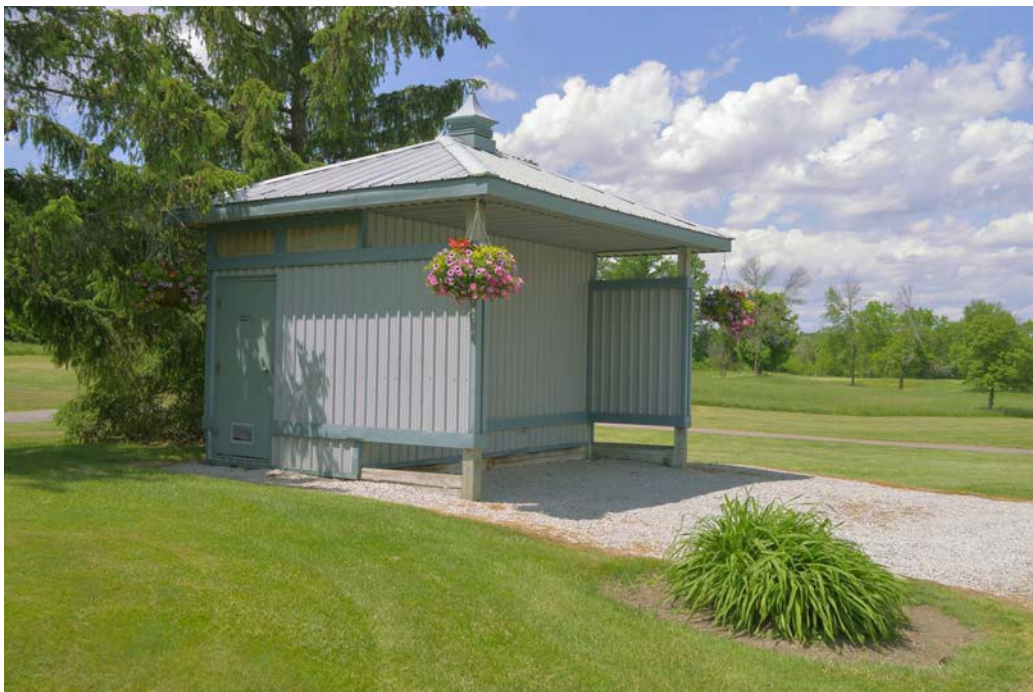
Fig. 26 The only structure where the golf course subdivision is proposed is a washroom.
