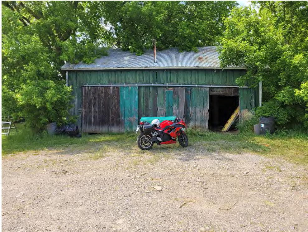
Figure 64: South façade of the driveshed with large slight doors, facing north.
