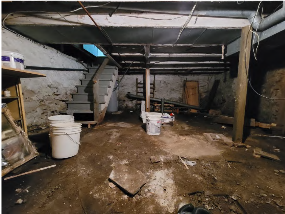
Figure 52: Basement with straight wood stairs, facing east
