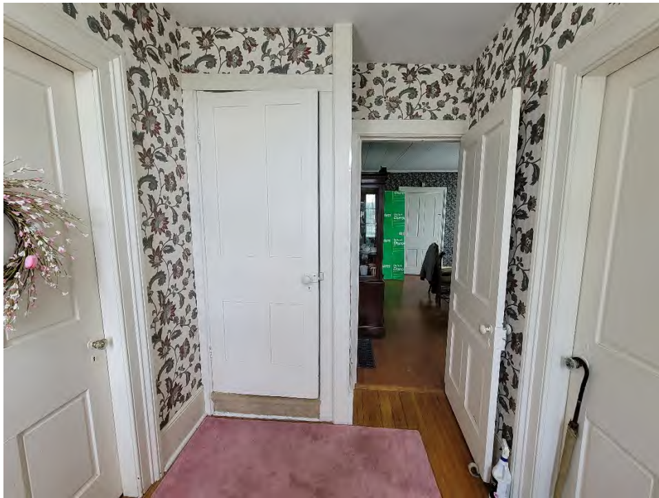
Figure 26: Vestibule with living room (left), stairs to second level (centre-left), dining room (centre-right), and office (right), facing west
