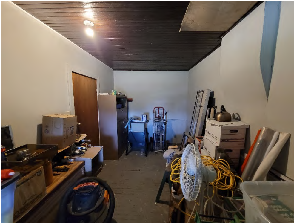
Figure 61: East half of the rear wing, facing north
