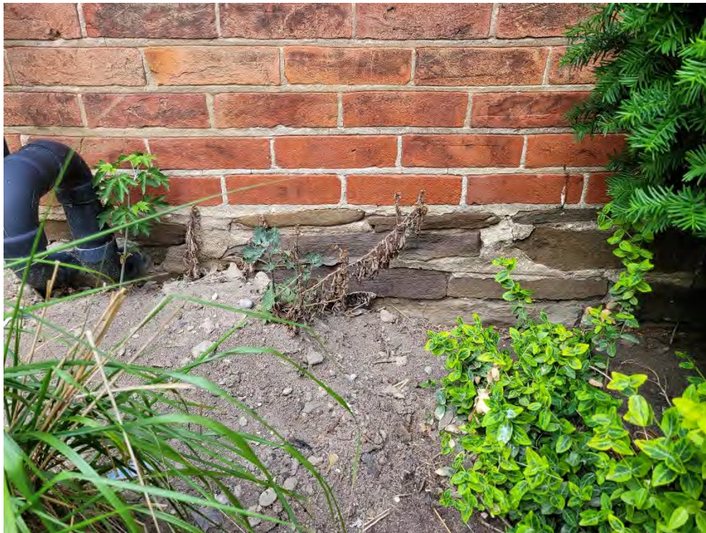
Figure 20: Coursed split fieldstone foundation
