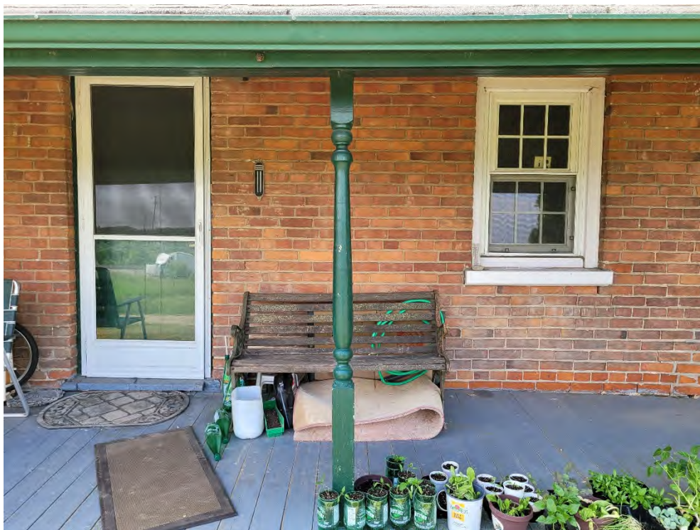
Figure 58: Doorway, window and turned wood post supporting verandah's roof, facing north
