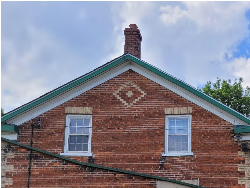
Figure 22: Cornice returns and single-stack brick chimney
