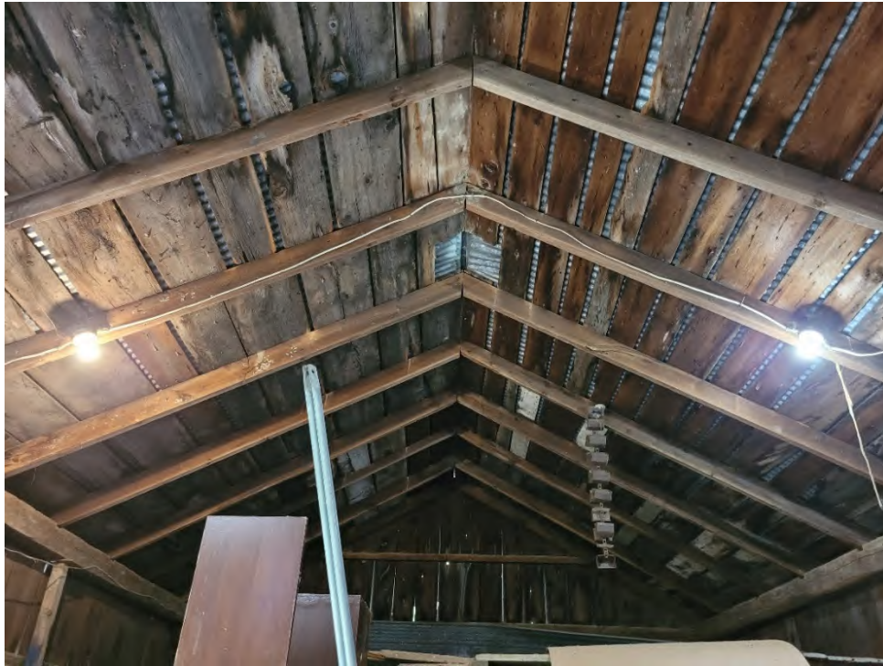
Figure 68: Dimensional cut rafters
