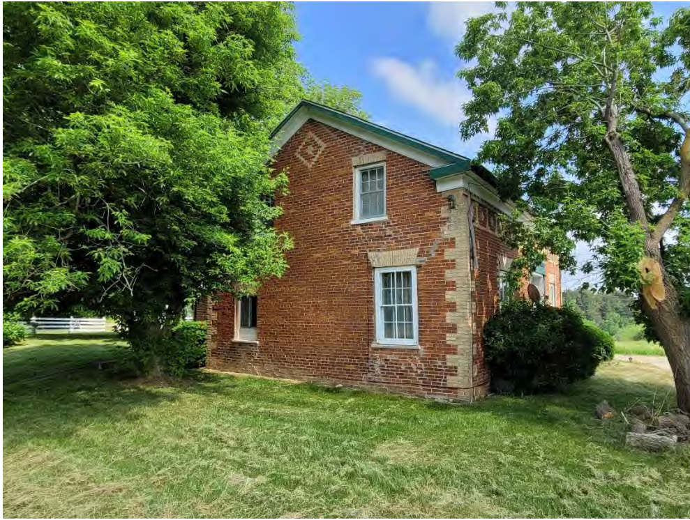
Figure 18: North end wall of the main block
