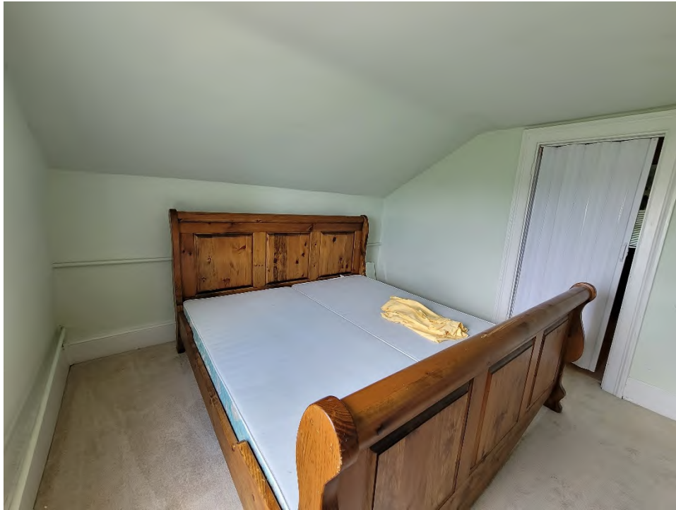
Figure 49: Southwest room with tie rod along south and west walls, facing northwest
