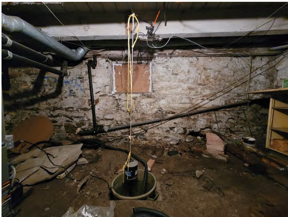
Figure 55: Basement with coursed fieldstone foundation, facing west
