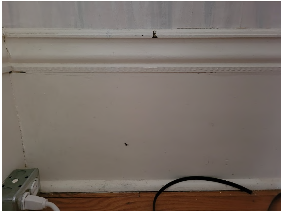
Figure 30: High moulded baseboards within living room
