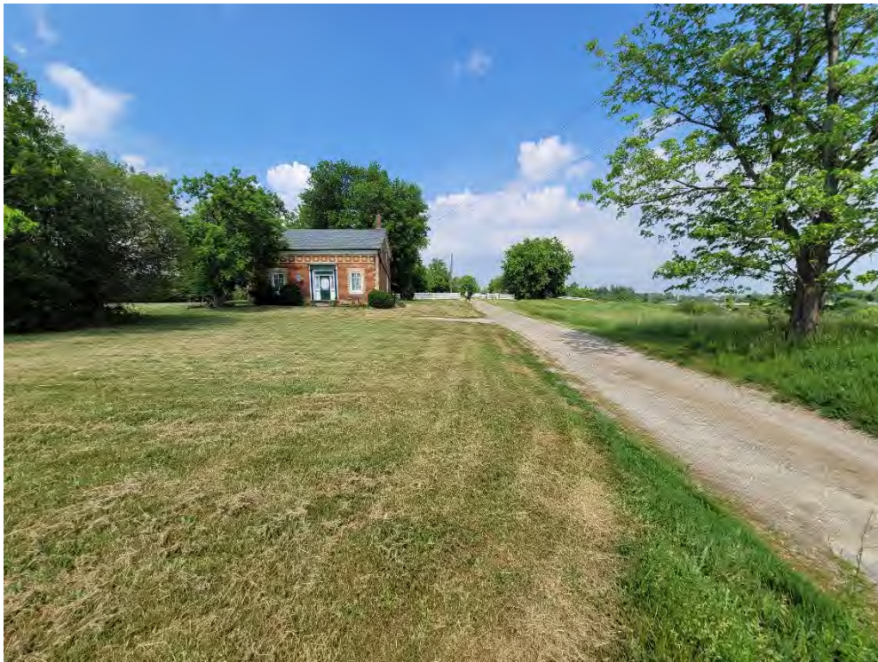
Figure 9: View facing east from Airport Road of the property's driveway, front lawn, and farmhouse
