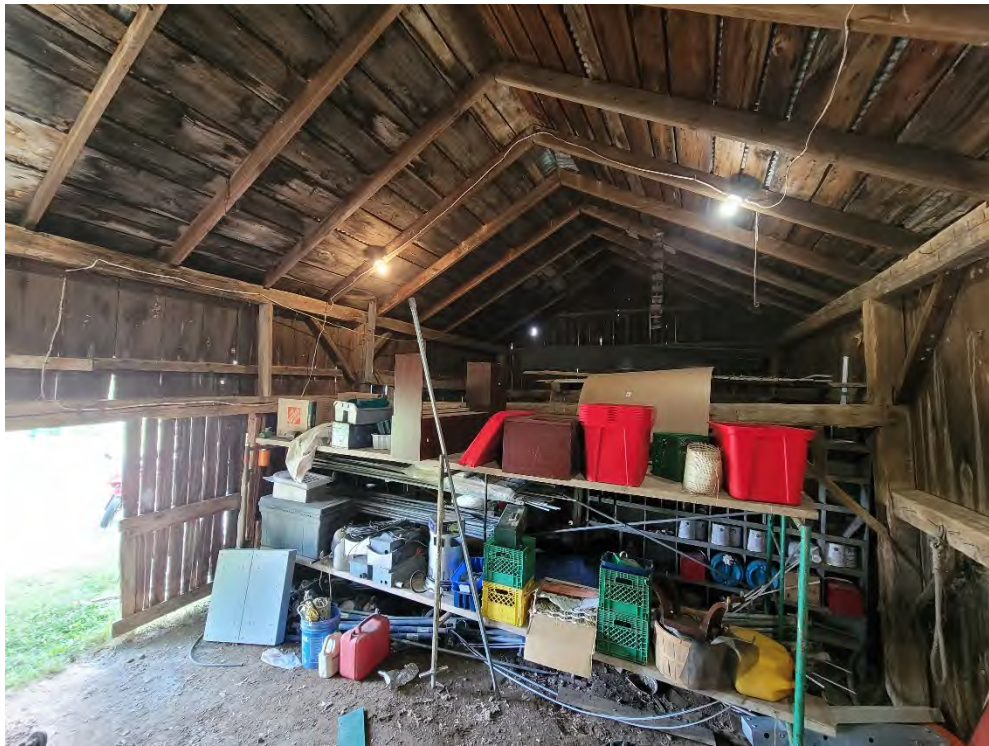
Figure 66: Interior of driveshed, facing west
