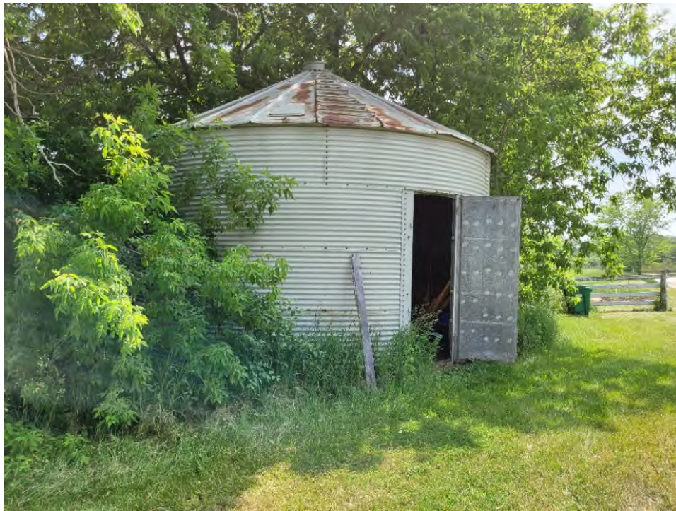
Figure 69: Exterior of metal grain bin, facing southwest
