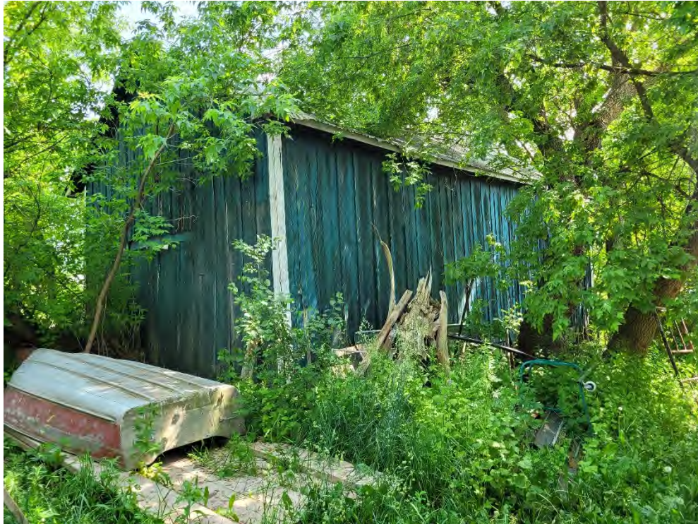
Figure 65: North façade and east wall of the driveshed, facing southwest
