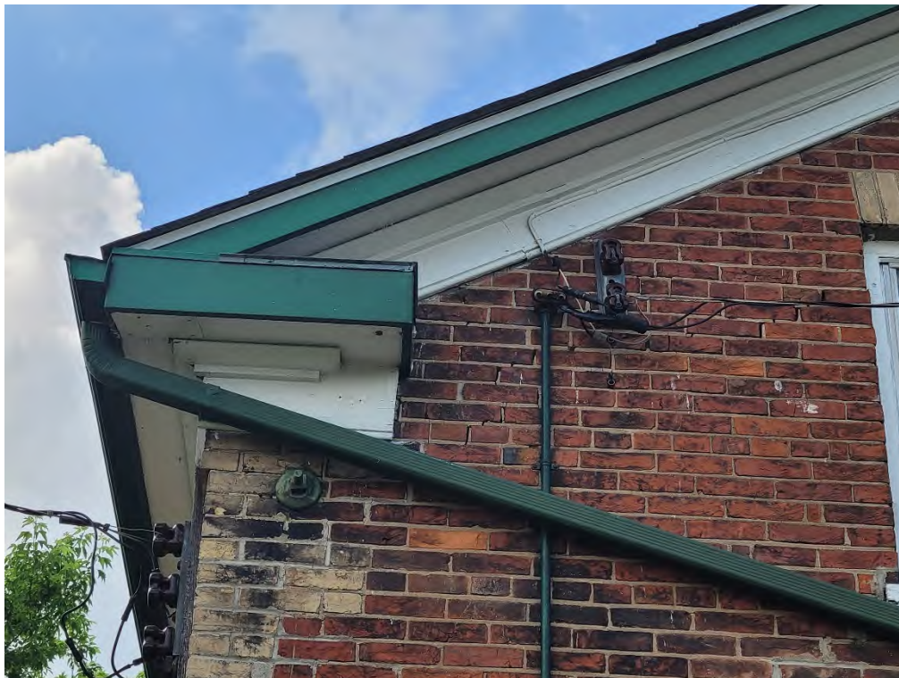
Figure 21: Projecting eaves and verges of the main block with cornice return, moulded frieze and soffit, plain fascia, prefabricated rainwater leader, and tie rod
