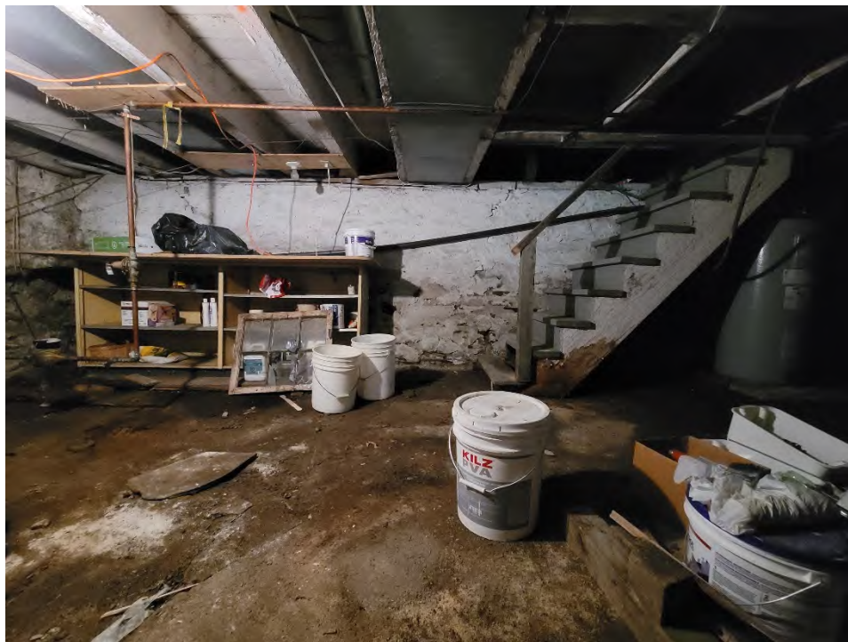
Figure 53: Basement, facing north
