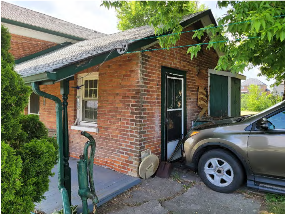
Figure 16: South façade and east end wall of the rear wing
