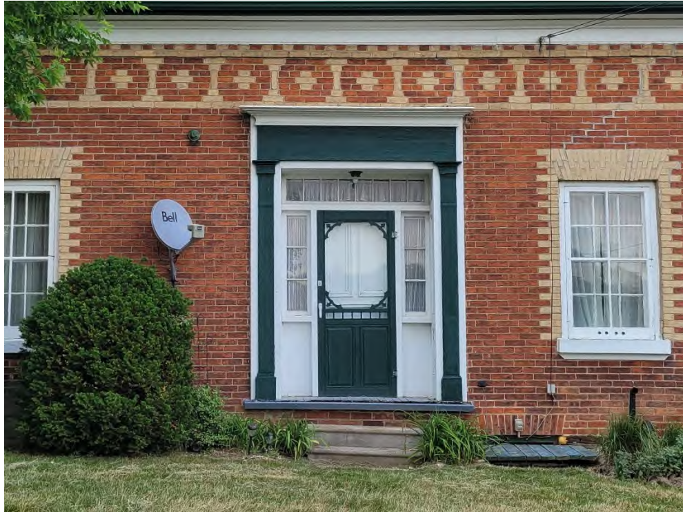
Figure 23: Recessed main entrance with transom, sidelights, pilasters, and entablature
