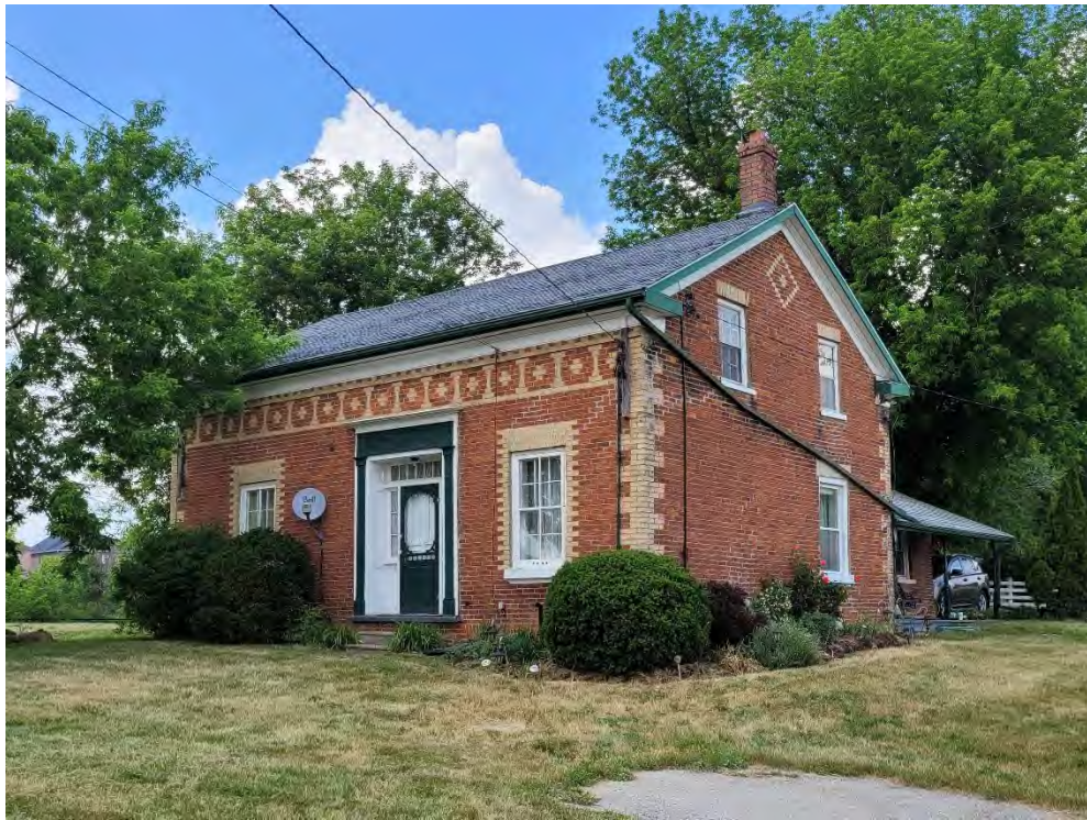
Figure 14: West façade and south end wall of the Sargent Farmhouse
