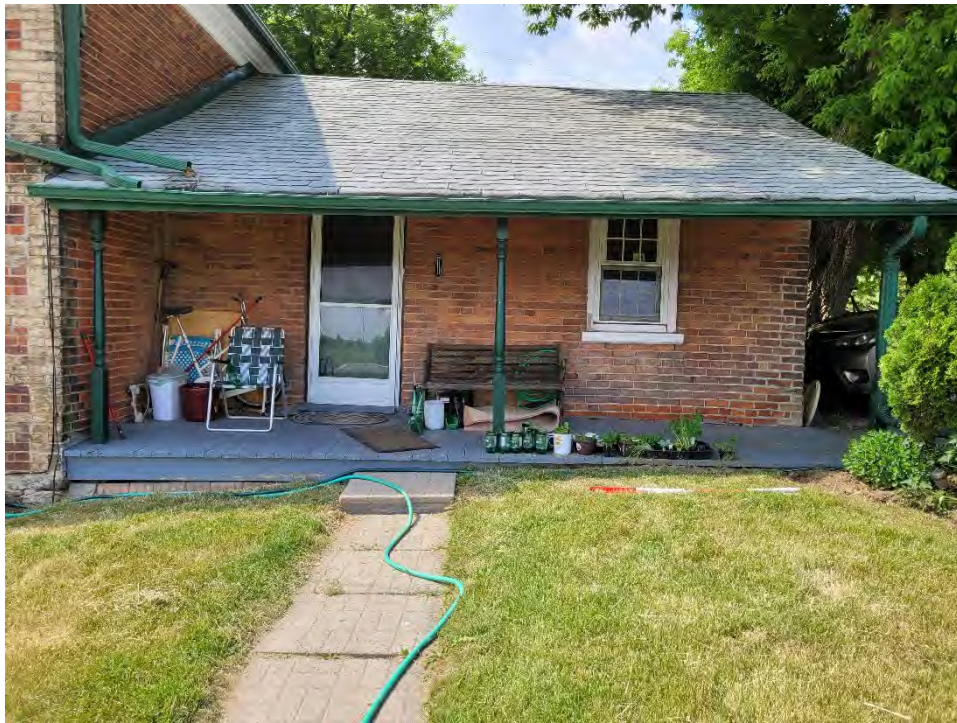
Figure 57: South façade of the rear wing with open verandah
