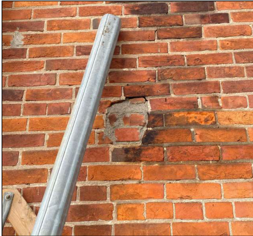
Photograph 10: Repair of past holes
