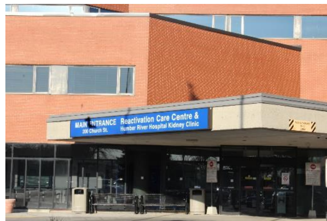
Reactivation Care Unit
